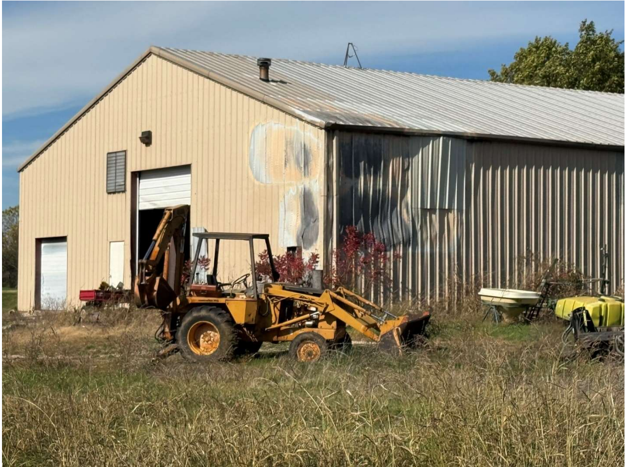
Deteriorated structure on Parcel 2.
