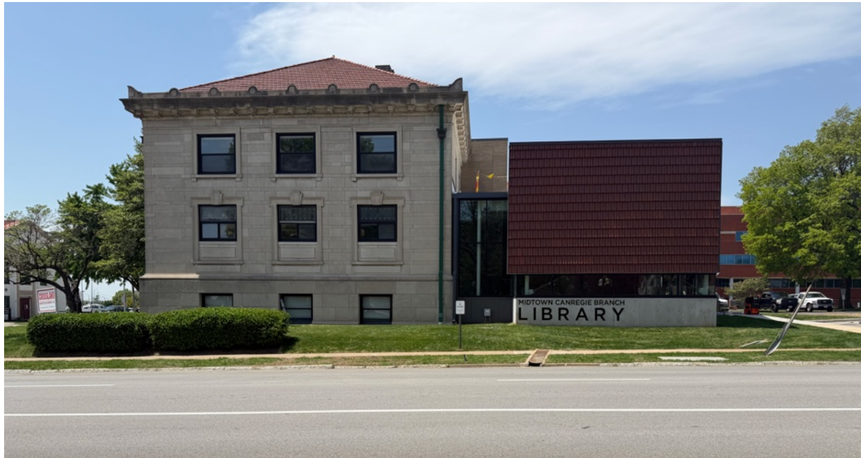
IMAGE 6: Construction photo of the new addition with proposed sign on the east elevation of the addition.
