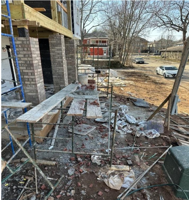
G49. The construction site with scattered debris, unfinished bricks, and scaffolding, indicating an incomplete work area.
