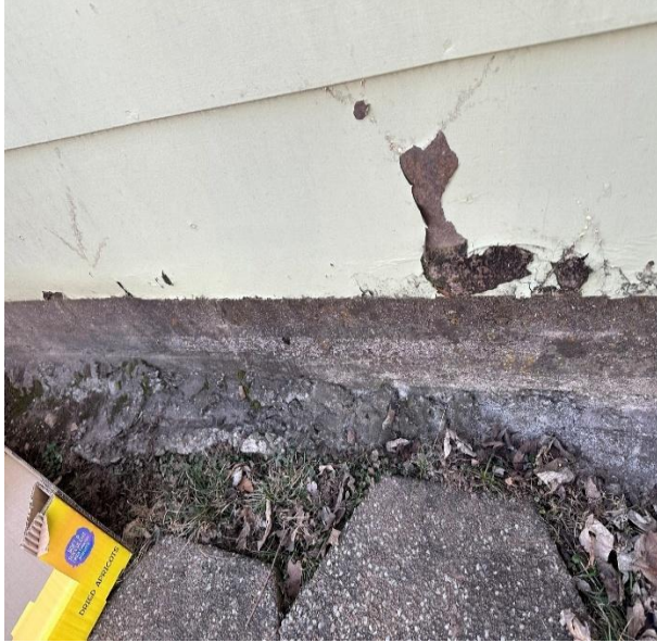
G36. The siding in this image is severely cracked and deteriorating, exposing the underlying structure to potential water intrusion and further structural issues.
