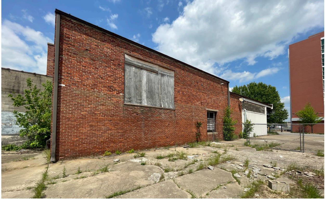
42. South Elevation of the building .
