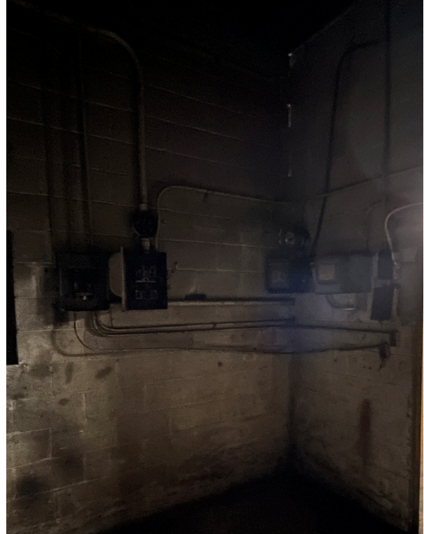
24. Wiring serving the existing electrical panels have been removed throughout the building.
