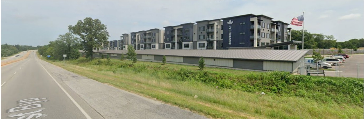
View from West Bypass looking northeast
