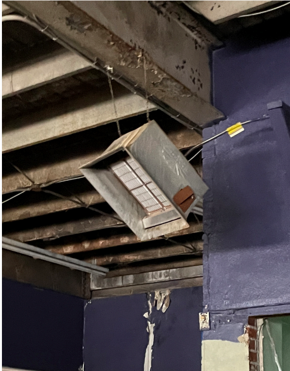
21. Gas service to the building has been shut off and the meter removed.
