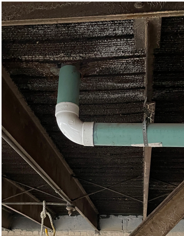
17. Roof drain penetration through existing roof slab.
