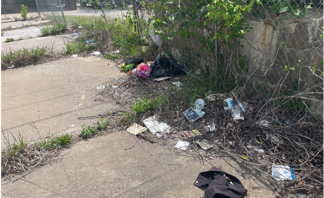
5. Trash and human waste have amassed in the exterior spaces around the building.
