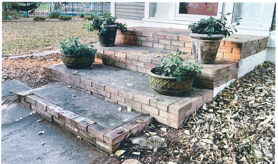
Current Front Porch/Steps
