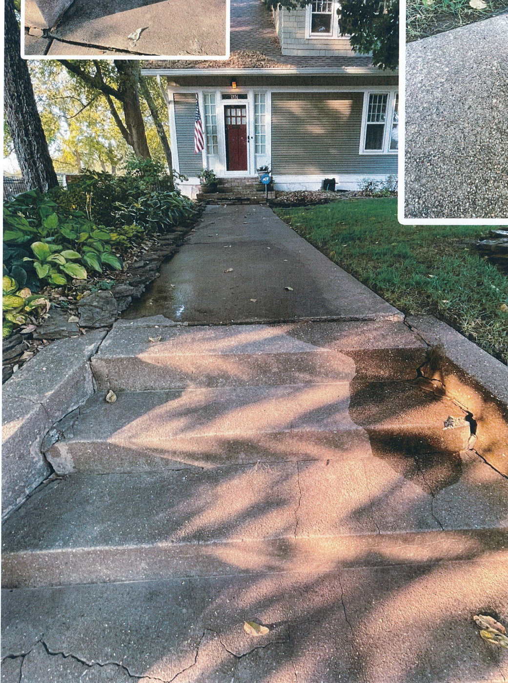
Current Entry Sidewalk & Steps
