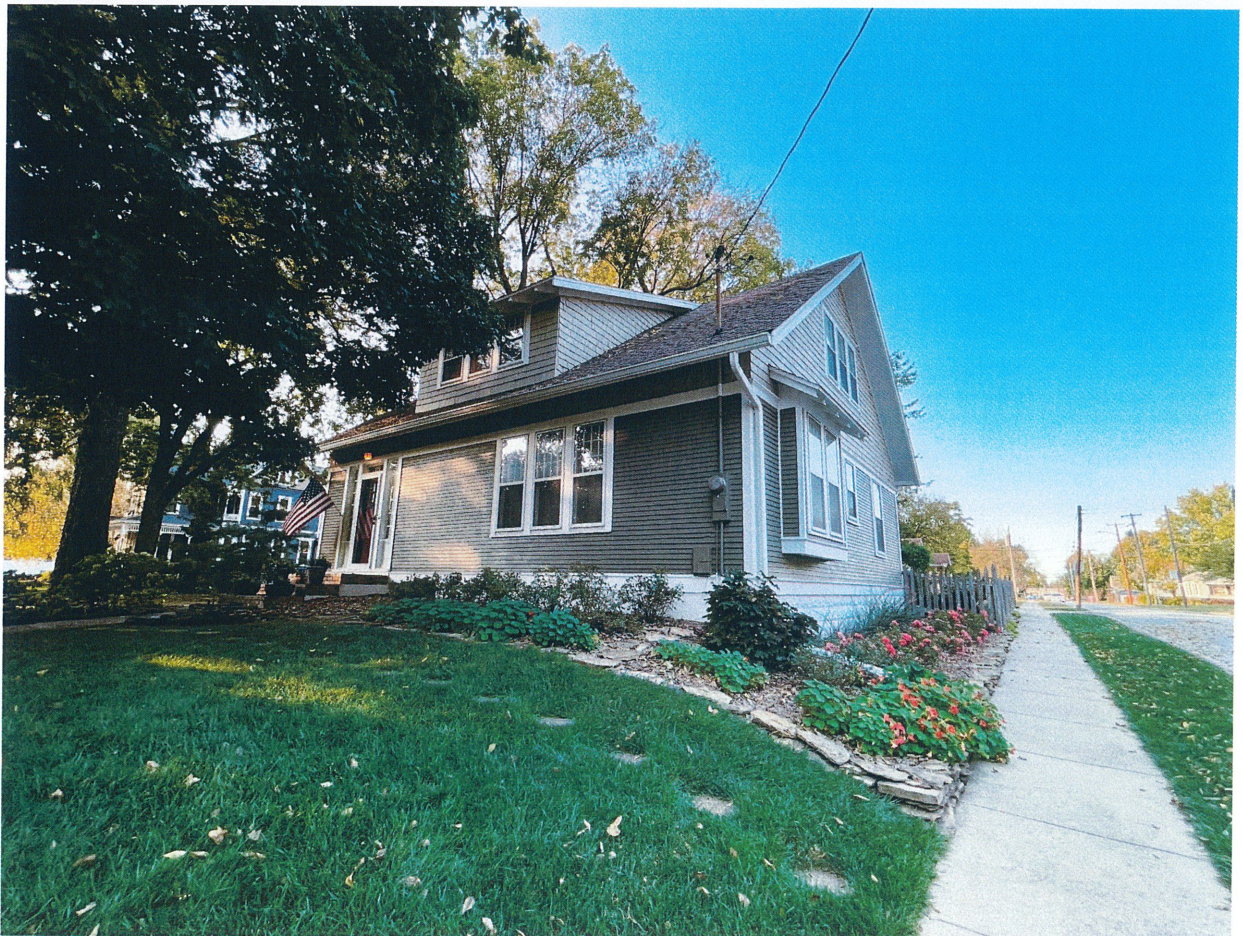
Views from the Southeast
