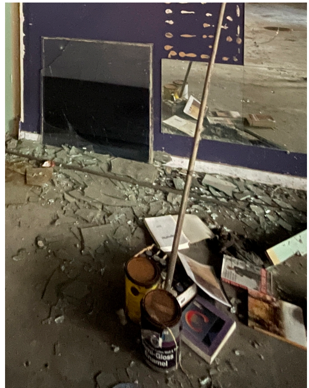
4. Broken Glass and debris.
