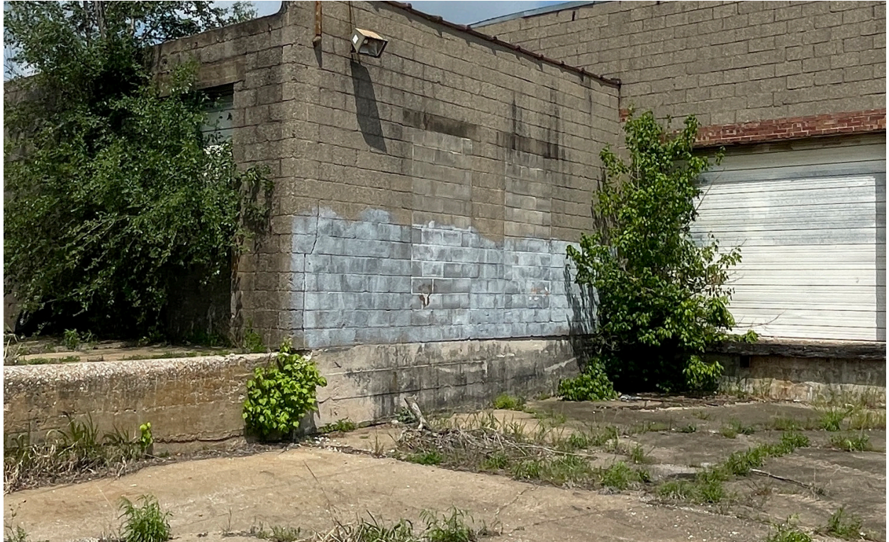
37. Area of existing building where graffiti was covered up.
