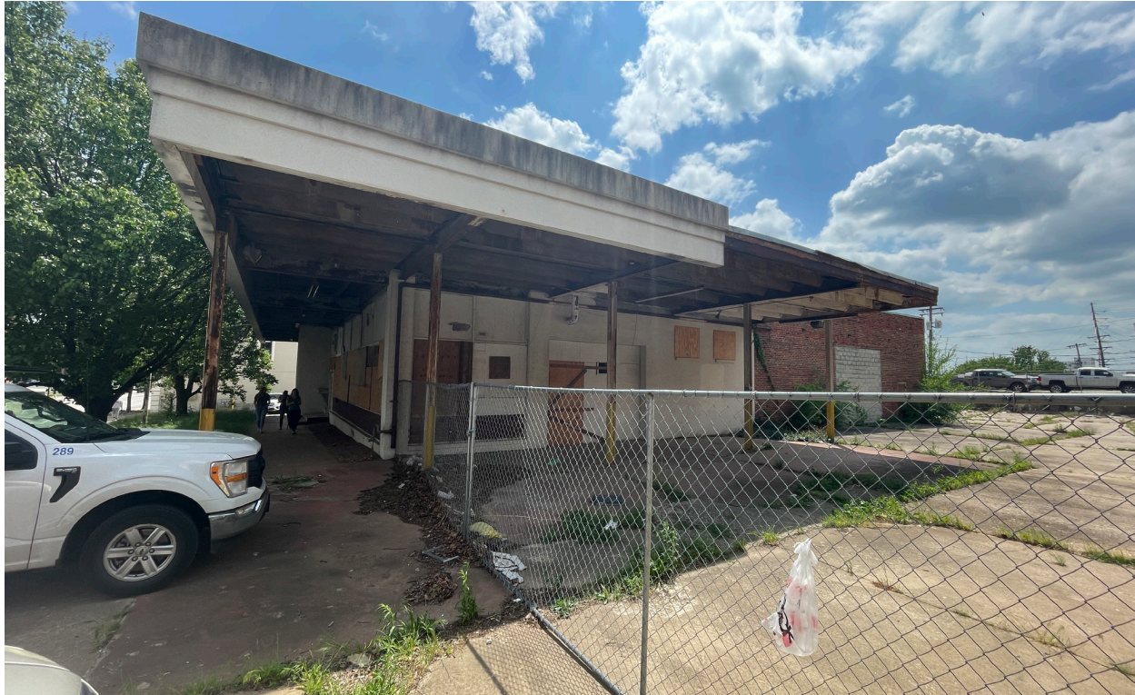
39. North elevation of the building.
