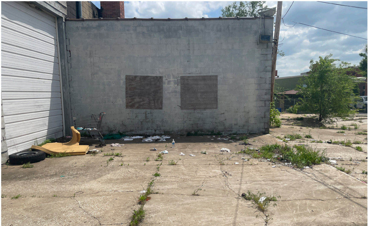
6. Southwest corner of the building where homeless individuals have been sleeping.
