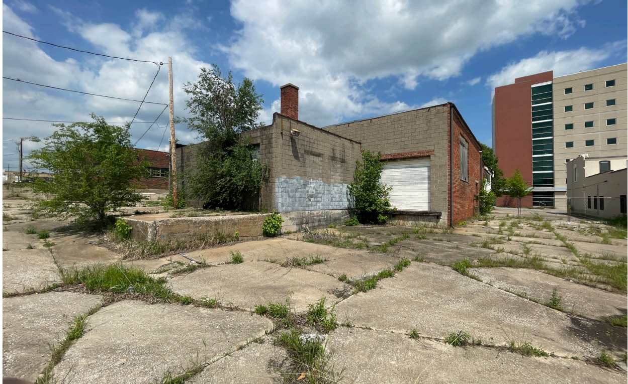
41. Portion of West elevation.
