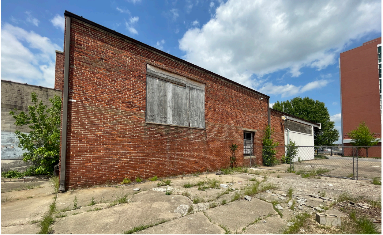
42. South Elevation of the building .
