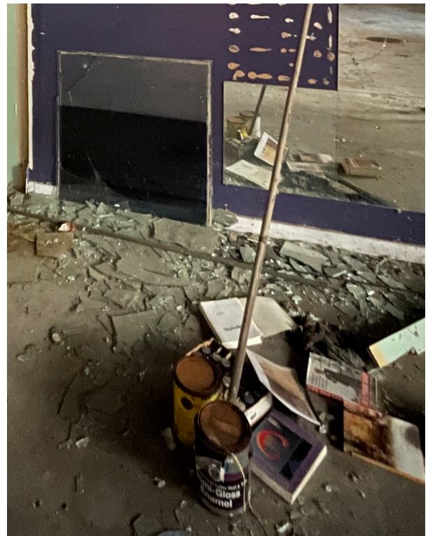
4. Broken Glass and debris.
