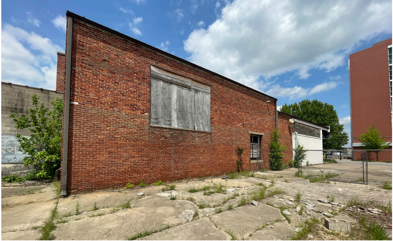
42. South Elevation of the building .
