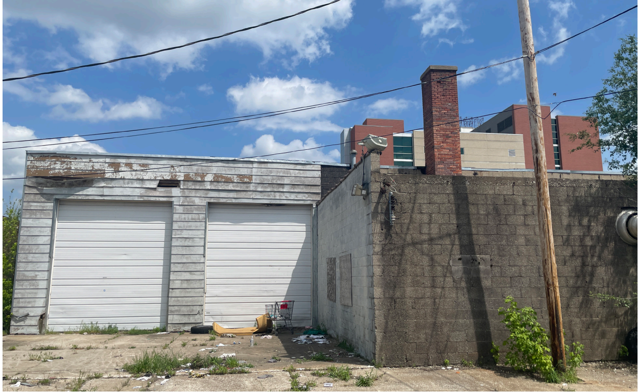
40. Portion of West elevation.
