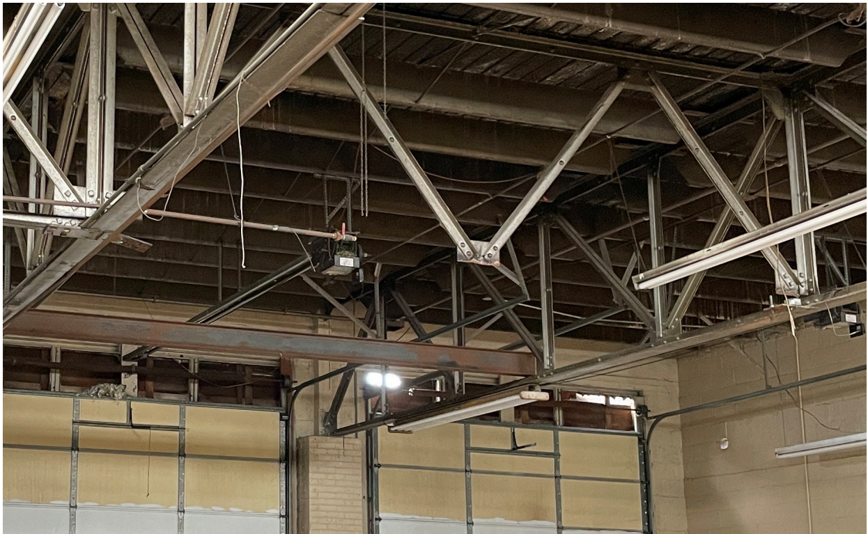
15. Portion of the existing lateral support for the garage area has been removed.
