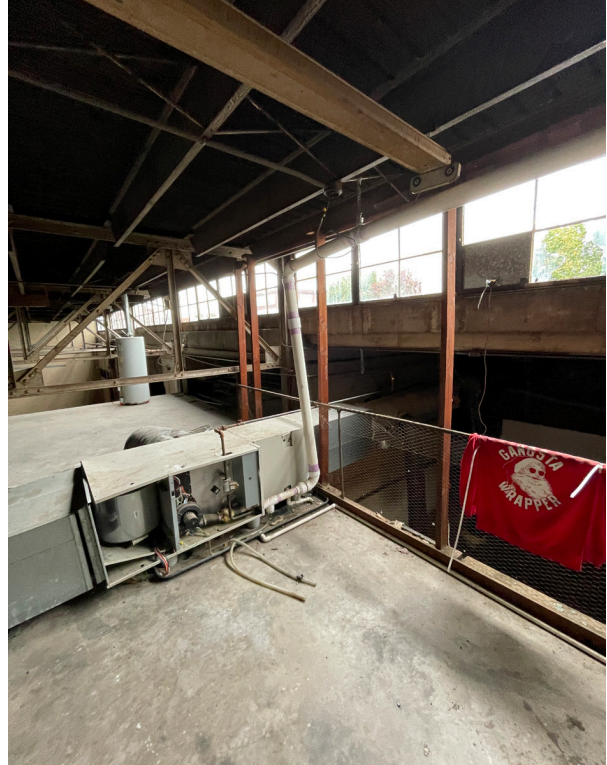
20. Electrical parts from the existing air handler unit have been removed.
