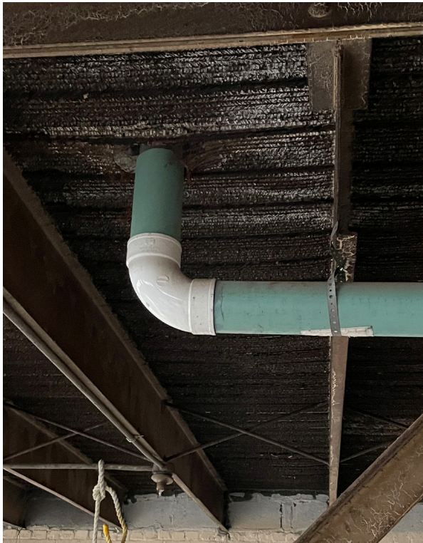
17. Roof drain penetration through existing roof slab.
