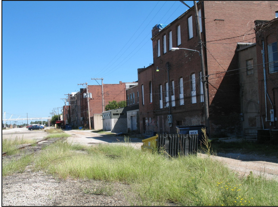
Property on north side of Commercial Street buildings
