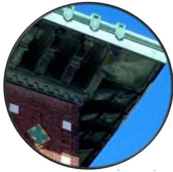
Copper Cornice Terracotta
