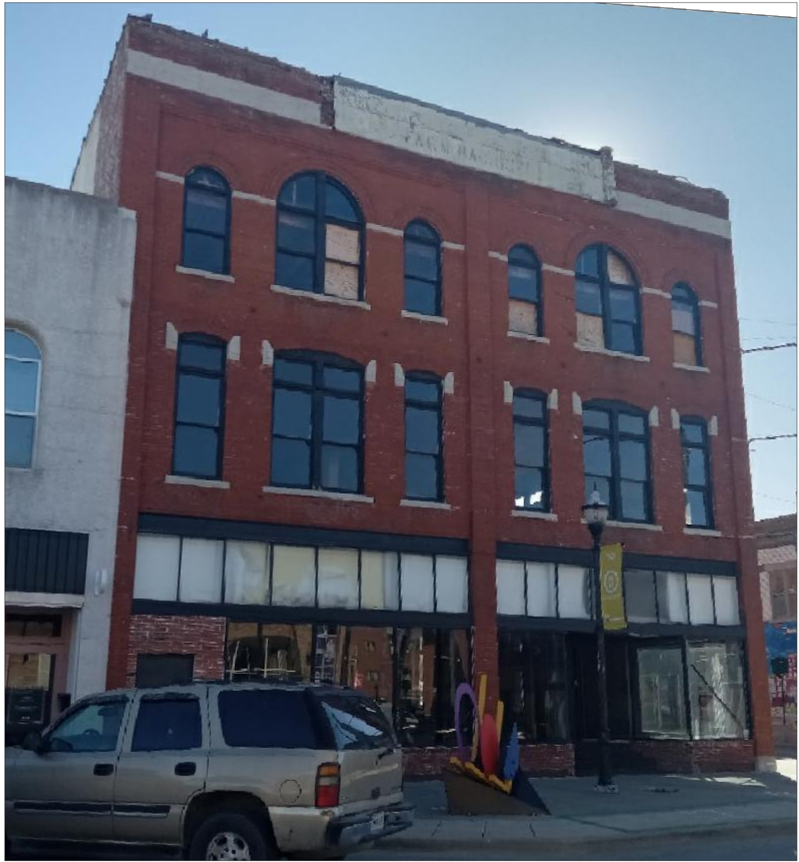
OVERALL VIEW: North Elevation No Scale
