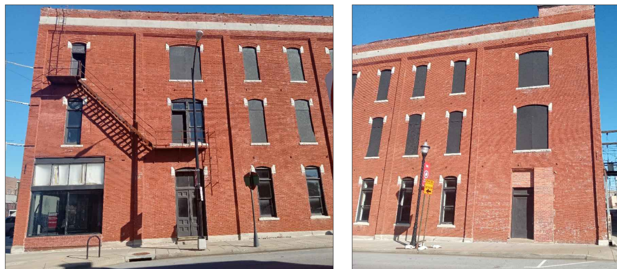
OVERALL VIEW: West Elevation No Scale
