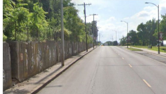
College St. looking West towards Kansas Expressway and future Jordan Creek Greenway connection- Sidewalk on south side of street is currently inaccessible due to utility poles centered within path.
