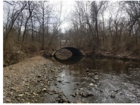
Abandoned Bridge culvert over Wilsons Creek- Hillcrest Ave – Future Pedestrian Bridge
