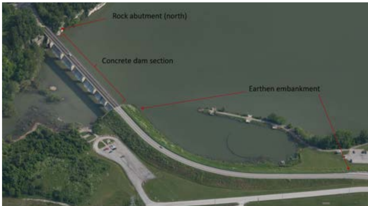
Figure 11: Lake Springfield Dam
