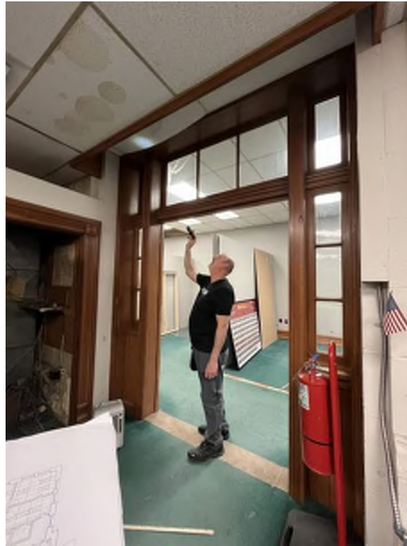
View looking at windows for Offices 118/119 see floor plan
