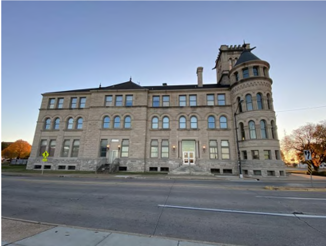
View of West Elevation
