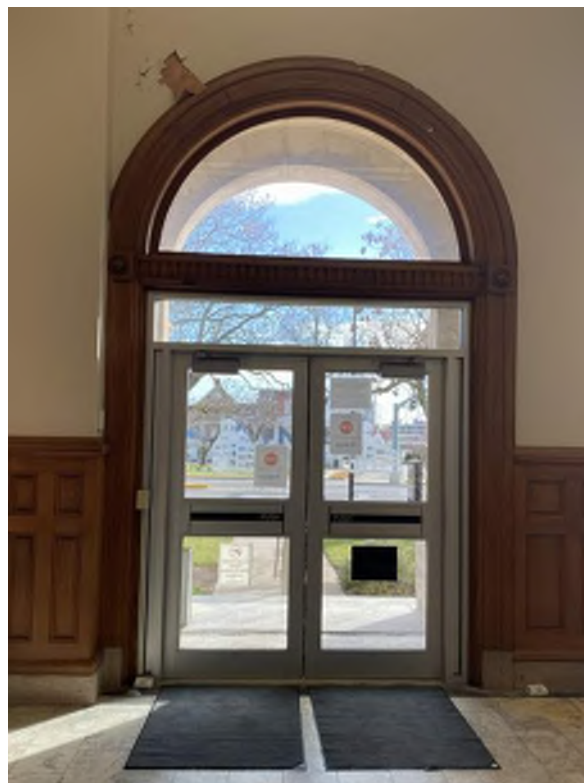
View looking out existing South Entry
