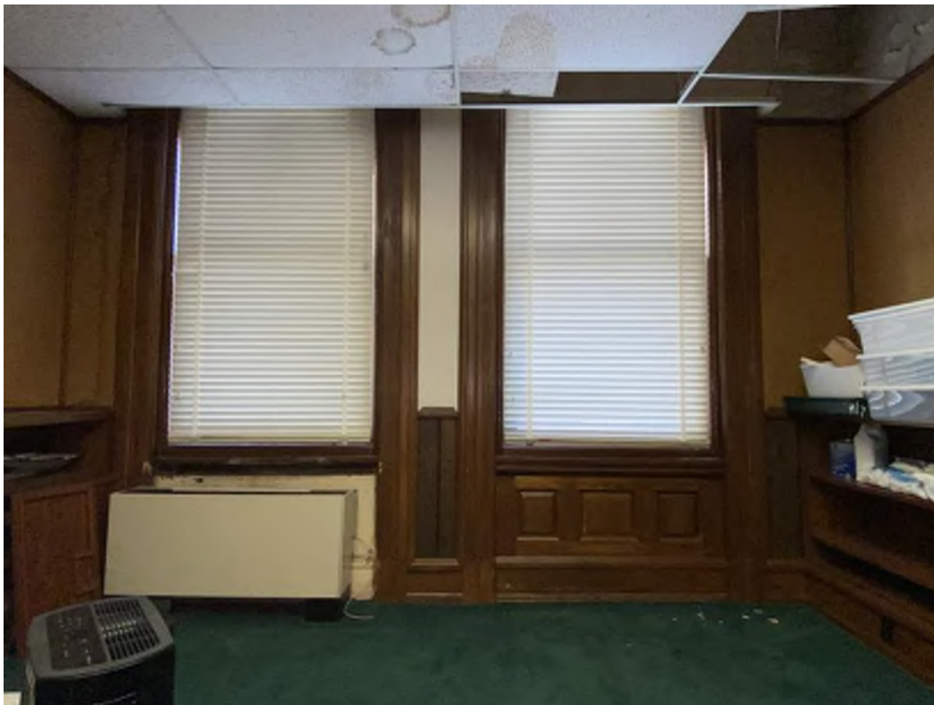
Typical wood wainscot/window trim in 2nd/3rd floor offices. Remove FCU unit, repair and refinish wall treatment/base.
