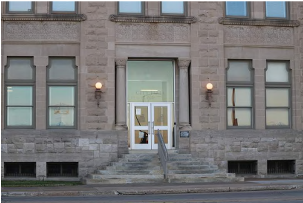
Existing West Entry, replace door/frame, repair stairs & railings
