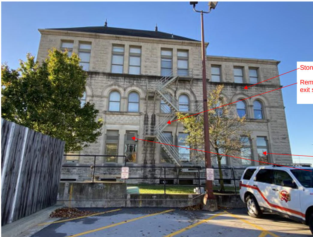
View of North Elevation
