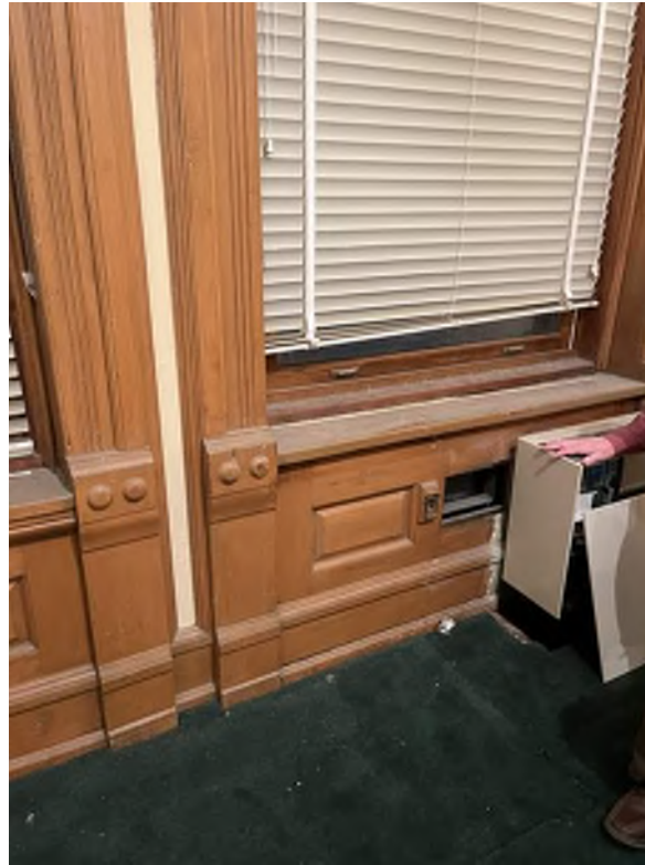
Typical wood wainscot/window trim in 2nd/3rd floor offices. Remove FCU unit, repair and refinish wall treatment/base.
