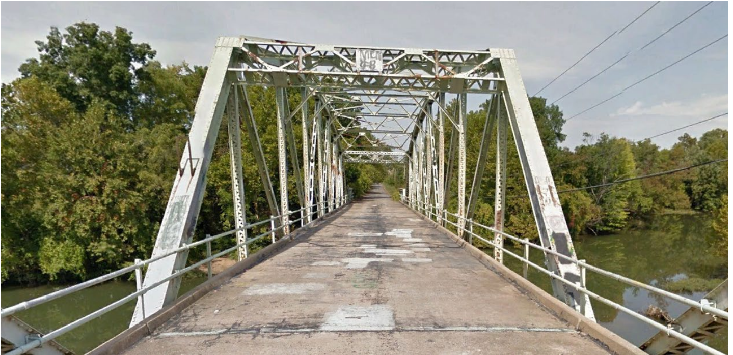
South End of Bridge (looking north)
