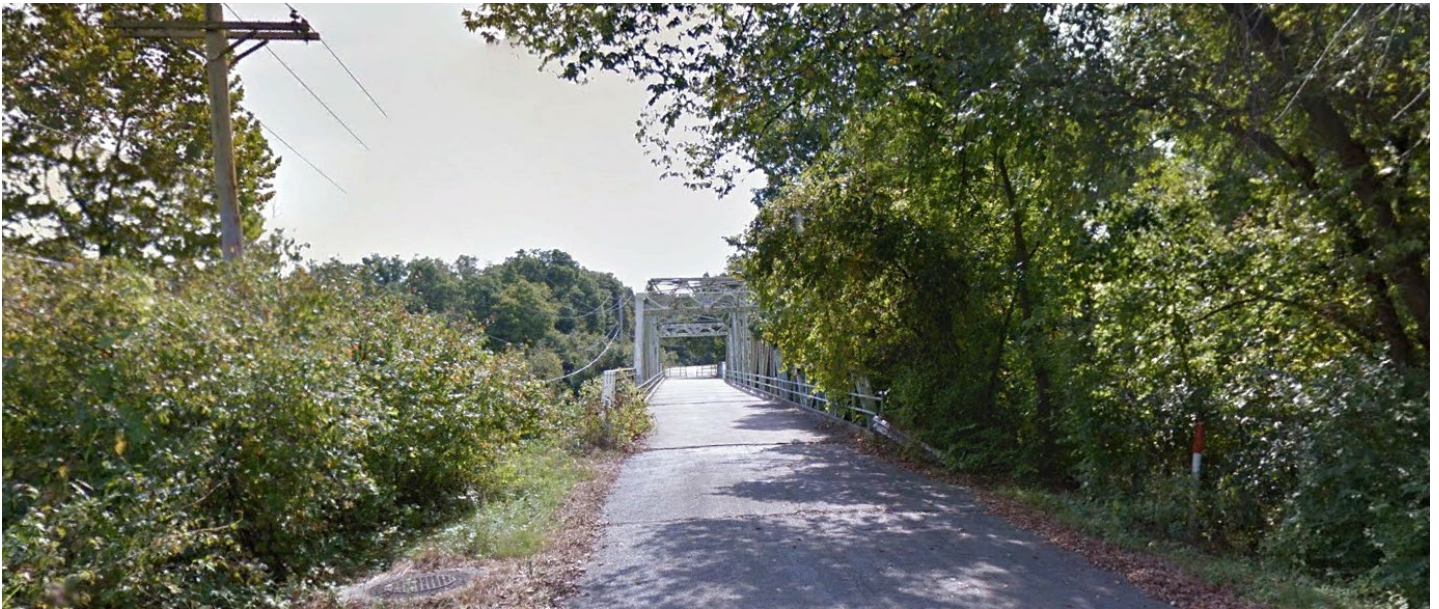
North End of Bridge (looking south)
