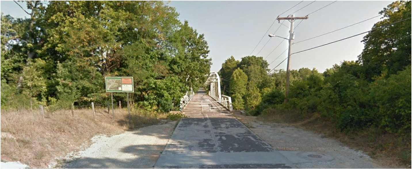
South End of Bridge (looking north)
