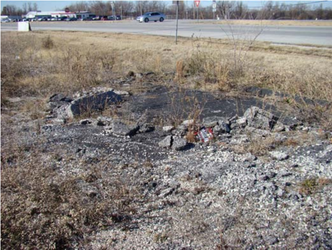
Rubble and debris remaining from past demolition activities and, potentially also, dumping.
