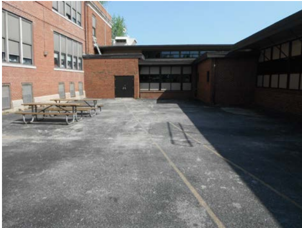
Figure 25: Robberson Elementary Courtyard
