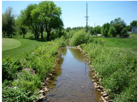
Figure 24: Ward Branch after stream bank stabilization
