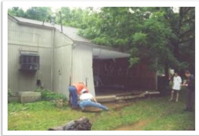
Figure 5. 2000 Flood in Shadowood Subdivision. Note missing wall on damaged home.
