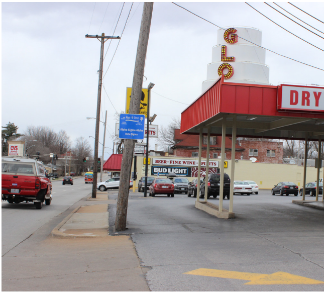
NATIONAL AVENUE AT CHERRY STREET
