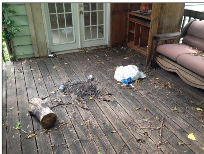
A27.) Beer cans are collected near an abandoned couch on the back deck of a vacant structure.
