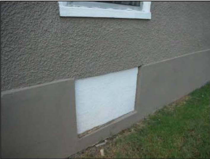
Windows boarded up
