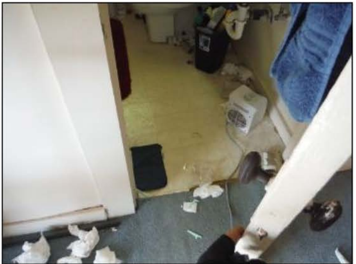
General wear and tear
