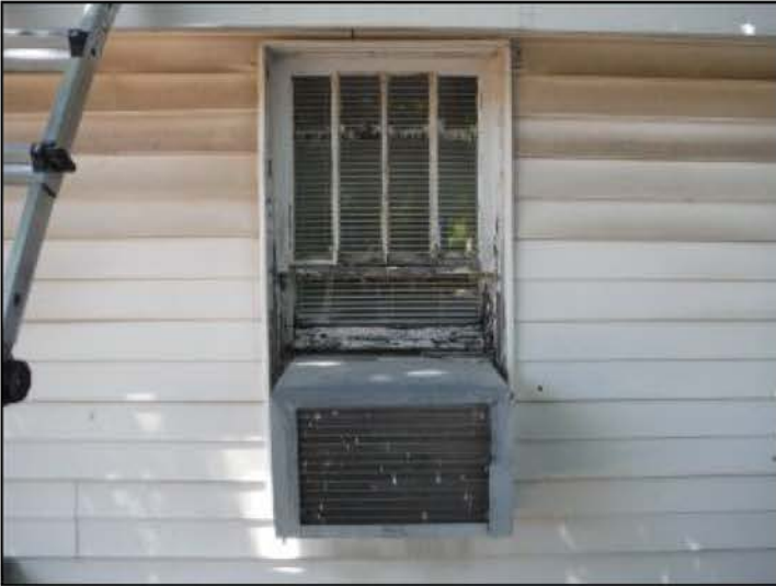
Older package air conditioner has limited life
