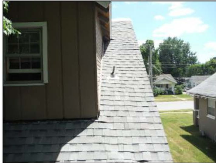
Limited inspection, not walked
