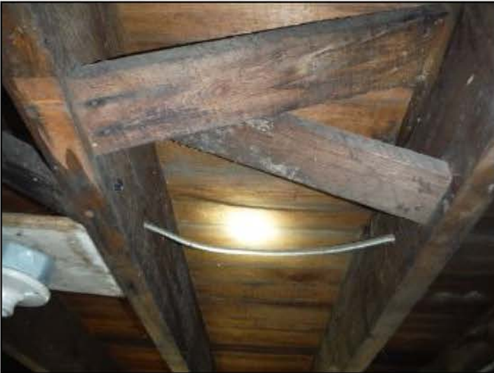
Old school X bridging is sign of good construction
