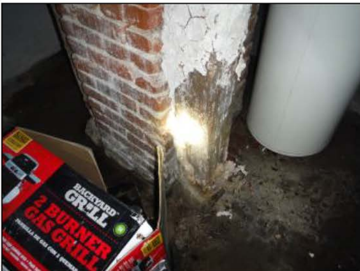
Rotted posts, refer to termite inspection report
