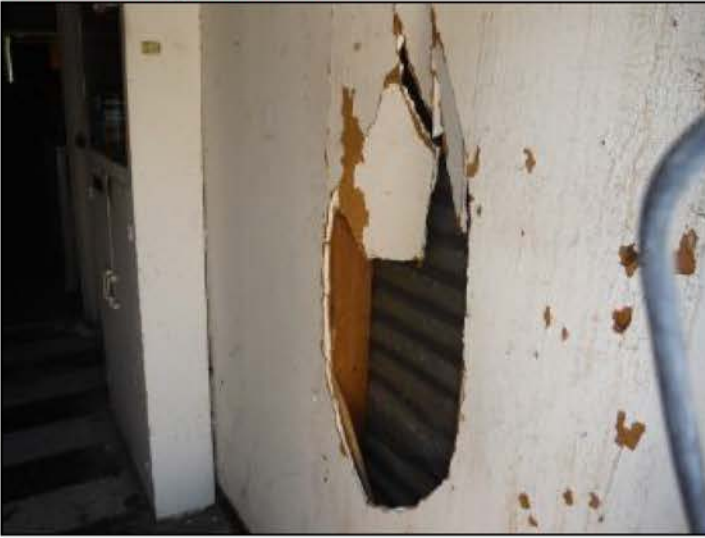
Damaged drywall
