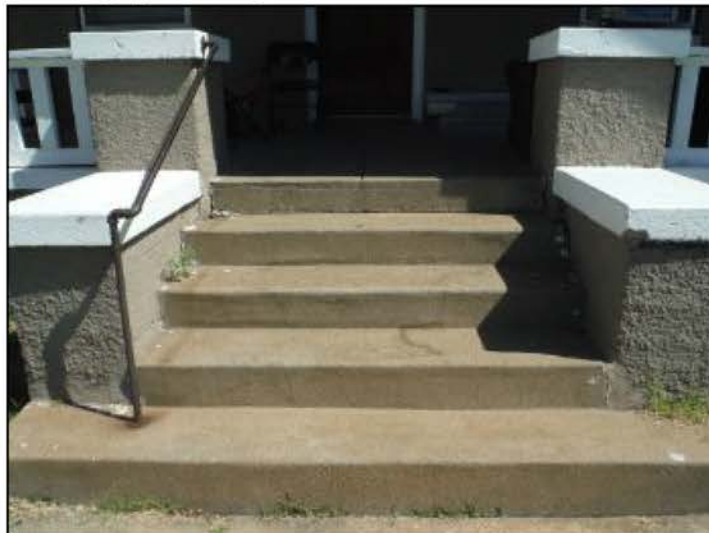
Serviceable concrete has a steel pipe railing one side
