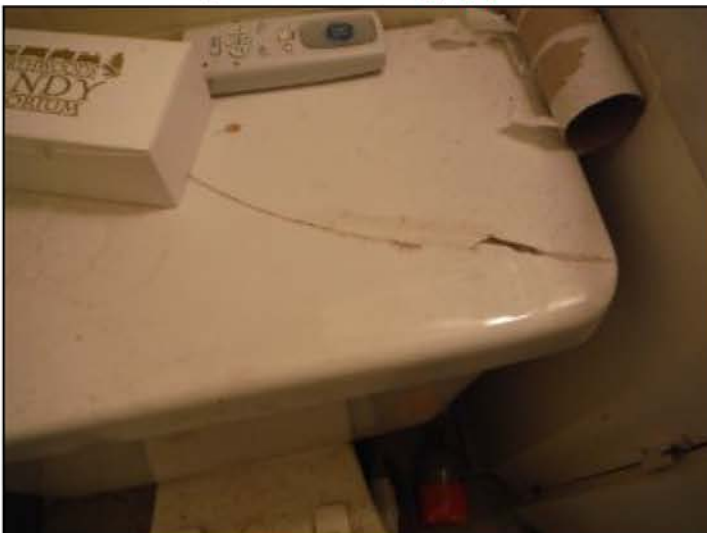
Damaged tank lid
