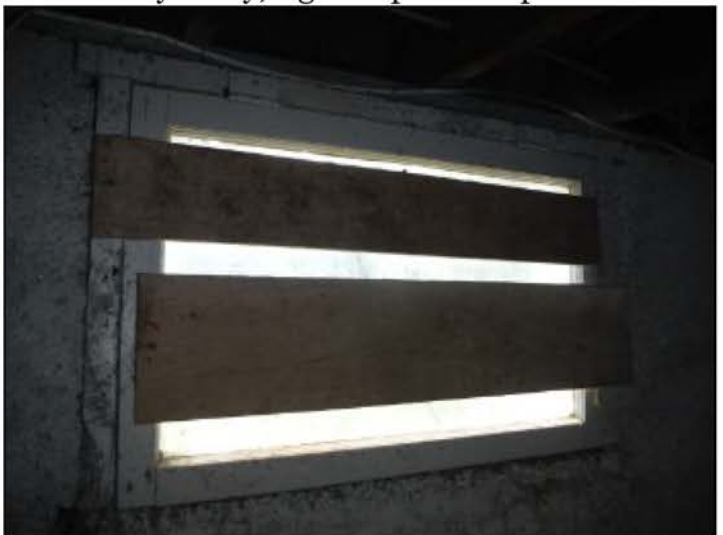
Windows boarded up
