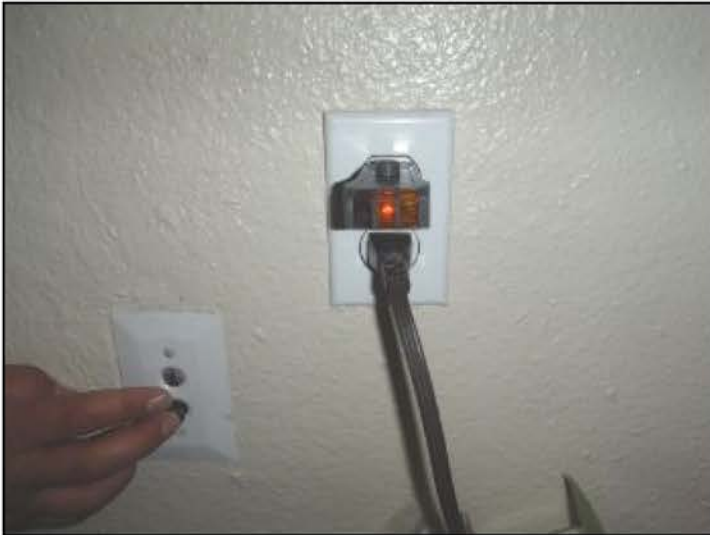
Ungrounded/miswired (reverse polarity) outlet/s found, suggest all be checked and corrected
