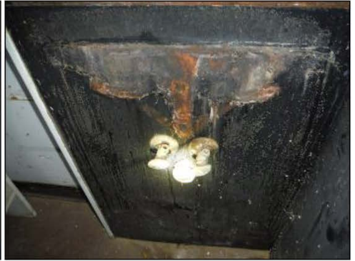
Some storage is hazardous (broken glass in photo)
