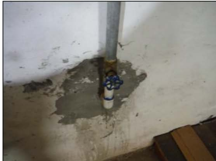
Main valve appears serviceable
