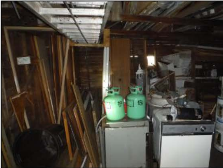
Storage limits inspection, some is hazardous
