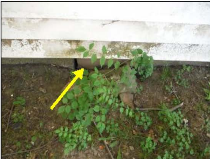
View port --- otherwise inaccessible below floor
