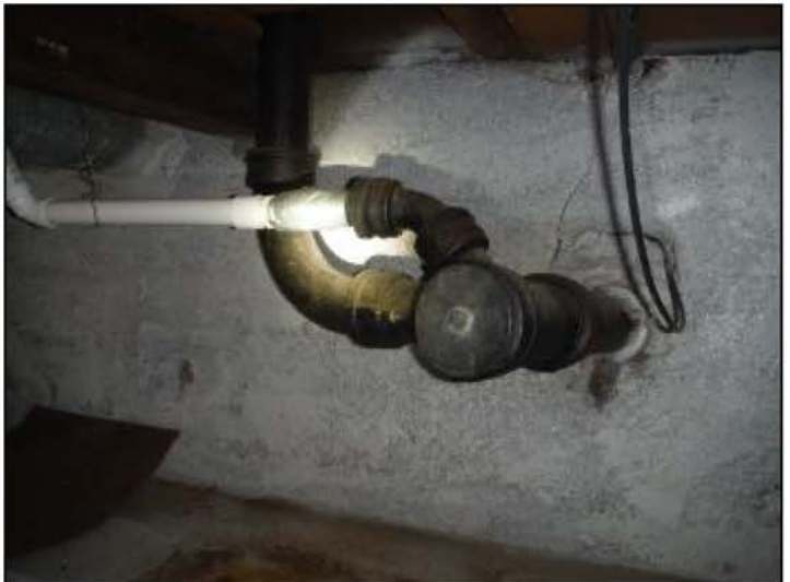
Most is older cast iron type
