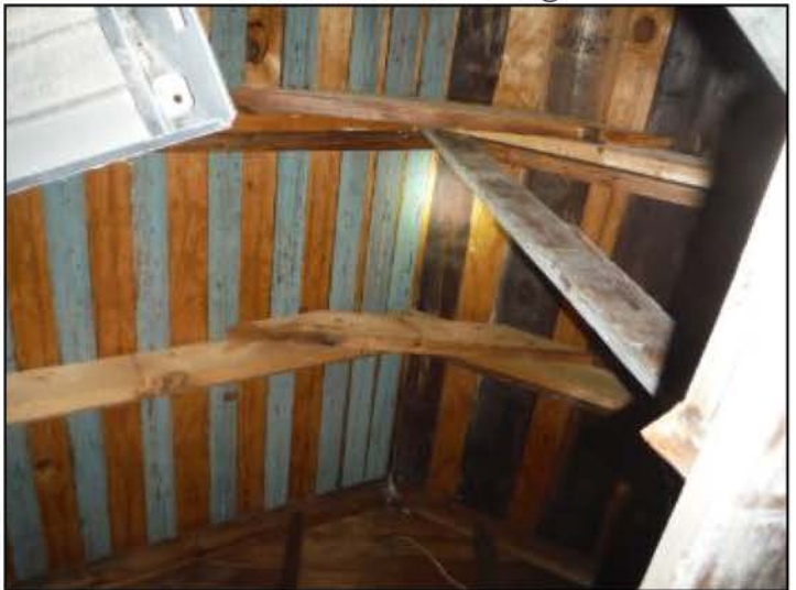
Has newer bracing and repairs
