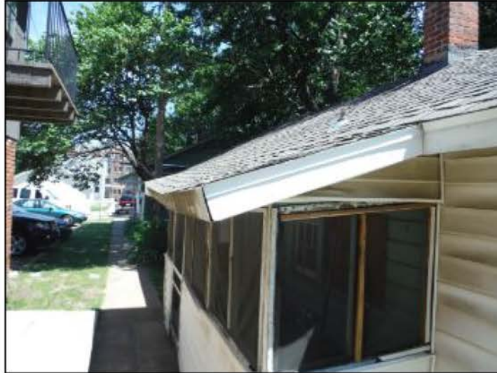
Same roofing as main roof
