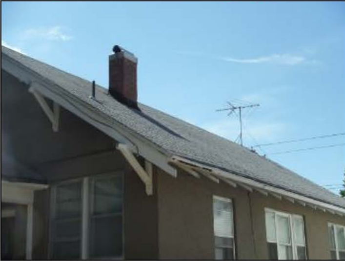
Two layers is limit since February 1995, this house has three
