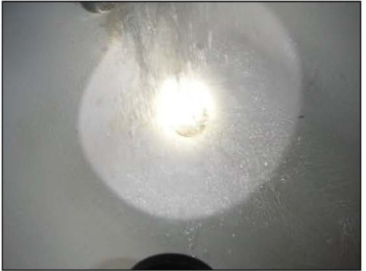
And stopper needs adjusting
