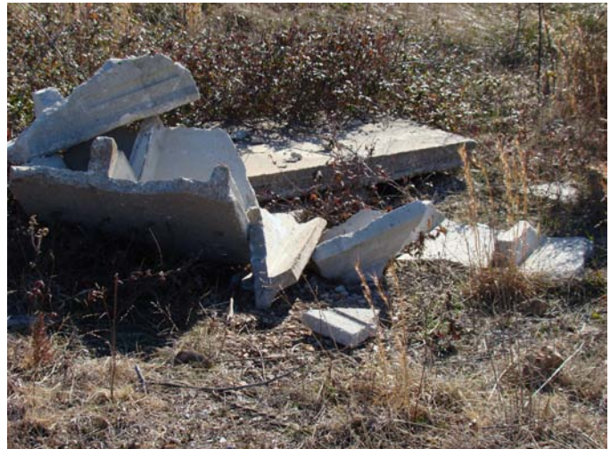
Evidence of illegal dumping occurring in the Redevelopment Area.
