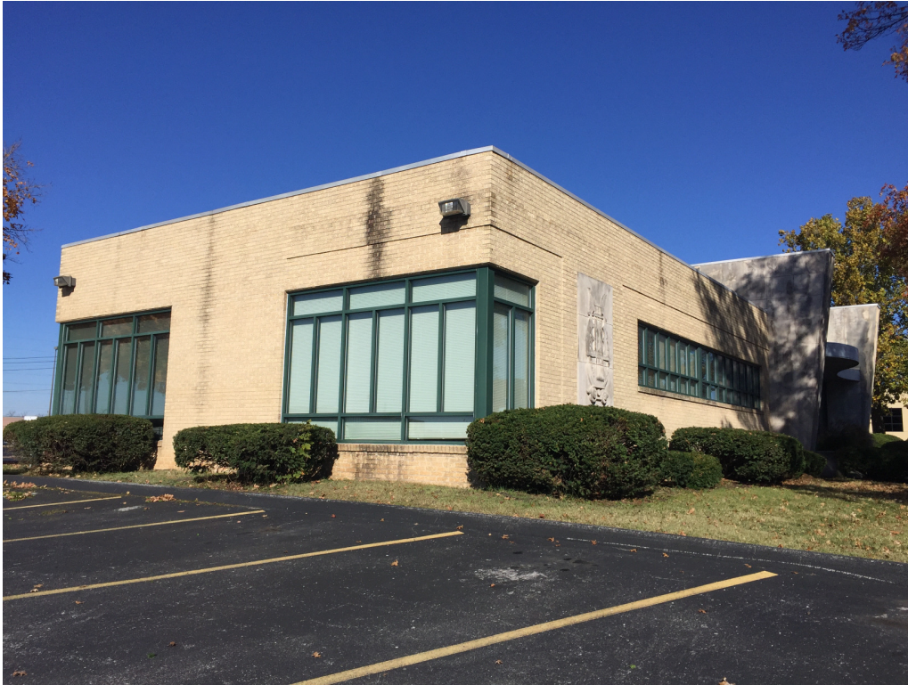
Figure 7 – Wrapped windows at south façade. Photo by author.
