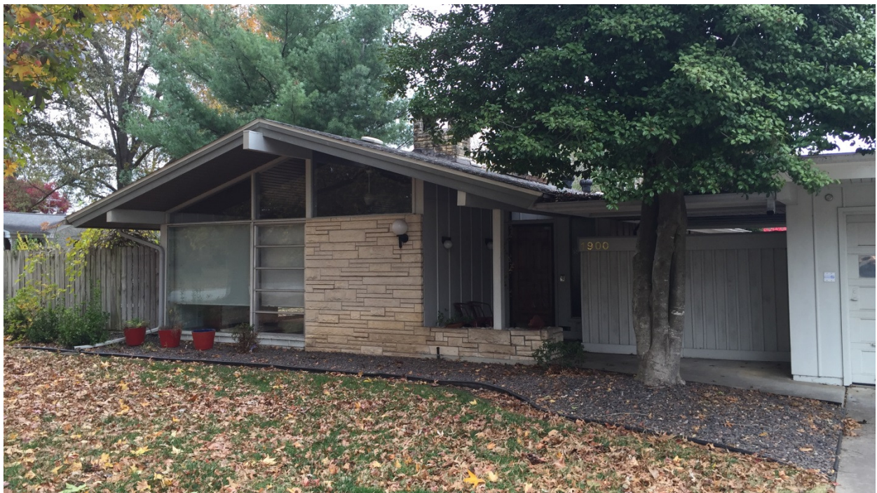
Figure 6 -West façade. Photo by author.
