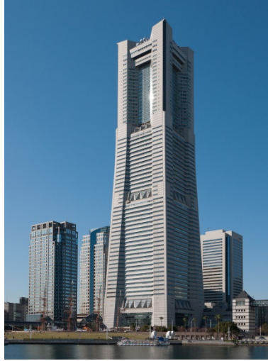
Yokohama Landmark Tower Japan – 1993
