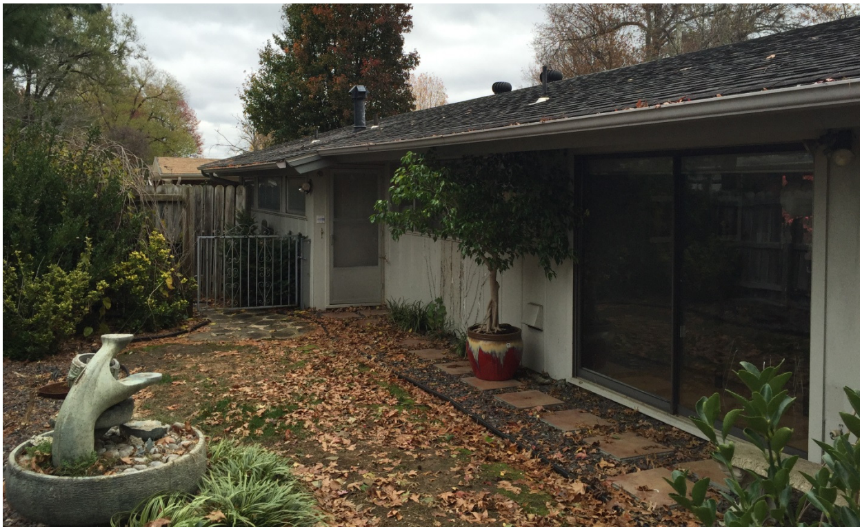
Figure 8 – North façade. Photo by author.
