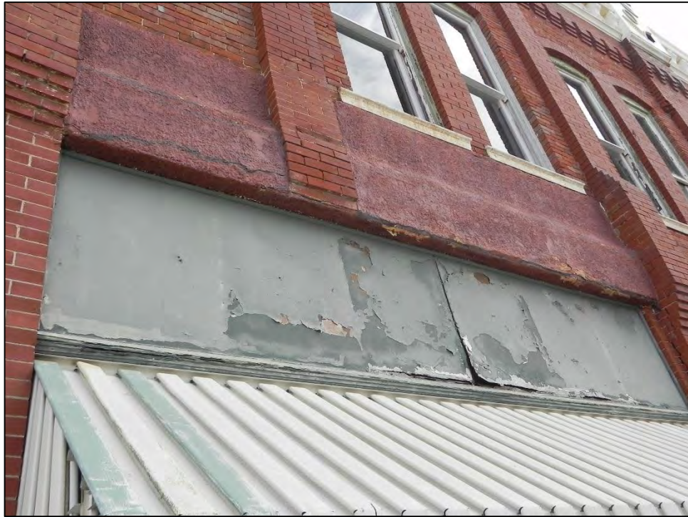
Photo 3: Detail of plastered area above transoms of north storefront at side west elevation, segmented by brick pilasters. March 14, 2014.
