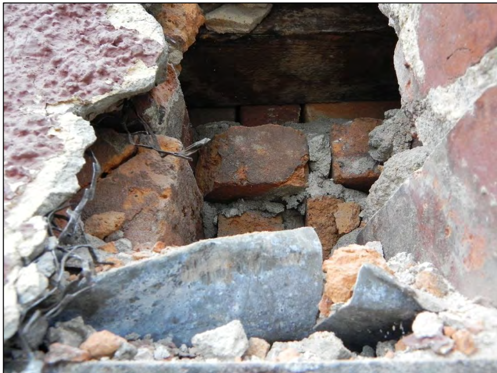
Photo 6: Detail of remnant of original metal cornice attached to steel support beam above transom area of north storefront at primary north elevation. Exposed following exploratory demolition.
