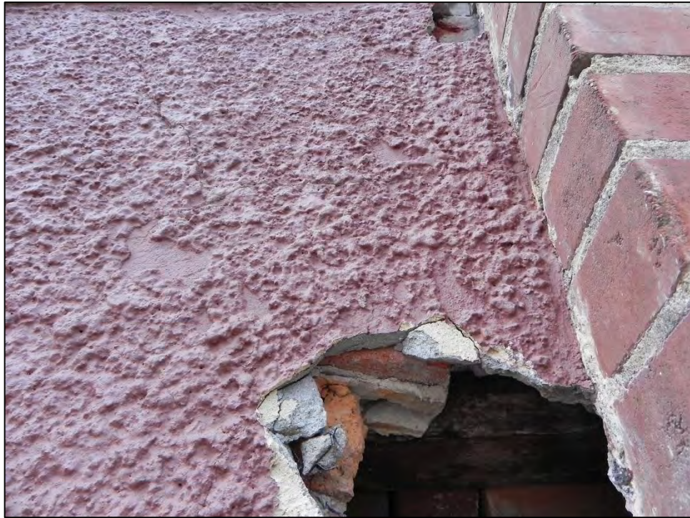
Photo 7: Detail of wood support beam above transom area of north storefront at primary north elevation. Exposed following exploratory demolition.
