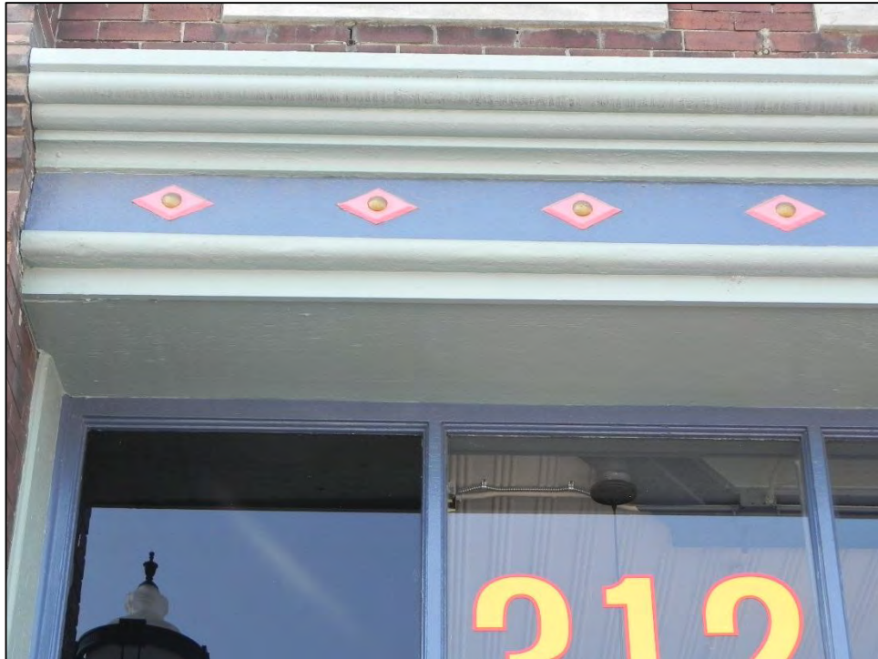
Photo 9: 312 East Commercial Street. Detail of original metal cornice above transom area of storefront at primary north elevation.
