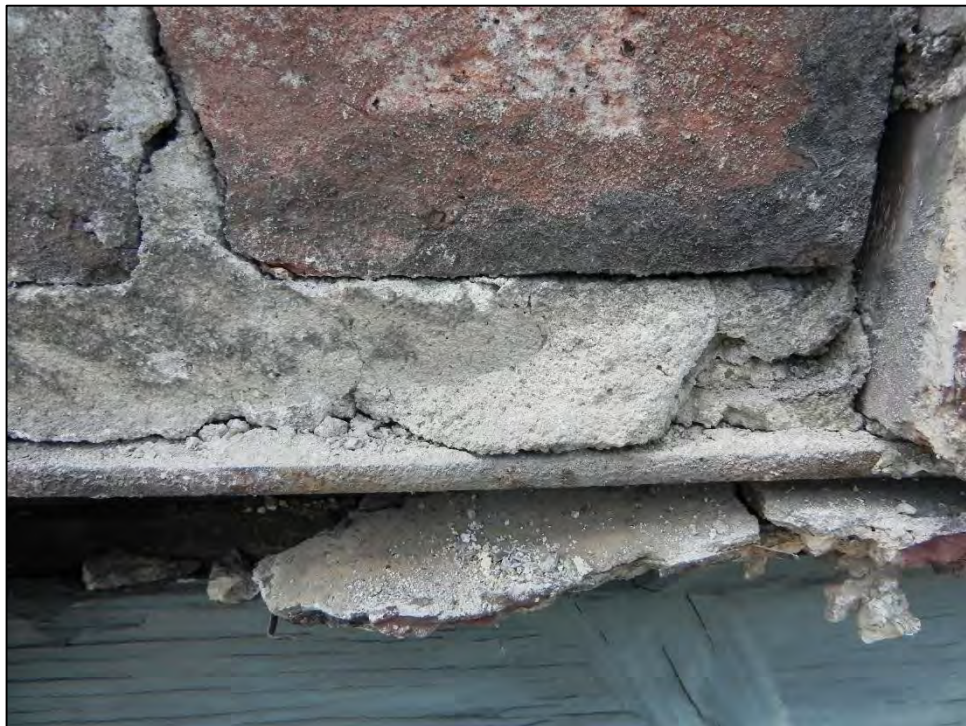
Photo 4: Detail of steel sill plate above transom area of north storefront at primary north elevation. Exposed, with brick above, following exploratory demolition.
