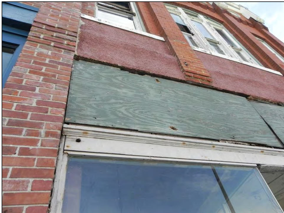
Photo 2: Detail of plastered area above transoms of north storefront at primary north elevation, segmented by brick pilasters. March 14, 2014.
