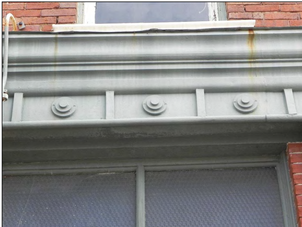
Photo 8: Detail of original metal cornice above transom area of south storefront at side west elevation.
