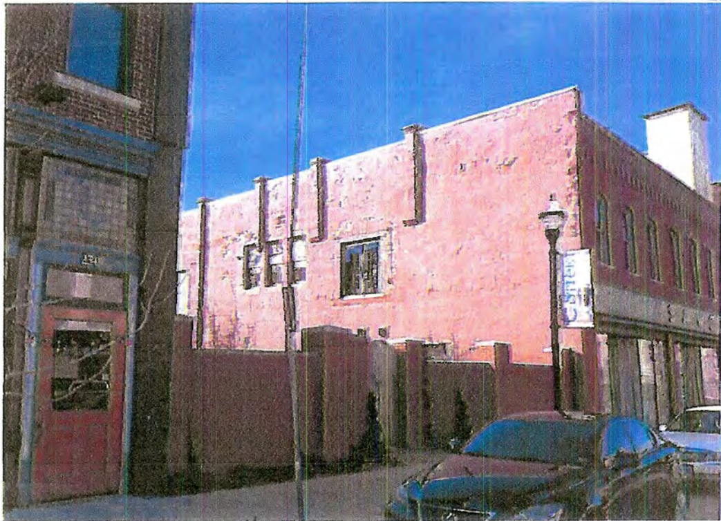
PHOTO #1: COMMERCIAL STREET LOOKING WEST AT EXISTING SAVOY BUILDING.
