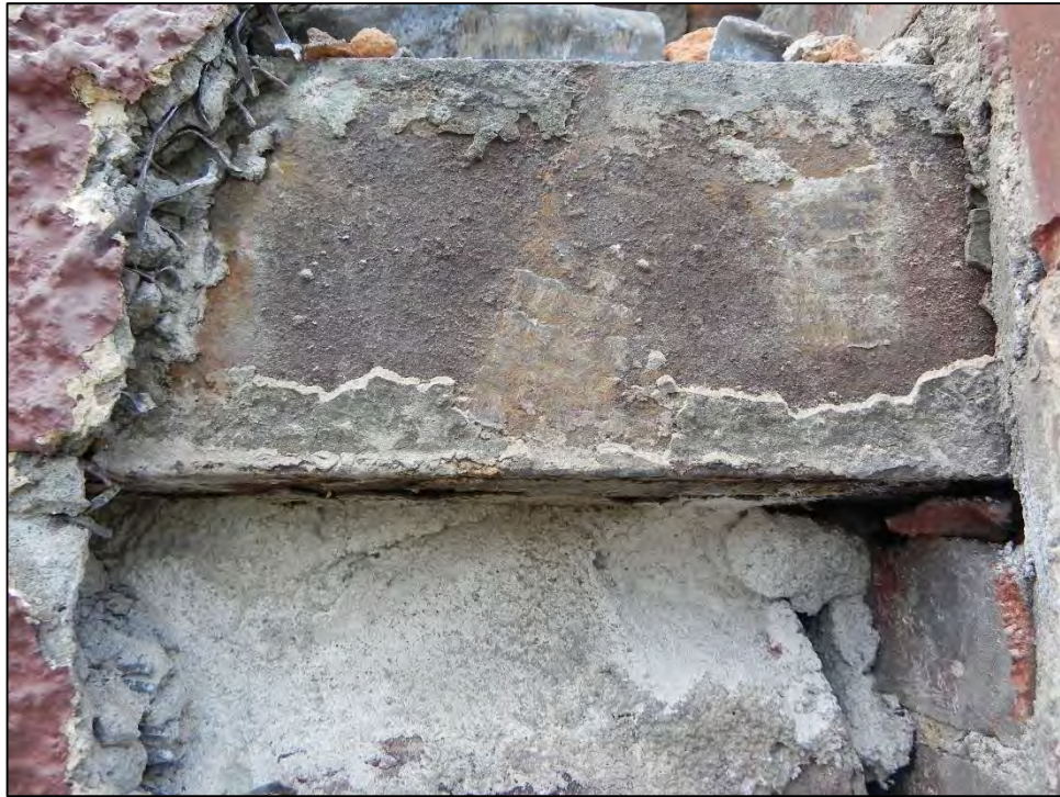
Photo 5: Detail of steel support beam above transom area of north storefront at primary north elevation. Exposed following exploratory demolition.
