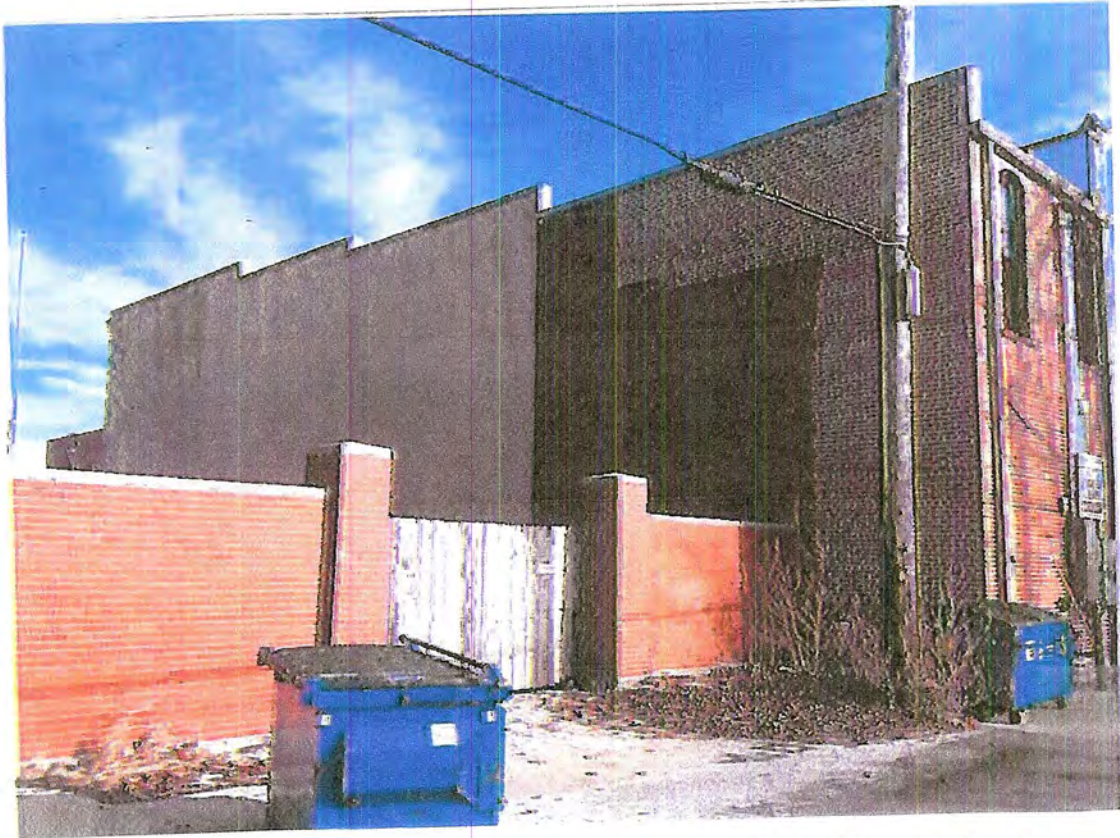
PHOTO # 3: BLAINE STREET LOOKING EAST TO ADJACENT BUILDING.
