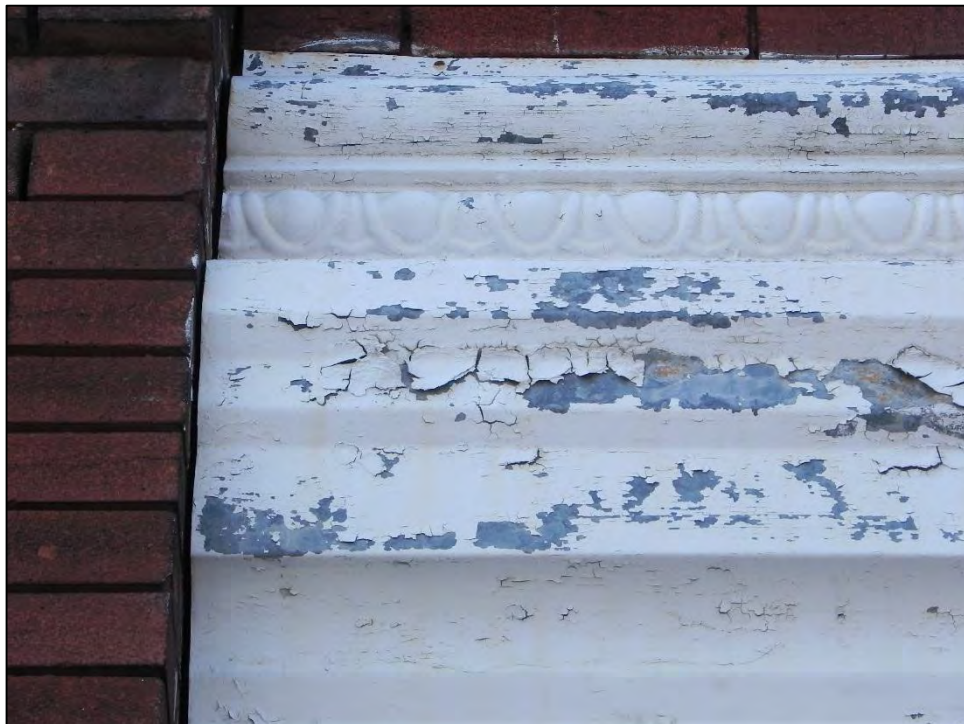
Photo 10: 308 East Commercial Street. Detail of original metal cornice above transom area of storefront at primary north elevation.
