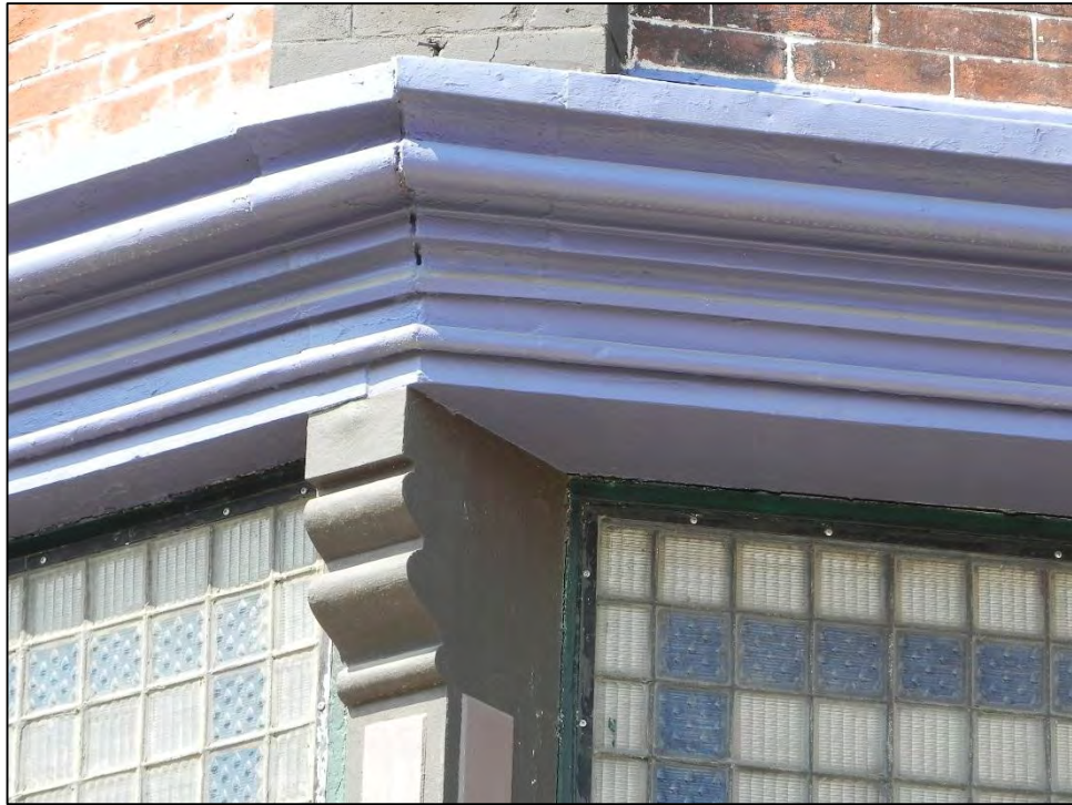
Photo 11: 234 East Commercial Street. Detail of original metal cornice above transom area of storefront at primary north elevation.
