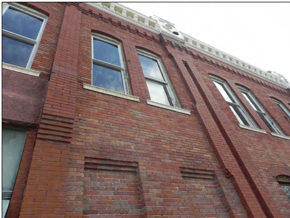
Photo 8: Detail of brickwork on north end of primary west elevation.
