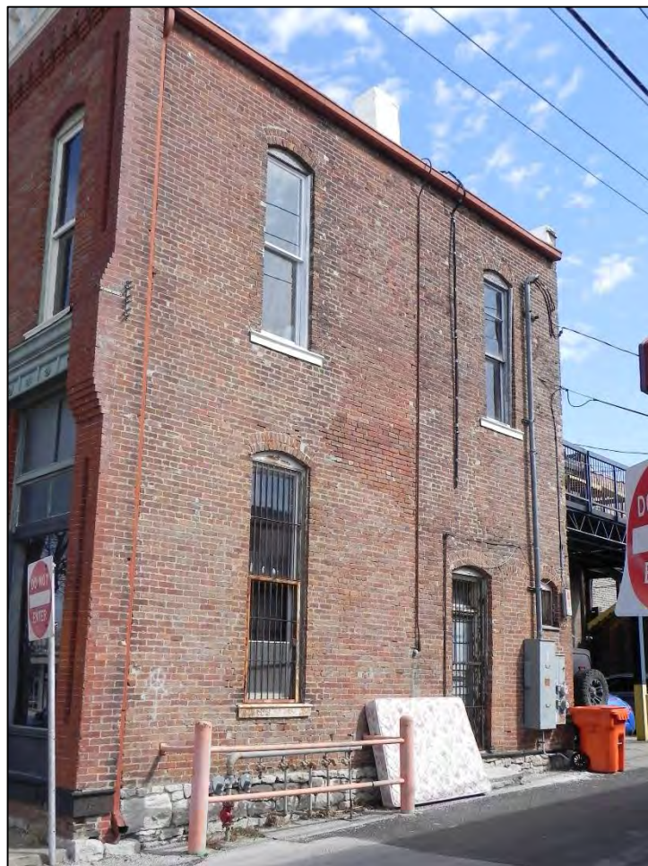
Photo 4: Rear south elevation.
