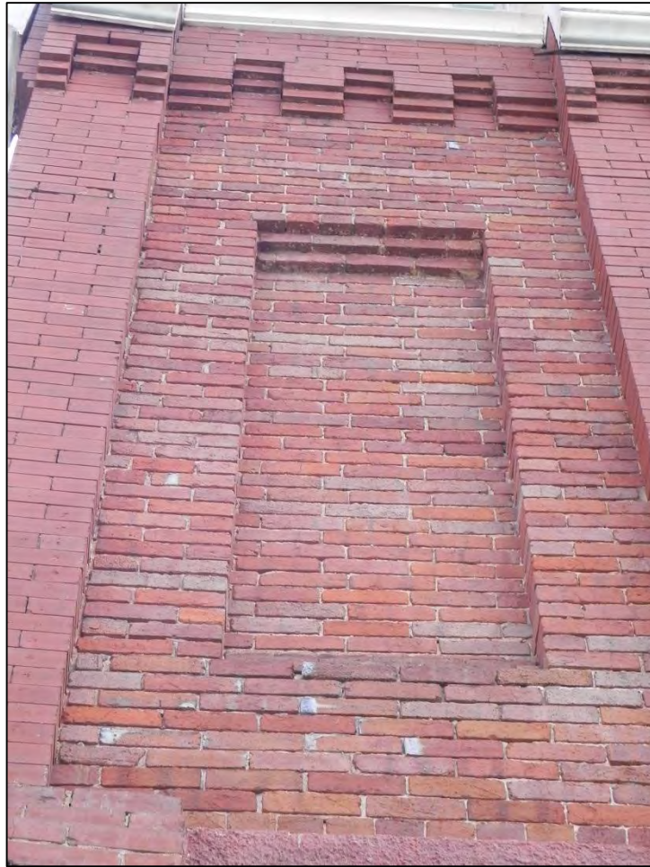
Photo 7: Detail of brickwork on north end of second story of primary west elevation.
