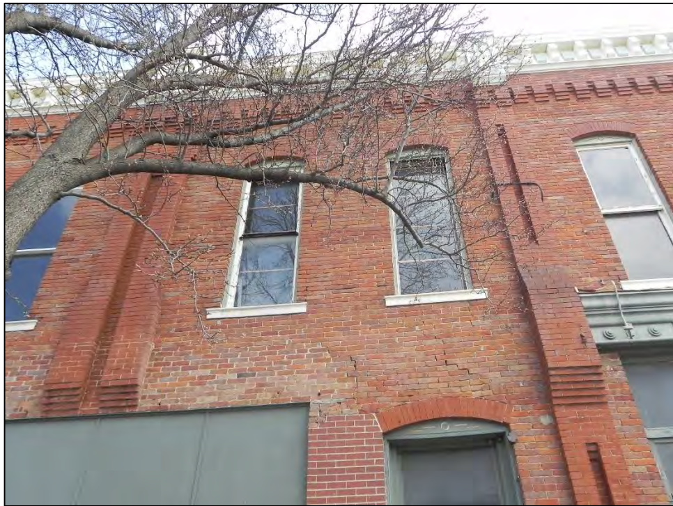
Photo 22: Detail of windows at second story of primary north elevation.
