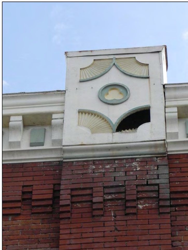
Photo 16: Detail of metal ornamentation at brick pilaster on primary west elevation.
