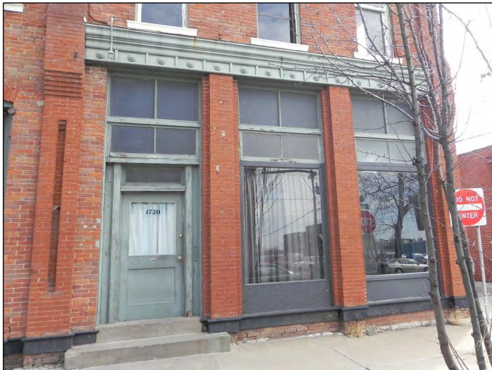
Photo 32: Detail of storefront at south end of primary west elevation.
