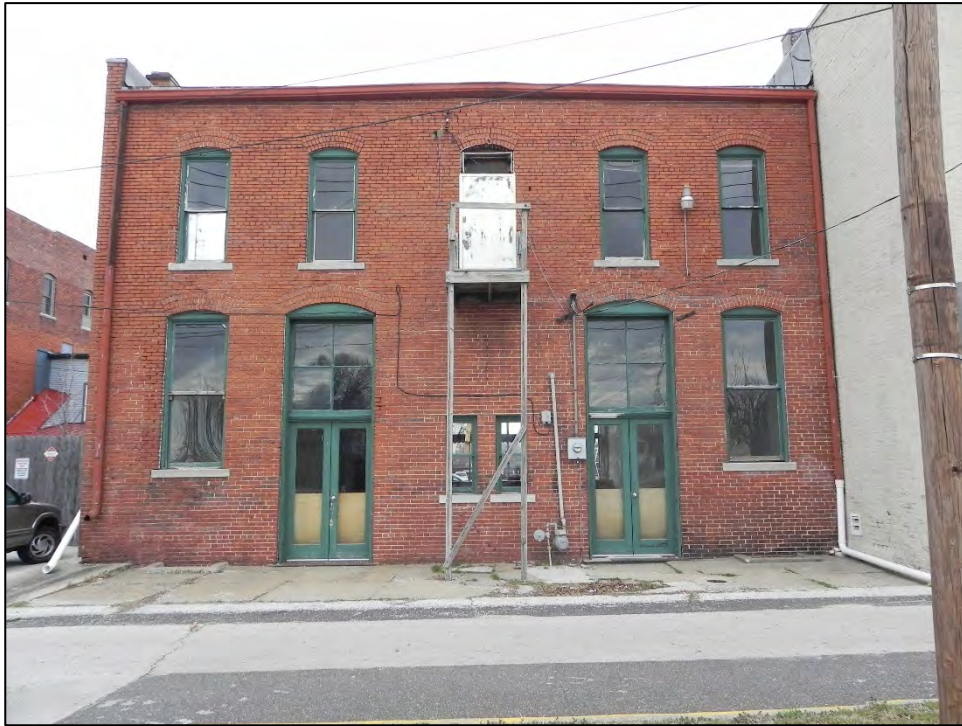
Photo 3: Rear south elevation.
