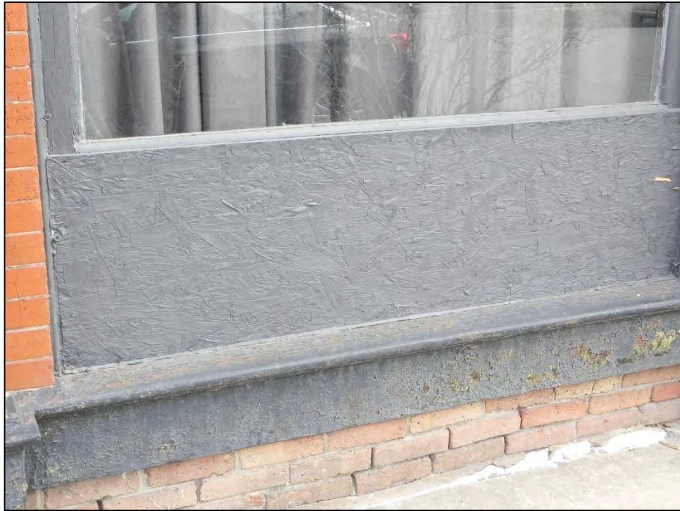
Photo 33: Detail of bulkhead of storefront at south end of primary west elevation.
