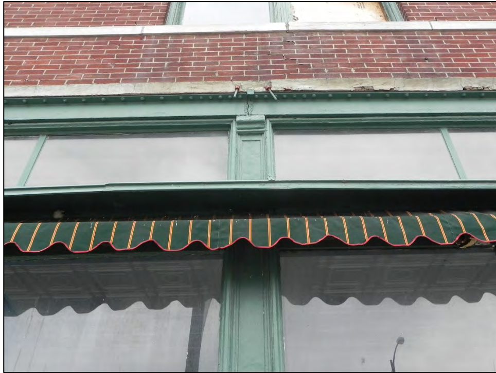
Photo 17: Detail of transoms and cast iron column at center of storefront at primary north elevation.
