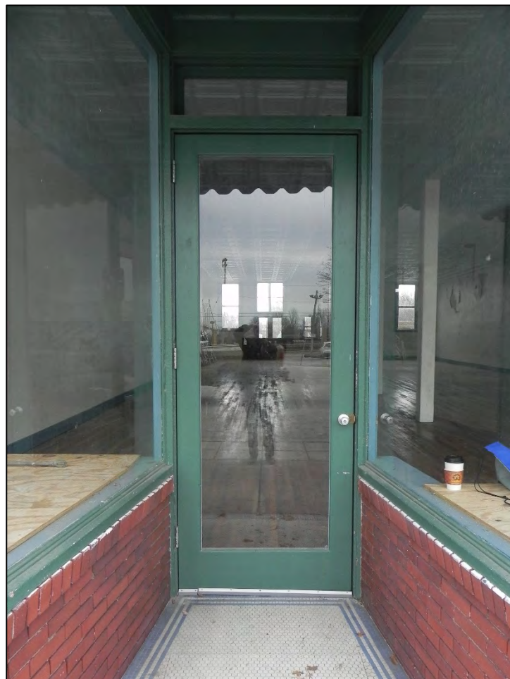
Photo 18: Detail of recessed entrance, with tile floor and modern wood door and transom, at storefront at primary north elevation.
