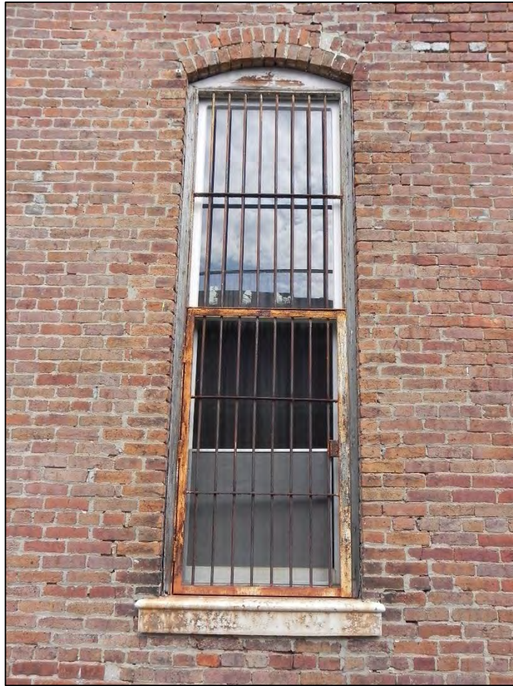
Photo 23: Detail of window at left of first story of rear south elevation.
