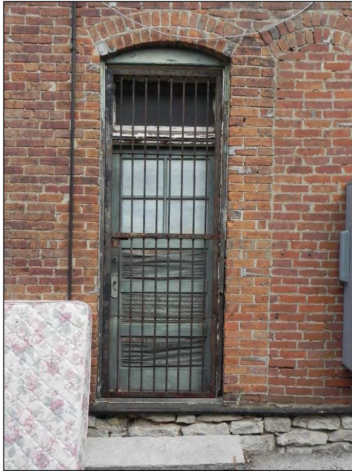
Photo 35: Detail of single door at rear south elevation.
