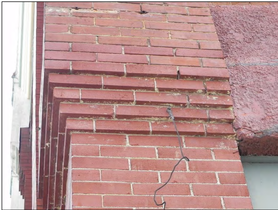
Photo 6: Detail of brickwork on pilaster at northwest corner.
