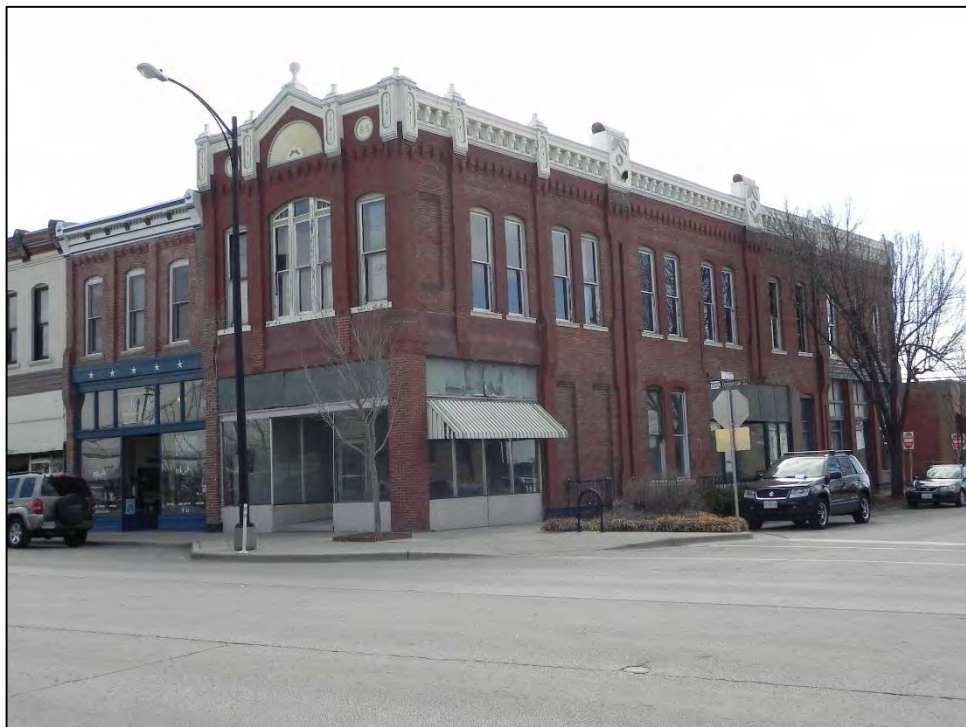
Photo 2: Primary north and west elevations.
