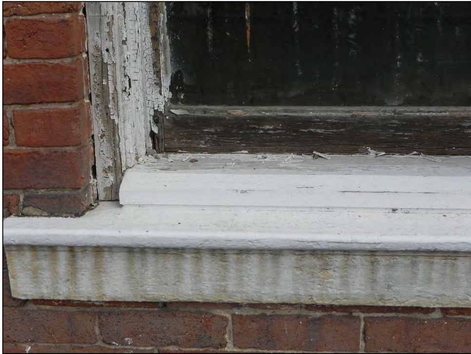
Photo 21: Detail of typical window at primary west elevation.
