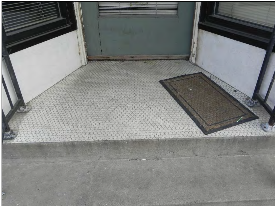
Photo 30: Detail of tiled floor or recessed entrance of center storefront at primary west elevation.
