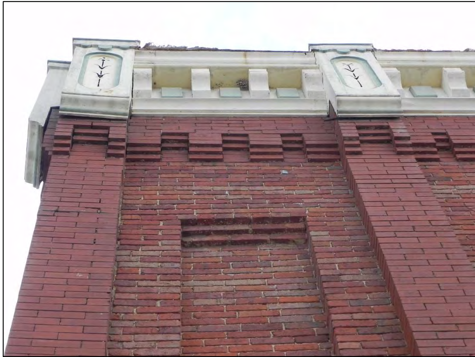
Photo 15: Detail of metal ornamentation at north roofline of primary west elevation.
