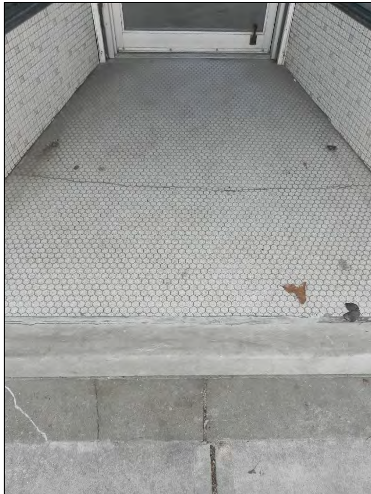
Photo 26: Detail of tiled floor of recessed entrance at storefront of primary north elevation..
