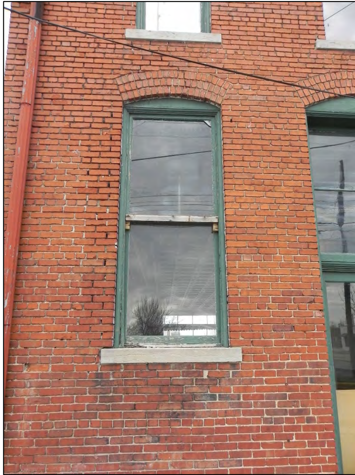
Photo 7: Detail of brickwork at first story of rear south elevation.
