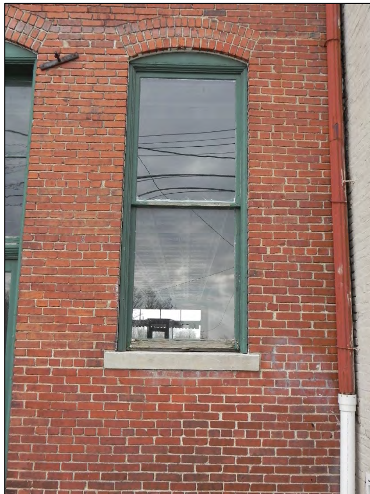
Photo 12: Detail of double-hung window at right of first story of rear south elevation.
