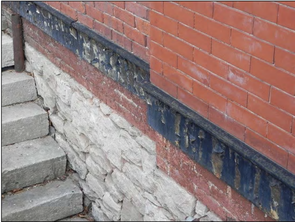
Photo 11: Detail of limestone foundation at stairwell on primary west elevation.
