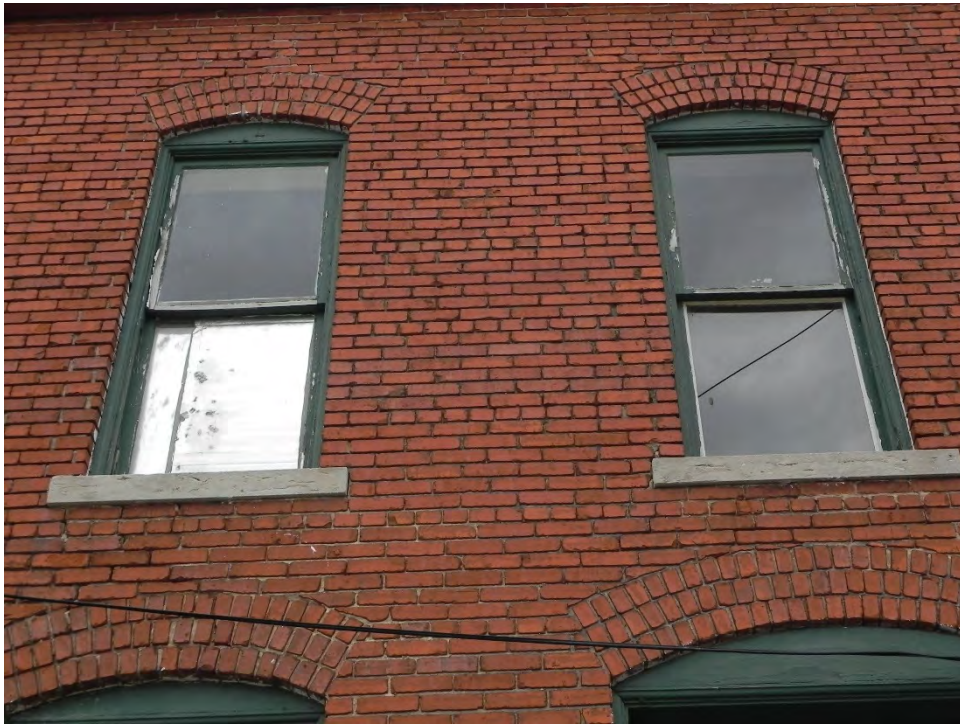
Photo 13: Detail of double-hung windows at left of second story of rear south elevation.
