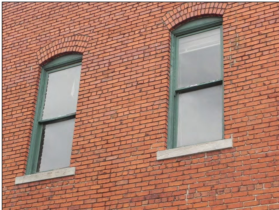
Photo 6: Detail of brickwork at second story of side west elevation.
