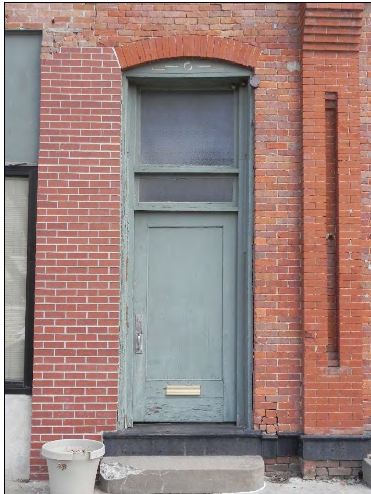
Photo 34: Detail of entrance to second story at primary west elevation.
