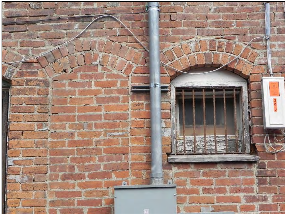
Photo 10: Detail of brickwork at first story of rear south elevation.
