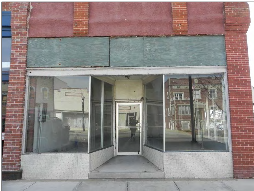
Photo 24: Detail of storefront at primary north elevation.
