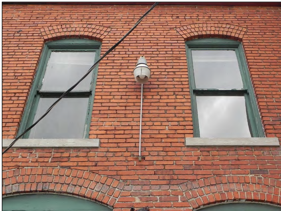
Photo 8: Detail of brickwork at second story of rear south elevation.
