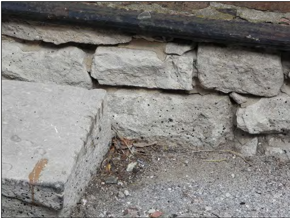
Photo 12: Detail of limestone foundation at rear south elevation.
