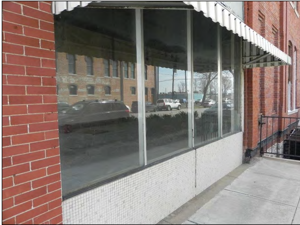
Photo 27: Detail of storefront at north end of primary north elevation.
