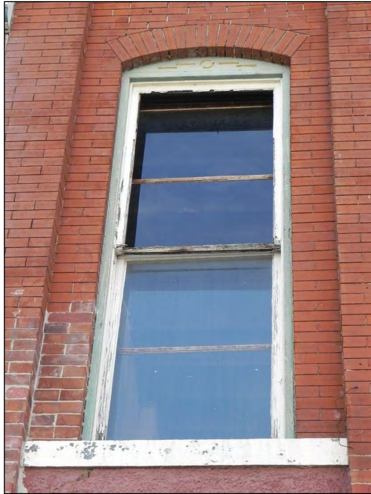
Photo 19: Detail of single window at left of second story of primary north elevation.
