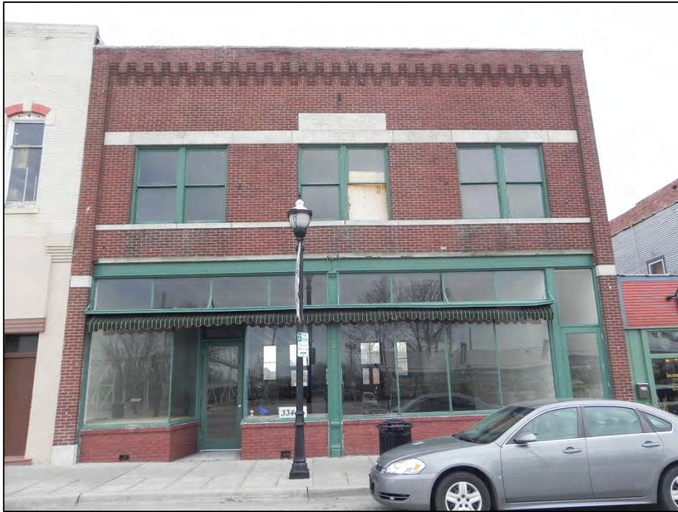
Photo 1: Primary north elevation.
