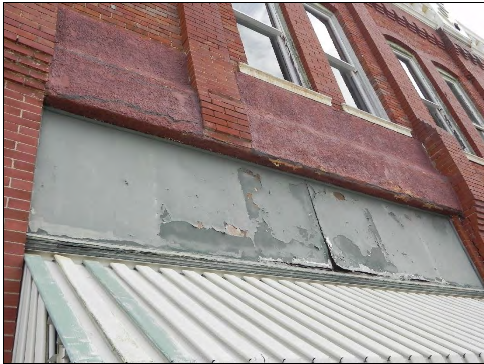
Photo 28: Detail of transom area above storefront at north end of primary west elevation.
