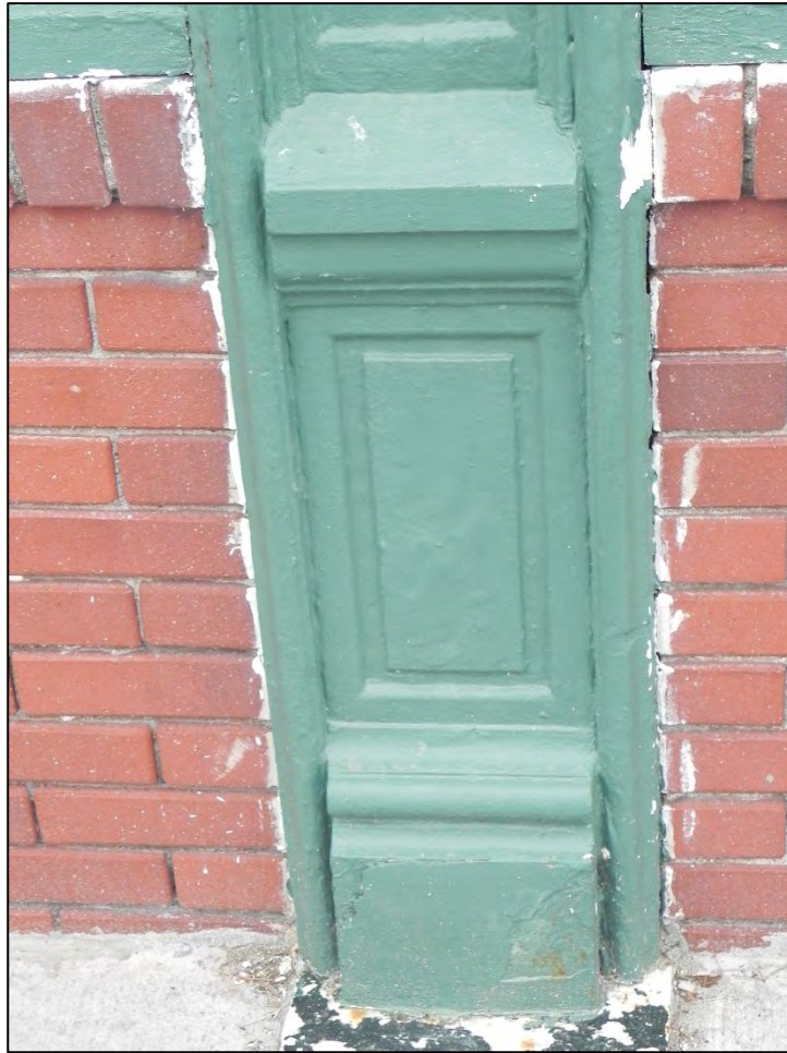
Photo 5: Detail of brickwork of storefront bulkhead at primary north elevation.
