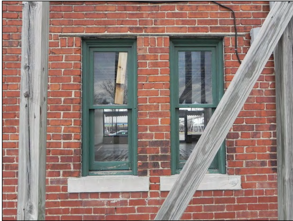
Photo 11: Detail of paired double-hung windows at center first story of rear south elevation.
