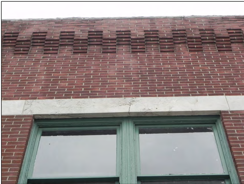
Photo 4: Detail of brickwork at second story of primary north elevation.
