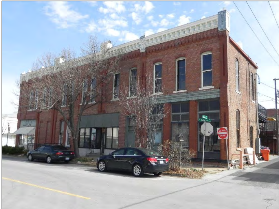
Photo 3: Primary west elevation.
