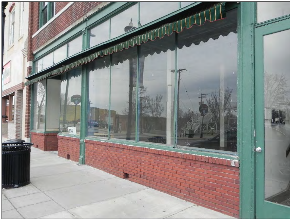
Photo 14: Detail of storefront at primary north elevation.
