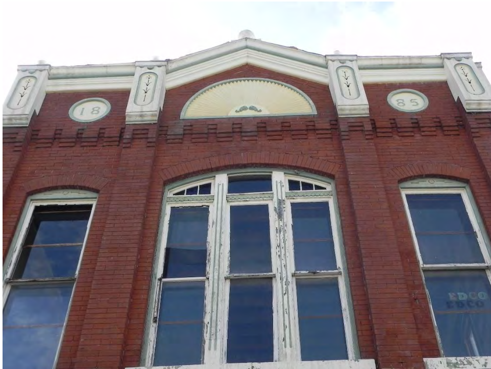
Photo 5: Detail of second story of primary north elevation.
