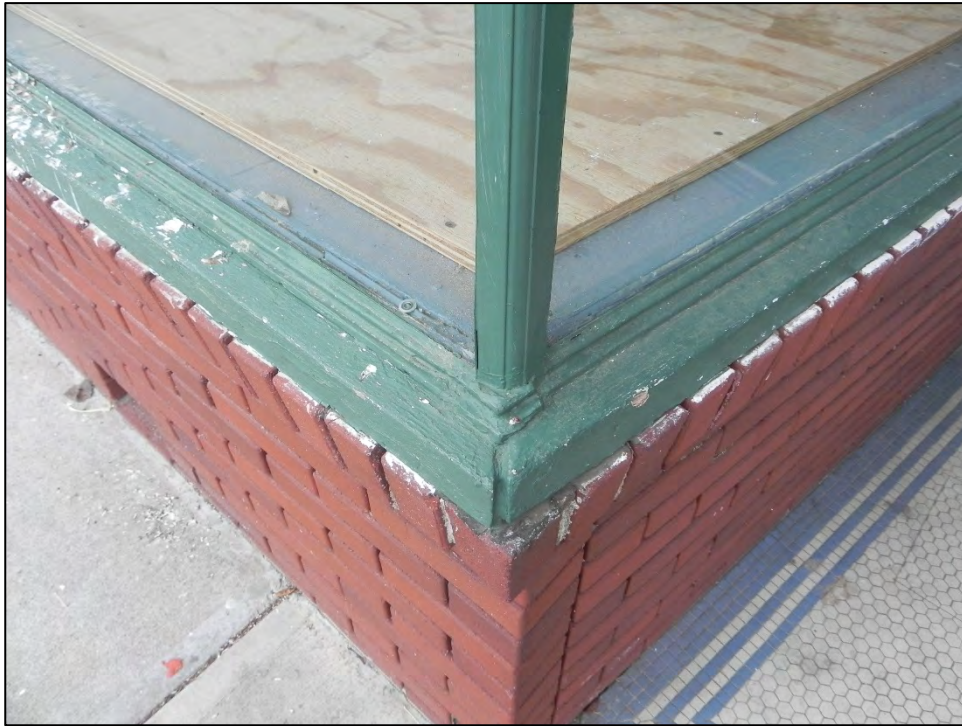
Photo 15: Detail of brick bulkhead at recessed entrance of storefront at primary north elevation.
