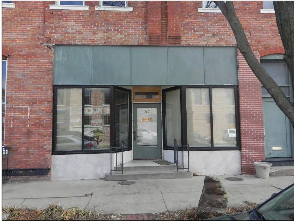
Photo 29: Detail of center storefront at primary west elevation.
