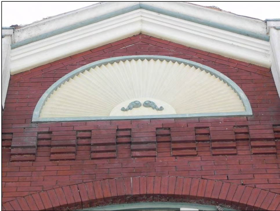
Photo 14: Detail of metal ornamentation at center second story of primary north elevation.
