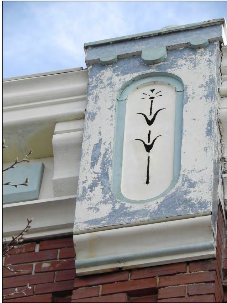
Photo 17: Detail of metal ornamentation on pilaster on primary west elevation.
