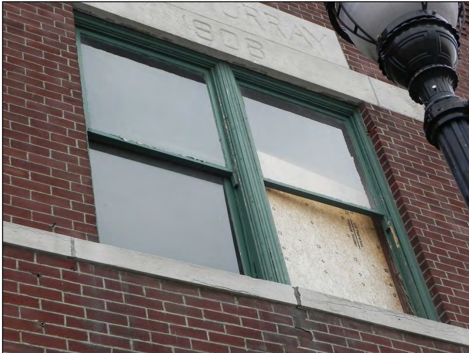
Photo 10: Detail of paired double-hung windows at center of second story of primary north elevation.
