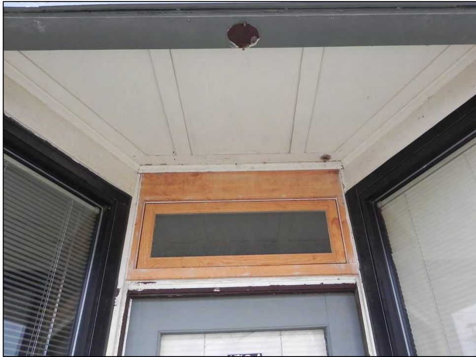
Photo 31: Detail of transom at recessed entrance of center storefront of primary west elevation.
