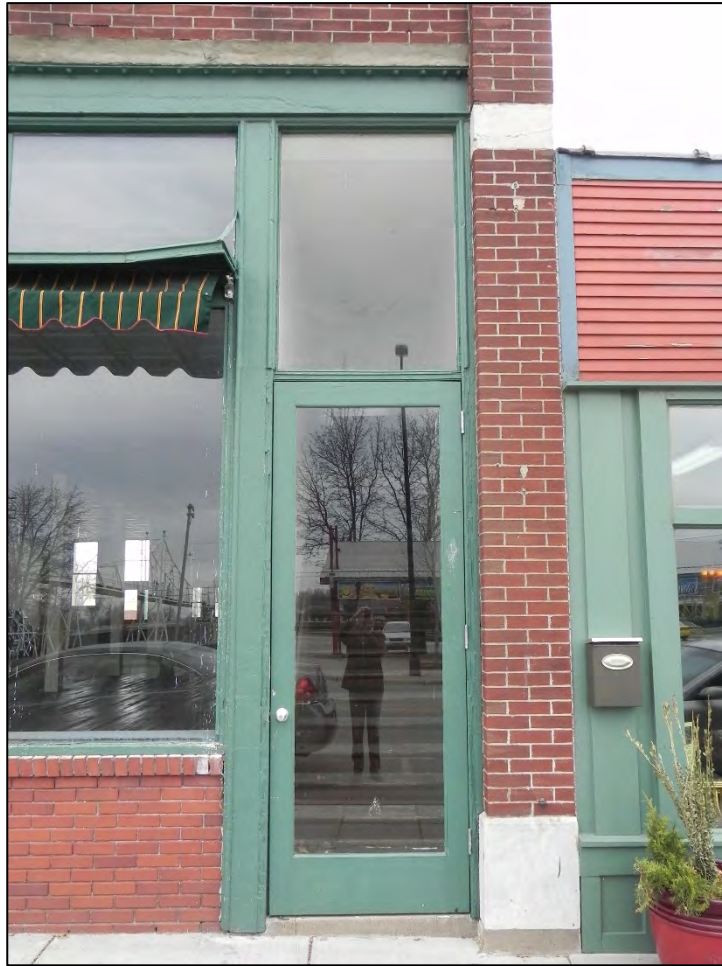
Photo 19: Detail of modern wood door and transom at second story entrance at right end of primary north elevation.
