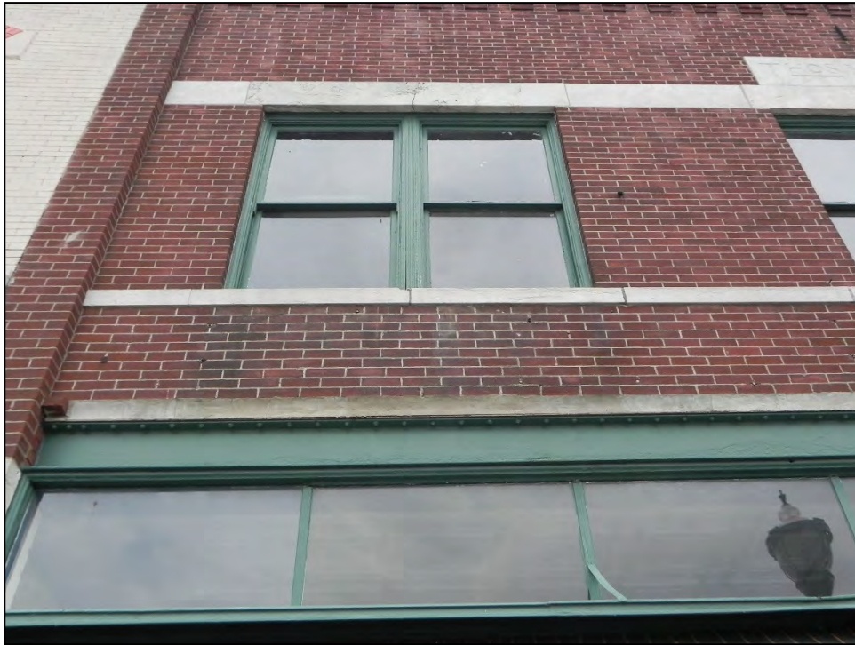
Photo 9: Detail of paired double-hung windows at left of second story of primary north elevation.
