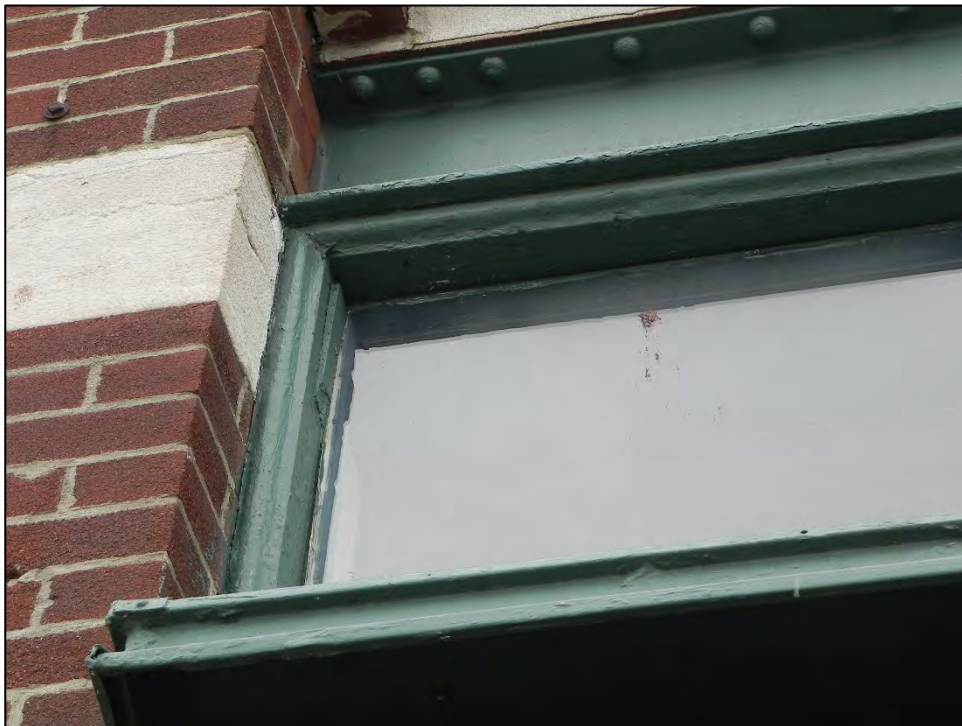
Photo 16: Detail of transom above left end of storefront at primary north elevation.
