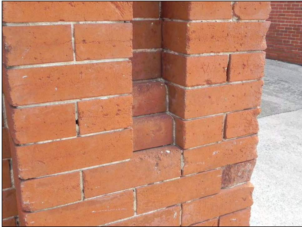
Photo 9: Detail of brickwork at south corner of primary west elevation.
