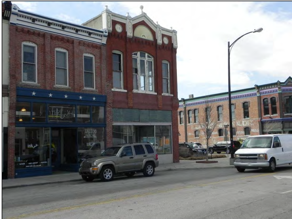
Photo 1: Primary north elevation. View to southwest.
