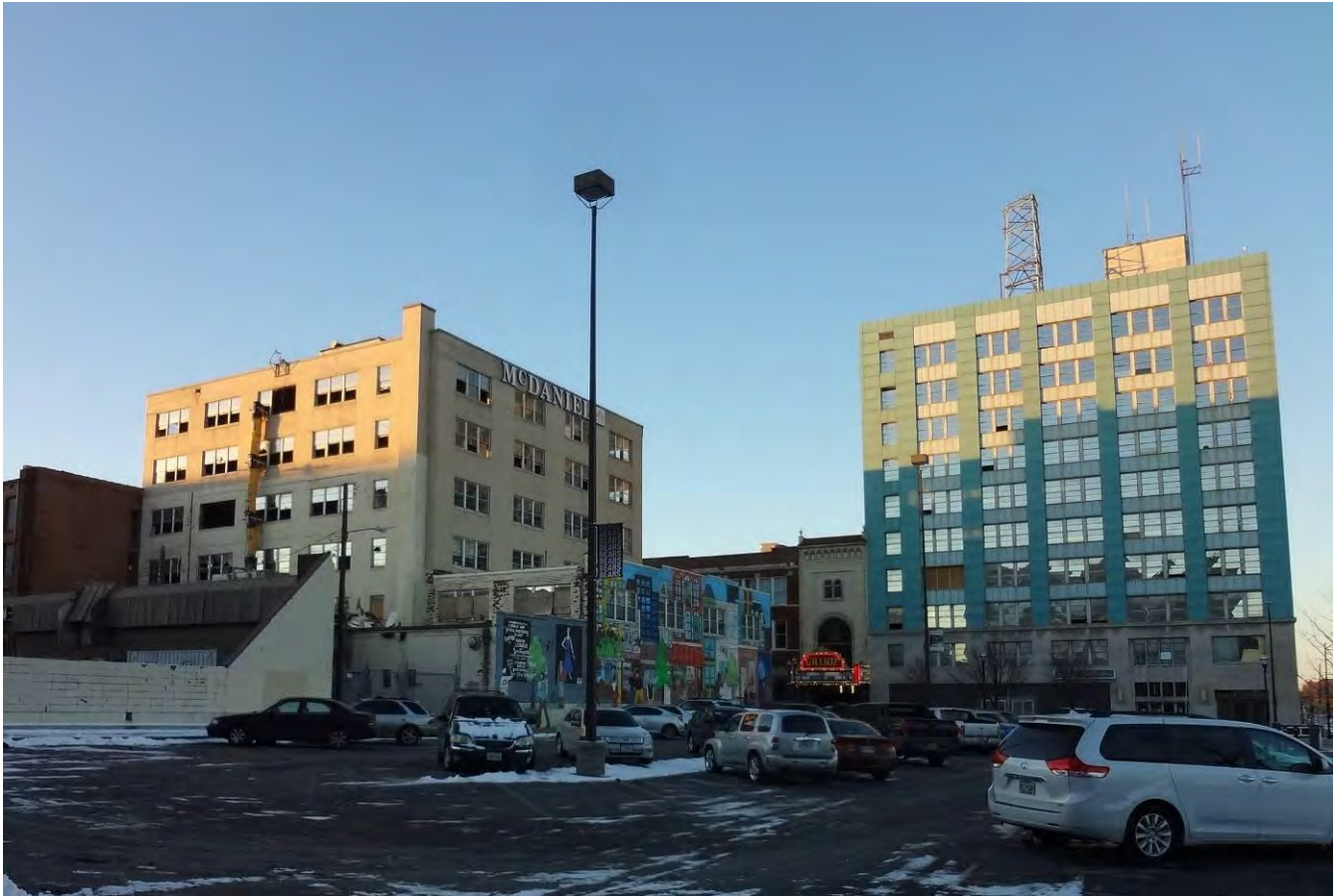
Figure 7. McDaniel and Woodruff Buildings. The Woodruff building is the large building on the right.
