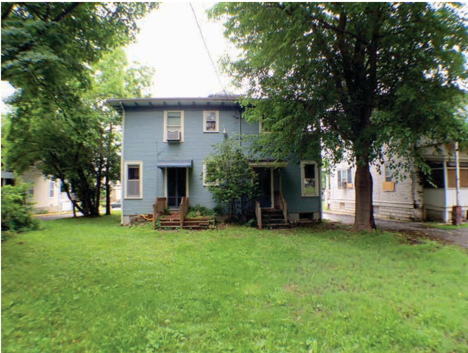
Existing Back of House
