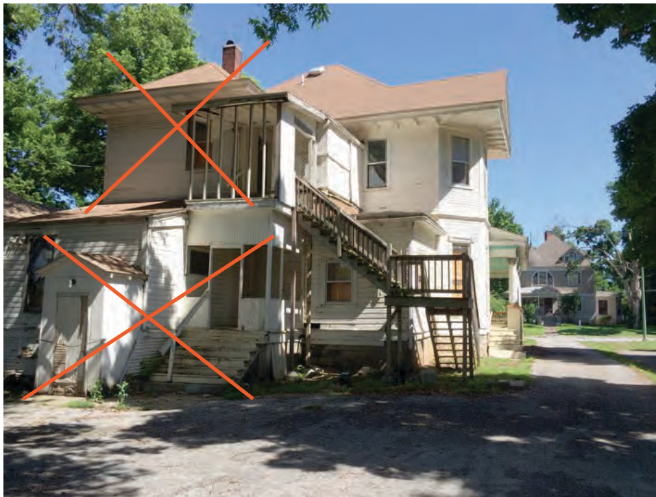
Existing Back of House
