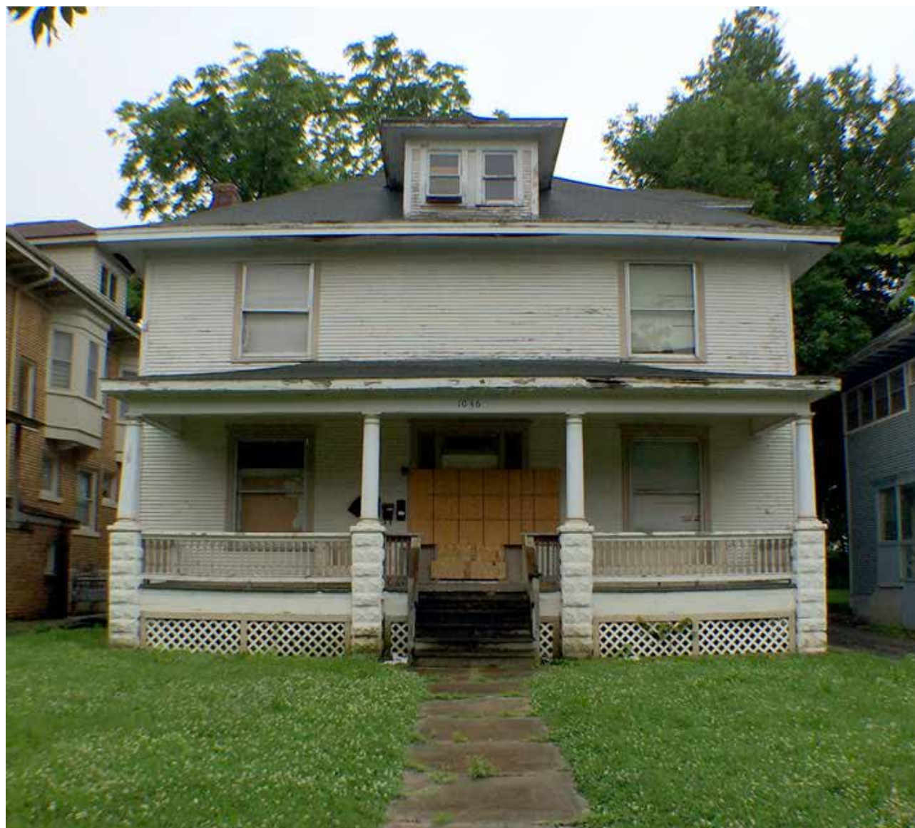
1046 E Walnut St Elevation Photo
