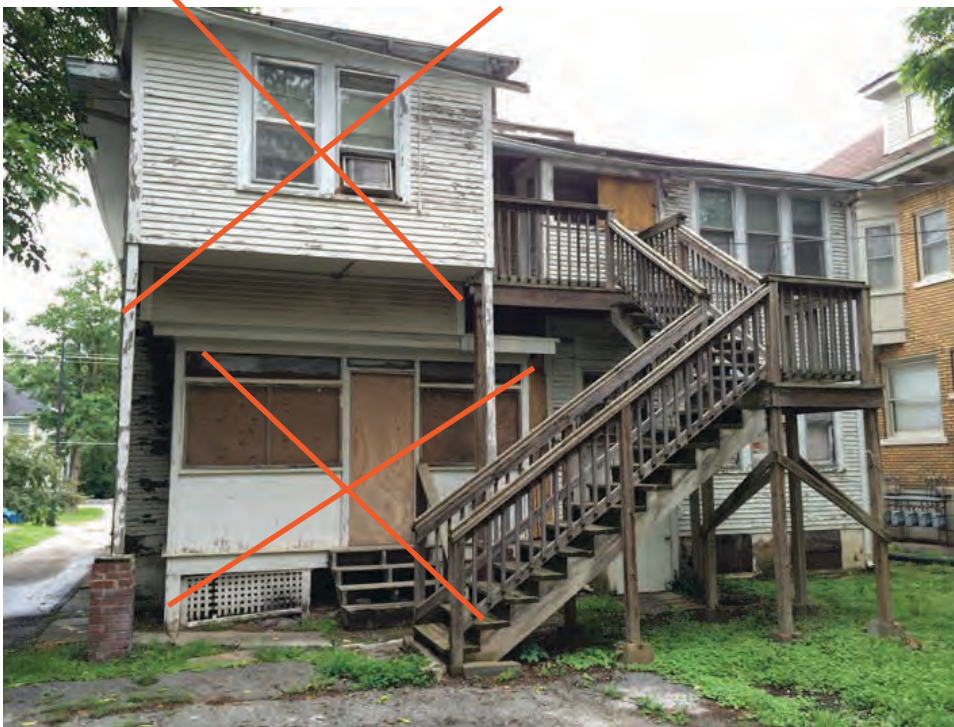
Existing Back of House
