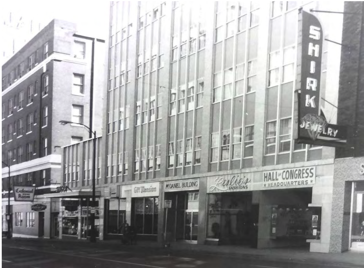
Figure 3. McDaniel Building in 1967. (Springfield Public Library Files.)
