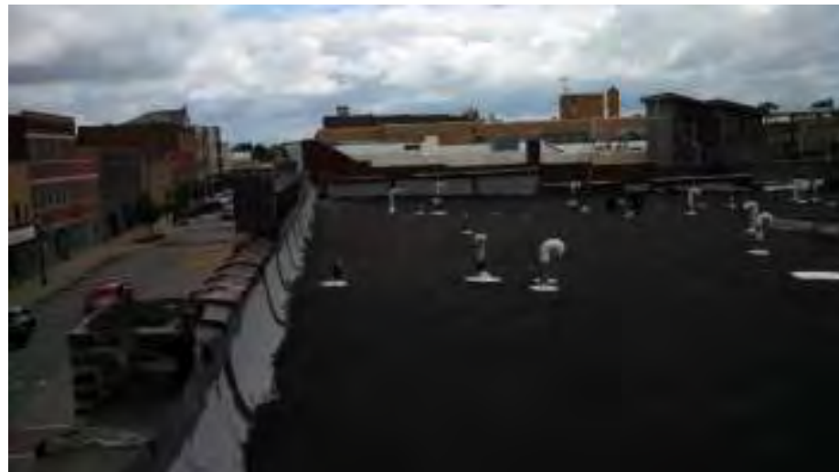
Existing Roof Looking Northwest
