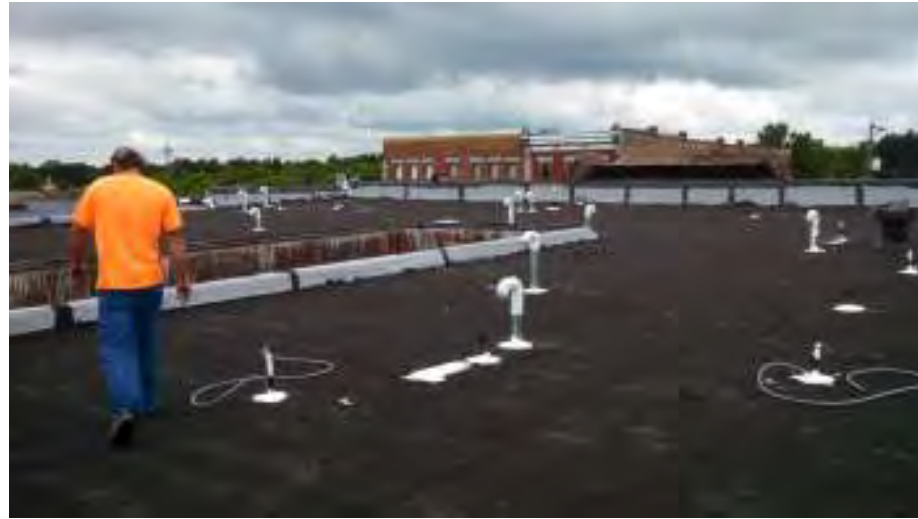
Existing Roof Looking Southwest
