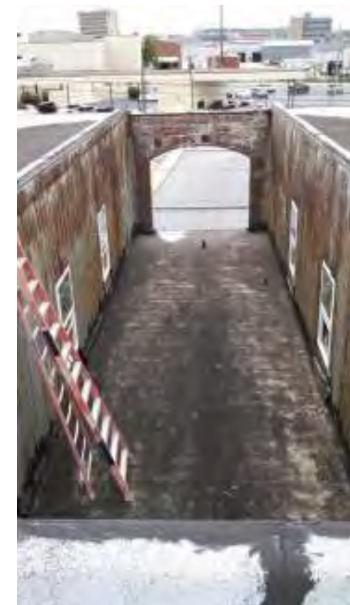
Lower Level Roof
