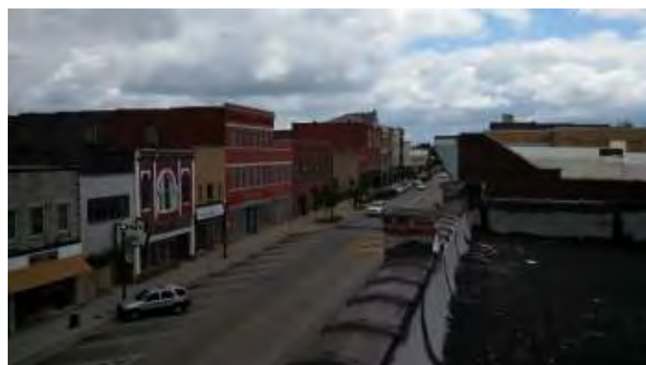
Existing Roof Looking North
