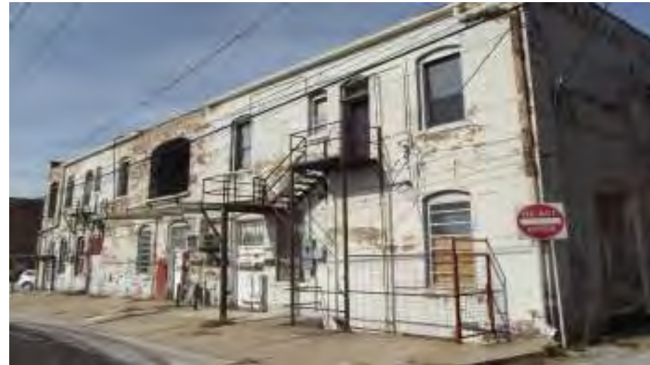
Existing Door and Balcony to Be Replaced
