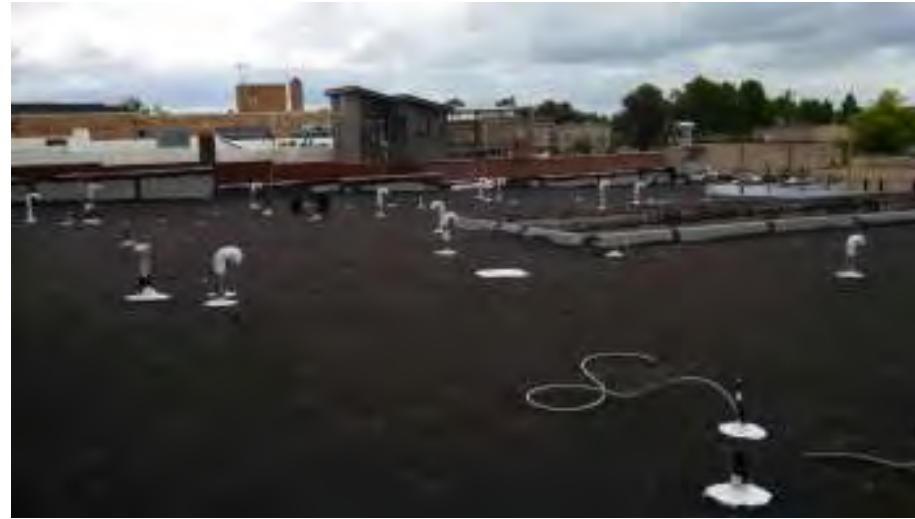
Existing Roof Looking East
