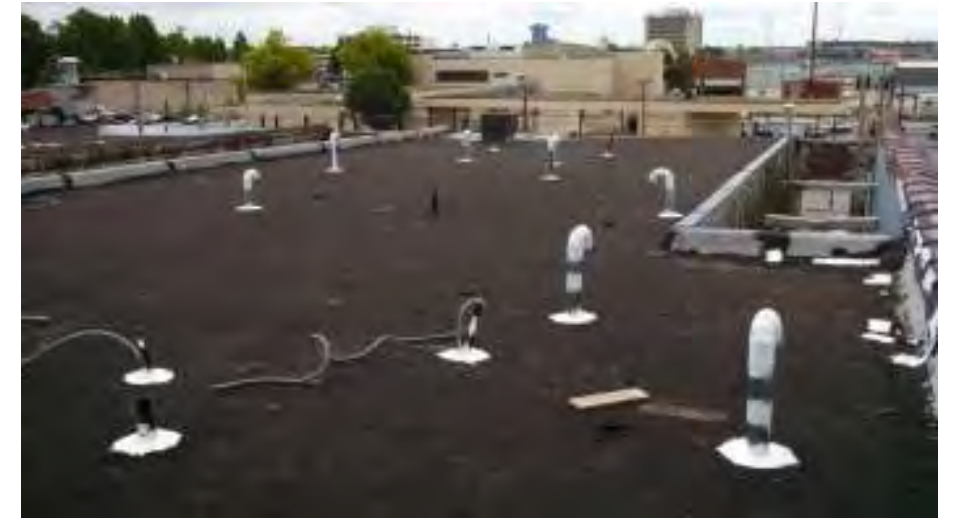
Existing Roof Looking South
