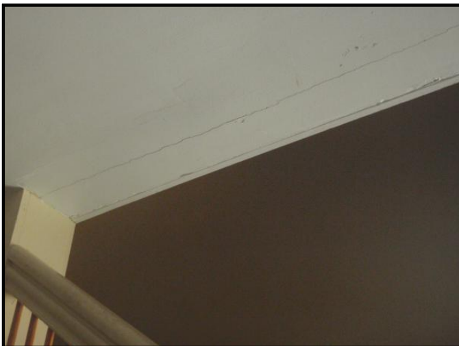
Settlement Cracks
