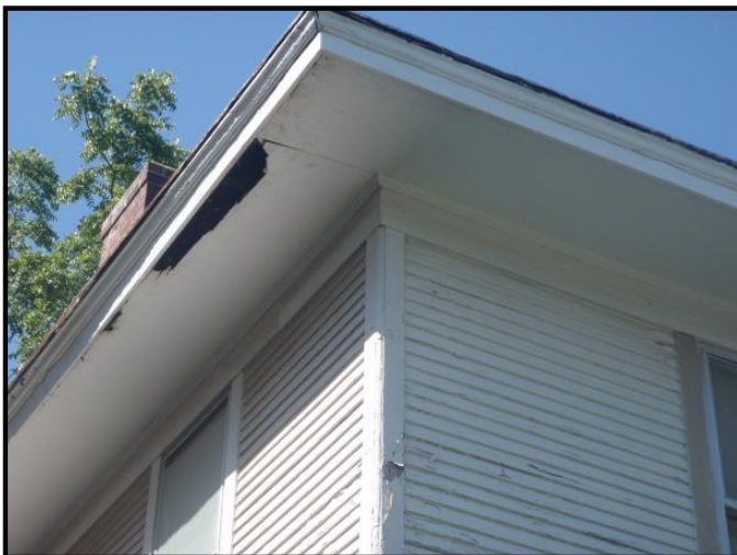
Rotting Soffit
