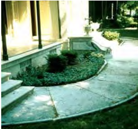
As part of a rehabilitation project, the deteriorated limestone walkways are being replaced in kind. Photo: NPS files.
