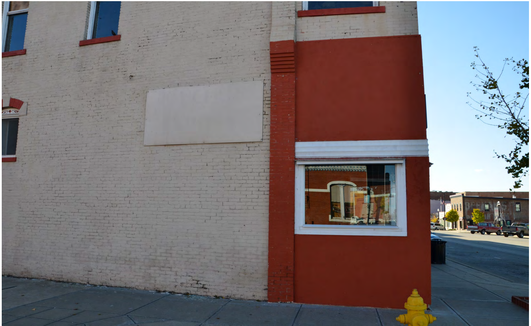
Jefferson street Before
