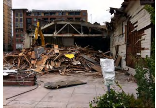
Demolition of a contributing building, 2011
