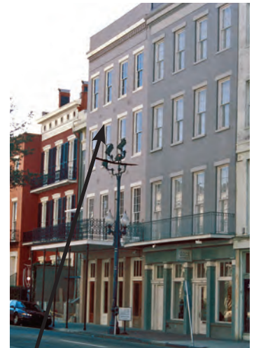
Figure 26. A rooftop addition would have negatively impacted the character of the primary facade (right) of this mid-19th century, four-story structure and the low-rise historic district. However, a third floor was successfully added on the two-story rear portion (below) of the same building with little impact to the building or the district because it blends in with the height of the adjacent building.
