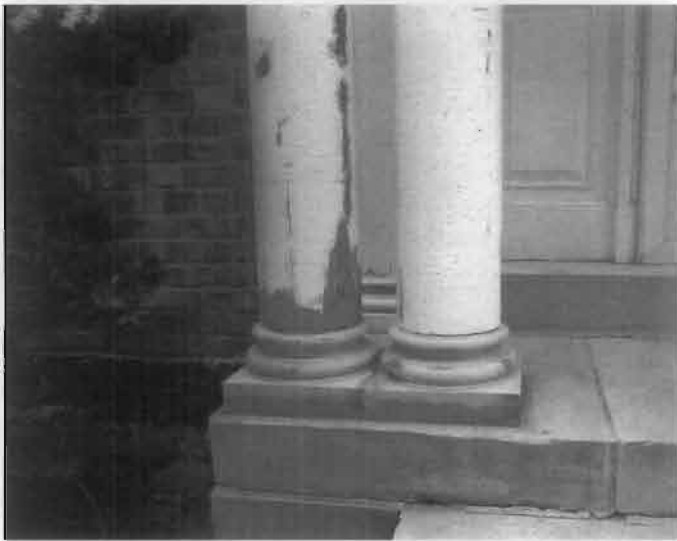
Figure 11. The lower shaft of the porch columns had decayed as water wicked up through the end grain (top). The column shafts were repaired in place by cutting out the deteriorated wood and making repairs using epoxy consolidants and fillers. (bottom). The column bases were replaced. Photos: Paul Marlowe, Marlowe Restorations.
