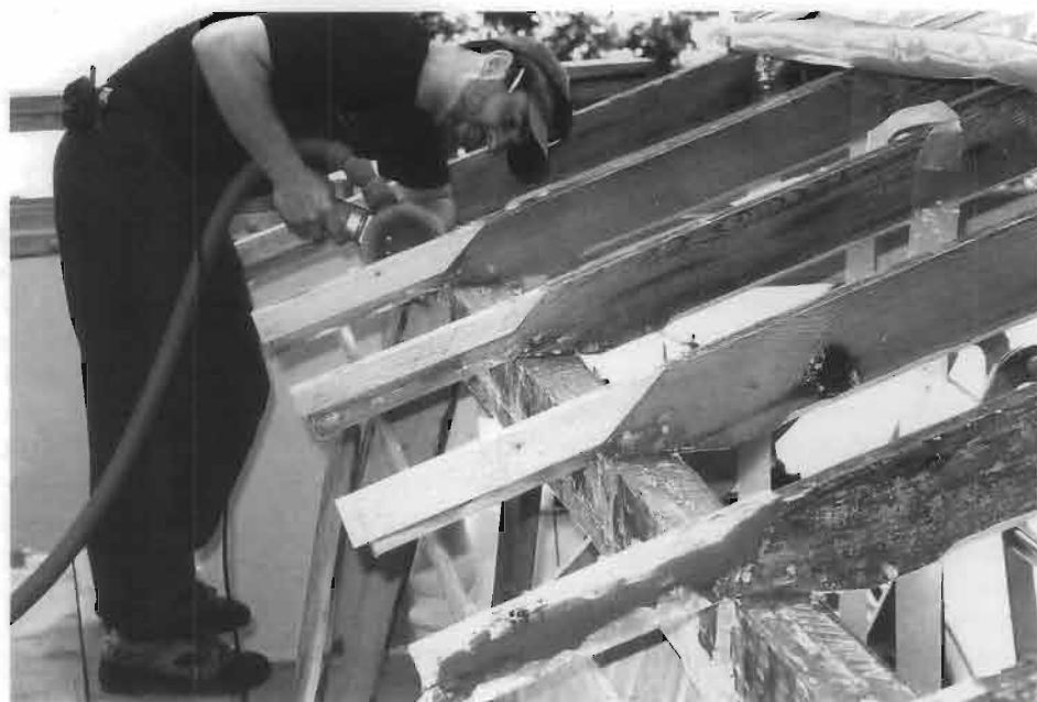
Figure 9. The ends of porch roof rafters are often susceptible to moisture decay. When concealed by a soffit or ceiling, rafters can be repaired by adding new sister boards. Where roof rafter ends are exposed, splicing new wood onto the old (dutchman repair) and use of epoxy consolidants and fillers both preserve sound historic fabric while retaining the historic appearance.
