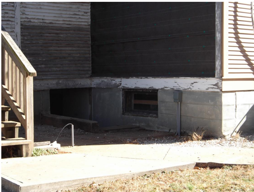
Basement Entry at the Northwest Corner
