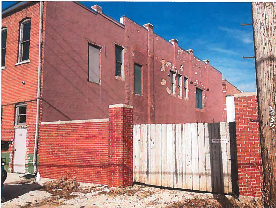
Photo 2: Blaine Street looking towards the courtyard and the East wall of the F.W. Woolworth Building. The existing brick half-wall and wood gate shall be removed.
