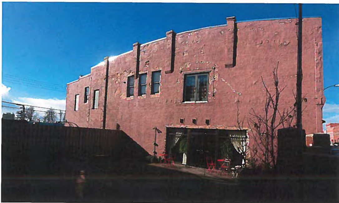
Photo 4: In the courtyard space looking at the East wall of the F.W. Woolworth Building.
