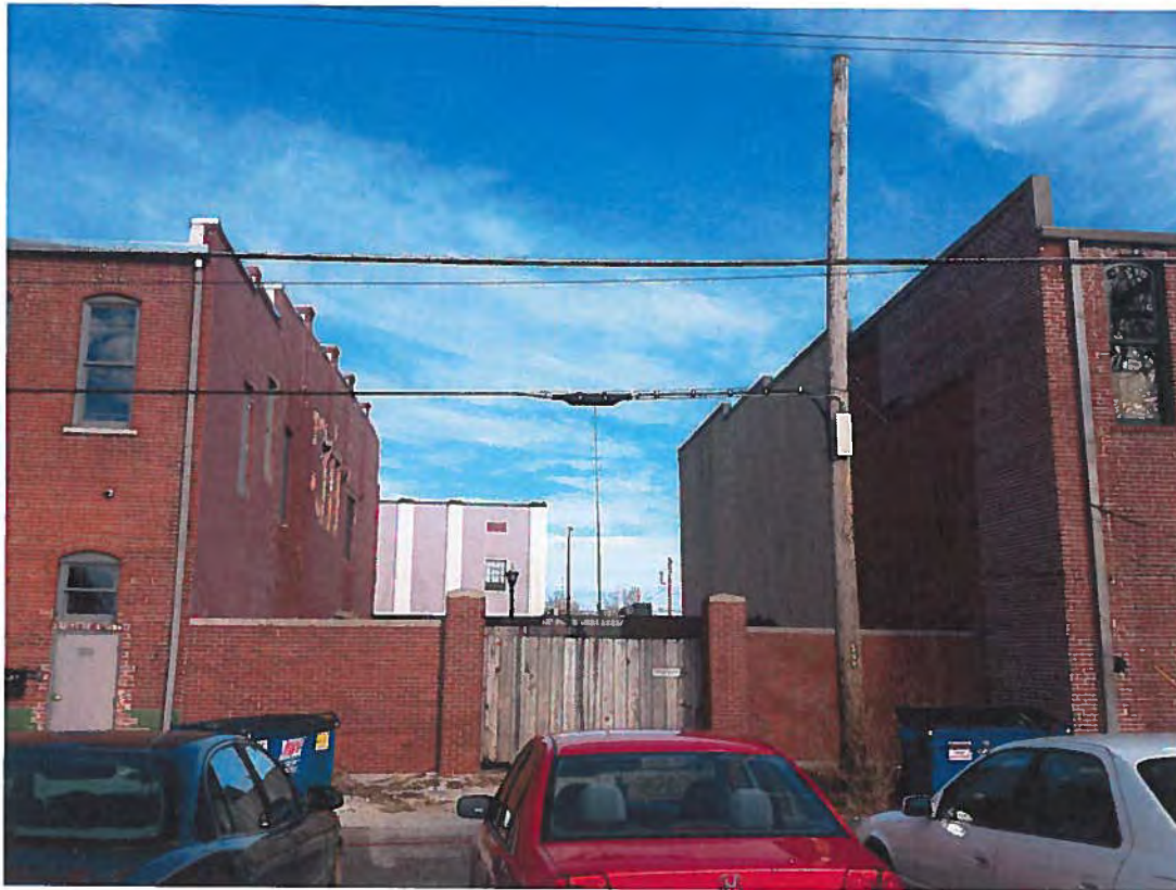
Photo 3: Looking North at the existing courtyard space and the full brick half-wall and gate to be removed.
