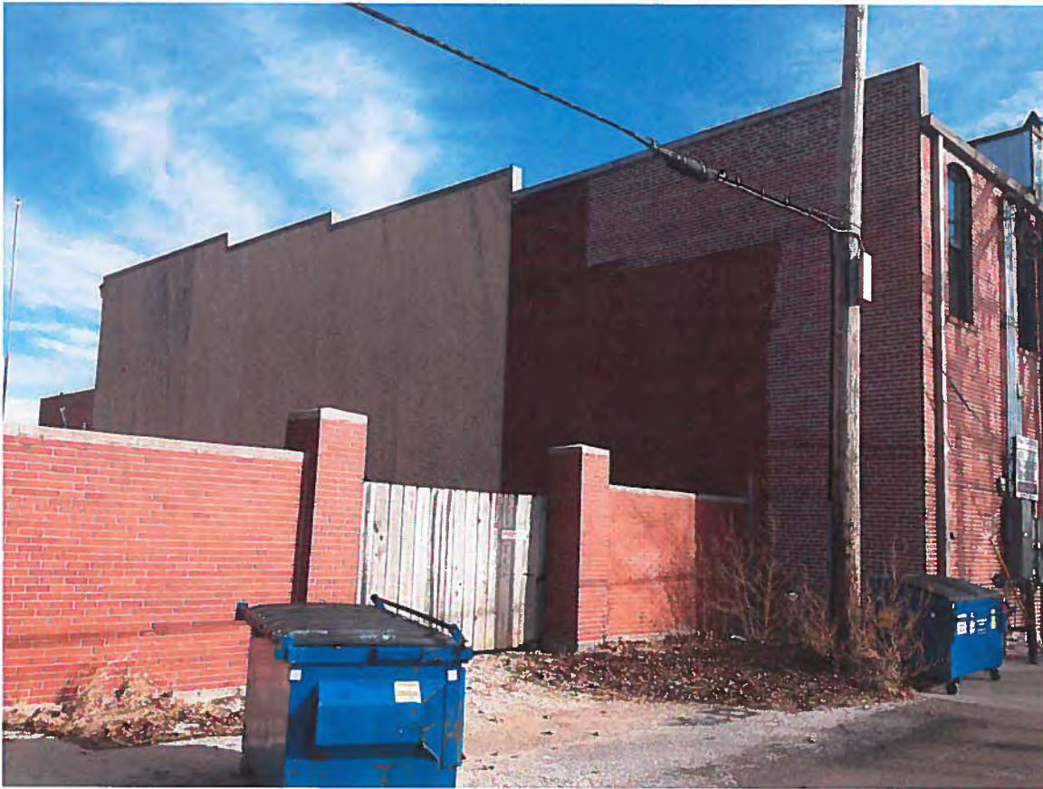
Photo 5: Blaine Street looking towards the adjacent building and existing brick half-wall to be removed.
