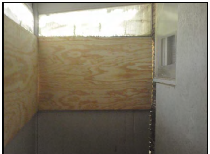
Screened in Patio
