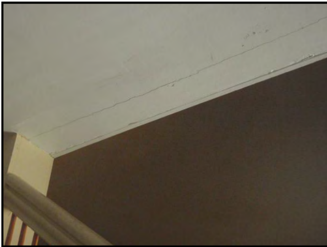
Settlement Cracks
