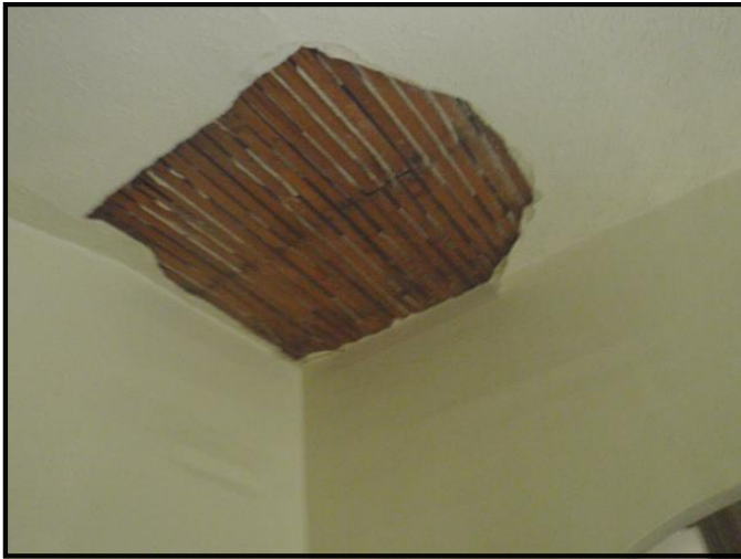
Unit #2 Kitchen Ceiling
