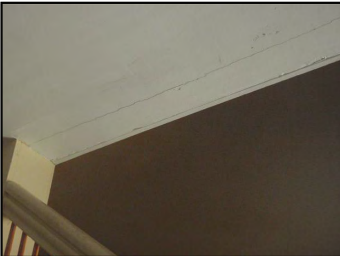
Settlement Cracks
