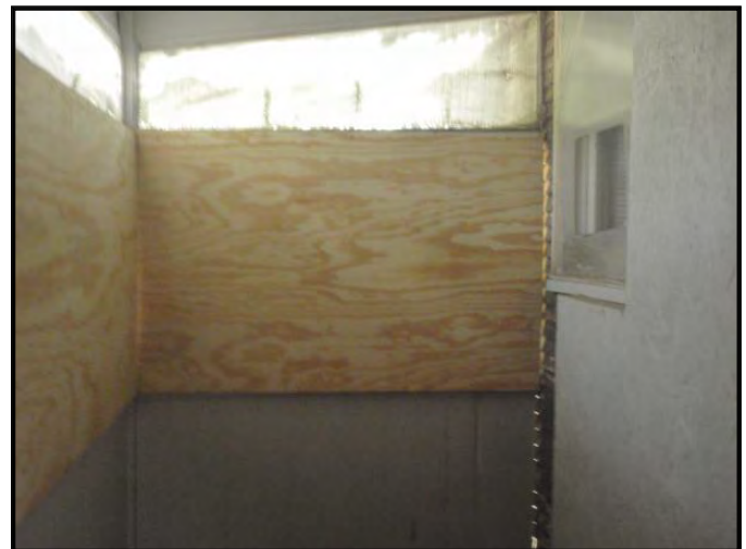
Screened in Patio
