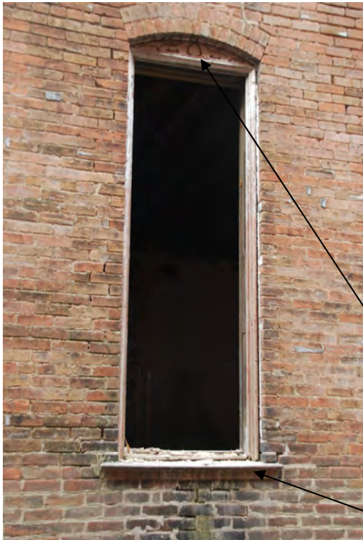
Image P7—Typical existing window east elevation
