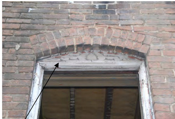
Image P8—Typical existing window head trim
