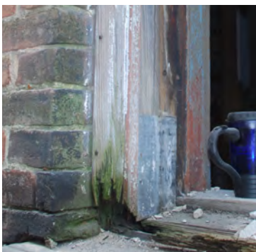
Images P9- All existing wood windows exhibit areas of rotted beyond restoration
