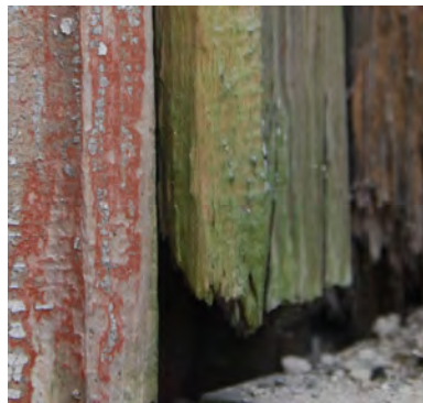
Images P9- All existing wood windows exhibit areas of rotted beyond restoration
