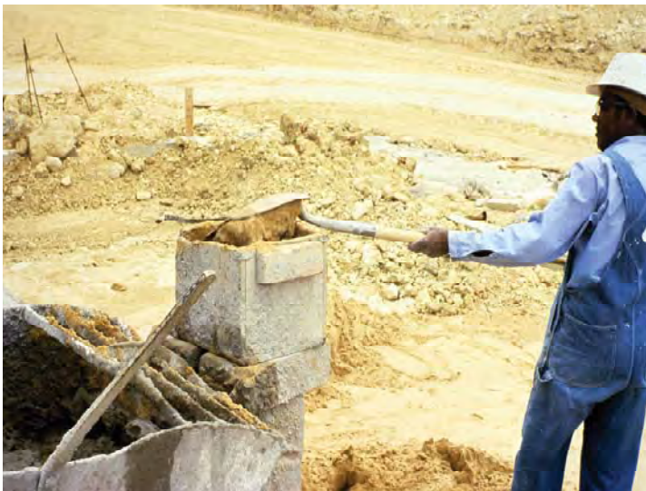
Photo 1 Obtaining Accurate Sand Quantities
