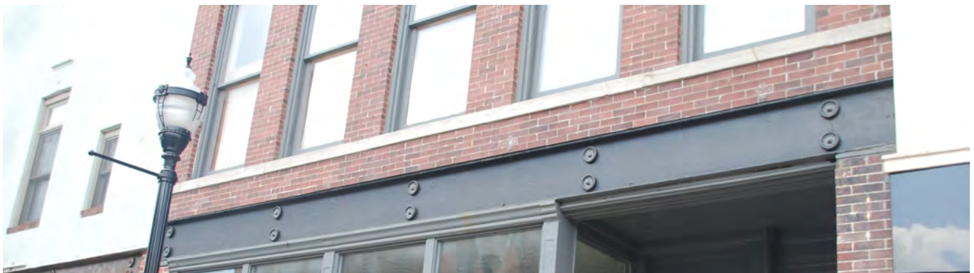
Image P12—Similar steel beam
