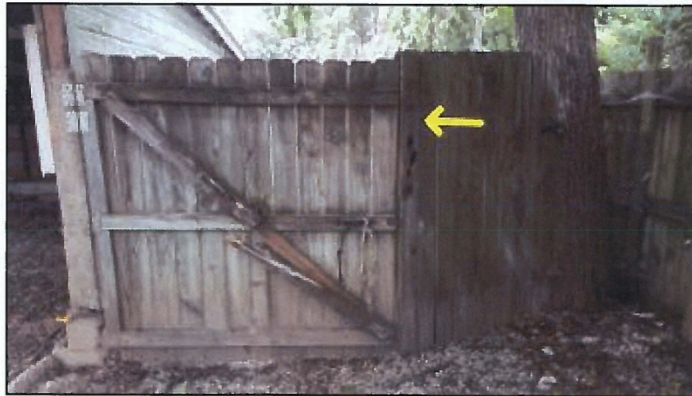
Sagging back gate
