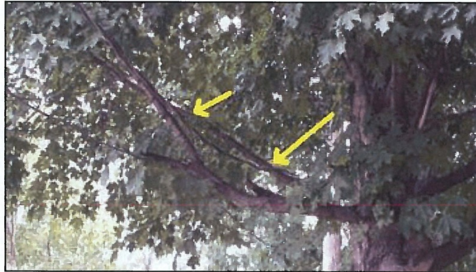
Trees touch wires
