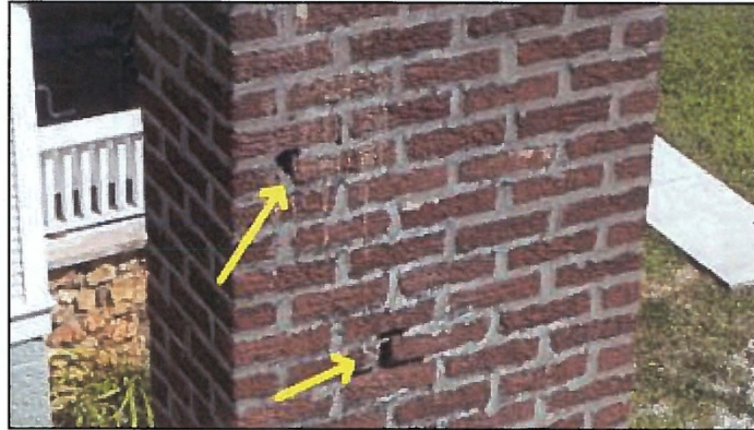
Missing mortar
