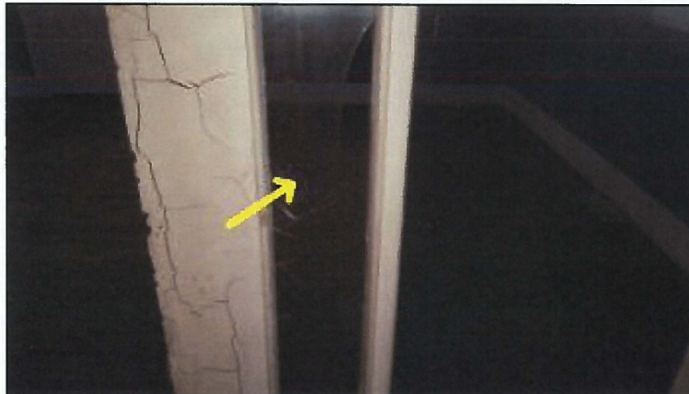
Broken glass in main living area doors.
