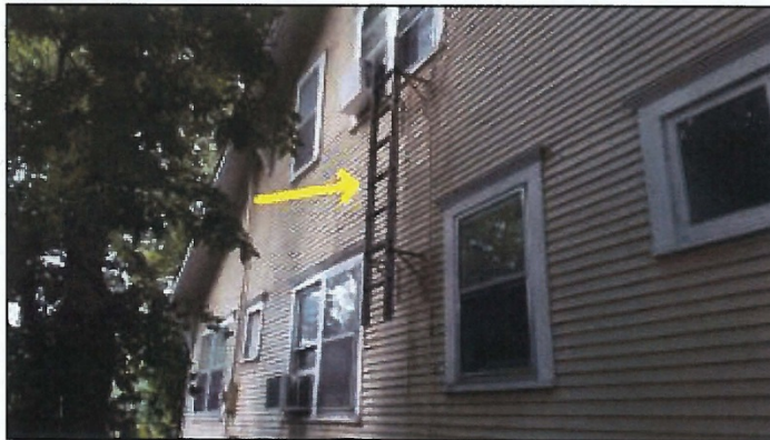
Fire escape ladder noted on East side
