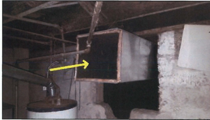
Furnace and majority of ductwork has been removed.
