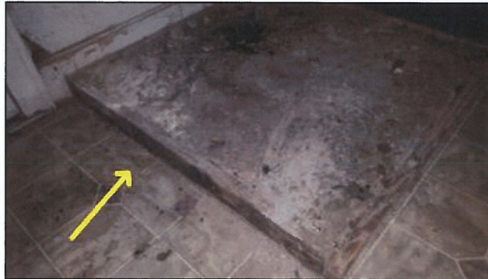
Stone/concrete hearth in dining room
