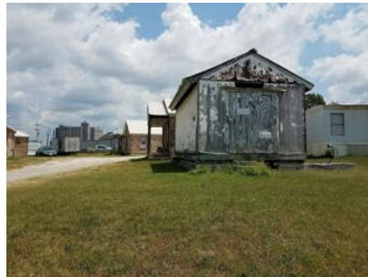
Figure 42 – 2300 block N Delaware Ave, east side
