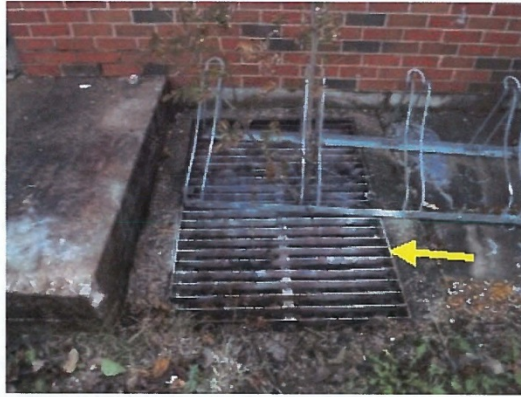
Drainage grate at the east side of the garage addition
