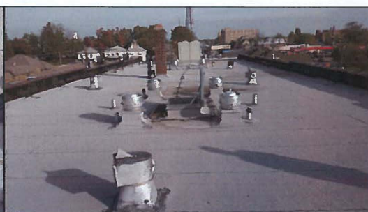
View of main roof looking North
