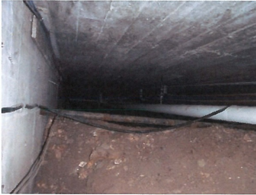
Partial view of south crawl space looking east
