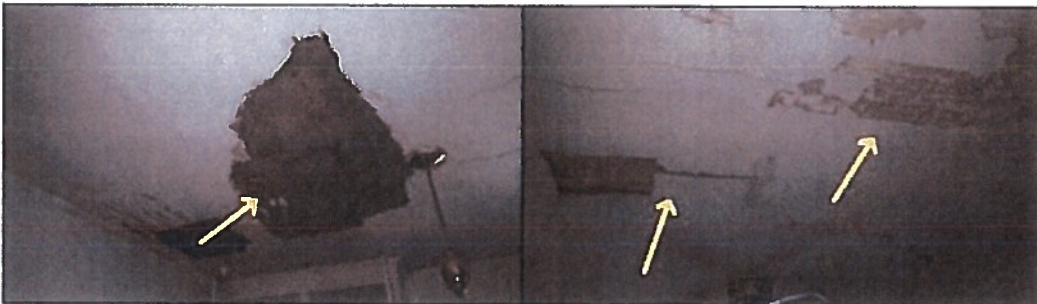
Dining room ceiling
