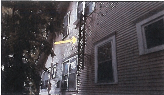
Fire escape ladder noted on East side
