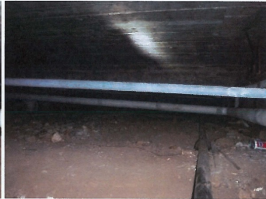
View at middle part of the NW crawl space
