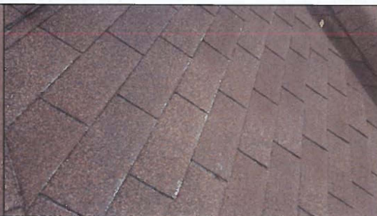
Granular loss/wear
