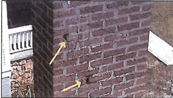
Missing mortar
