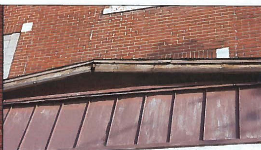
Exposed rafters - Entry
