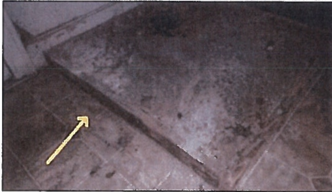
Stone/concrete hearth in dining room
