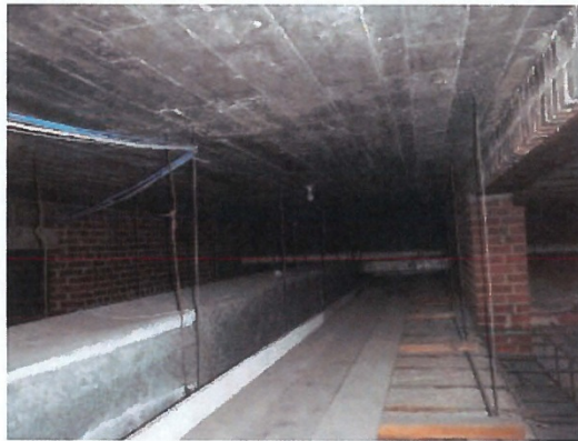
View in middle part of attic space looking west
