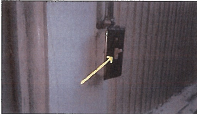
Improper switch
