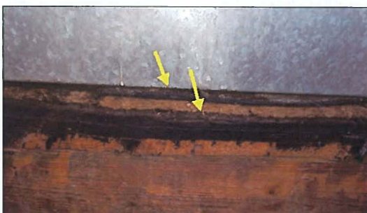
Multiple layers of roofing visible at access
