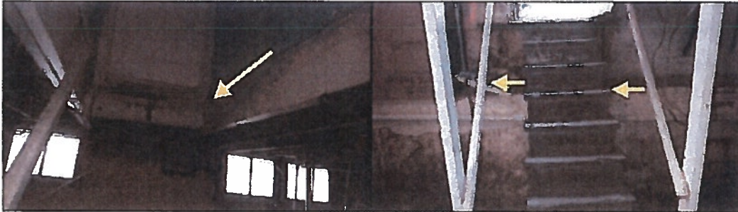
Interior stairway has been removed and door locked with deadbolt
