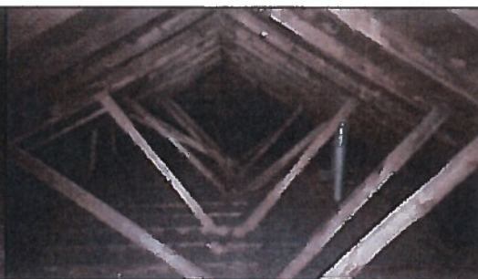
View of attic looking North from above living room.
