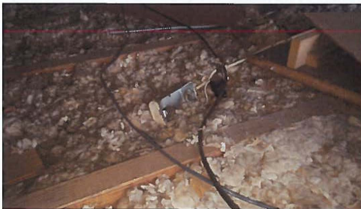
Exposed splices in attic
