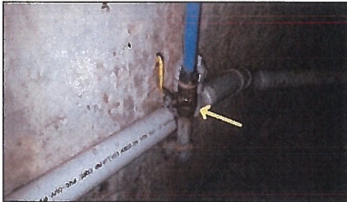
Main water shut off
