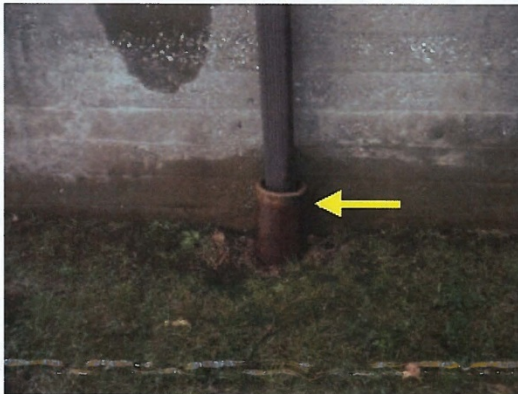
Downspouts at the east corners of the building dispel into sub-surface drains
