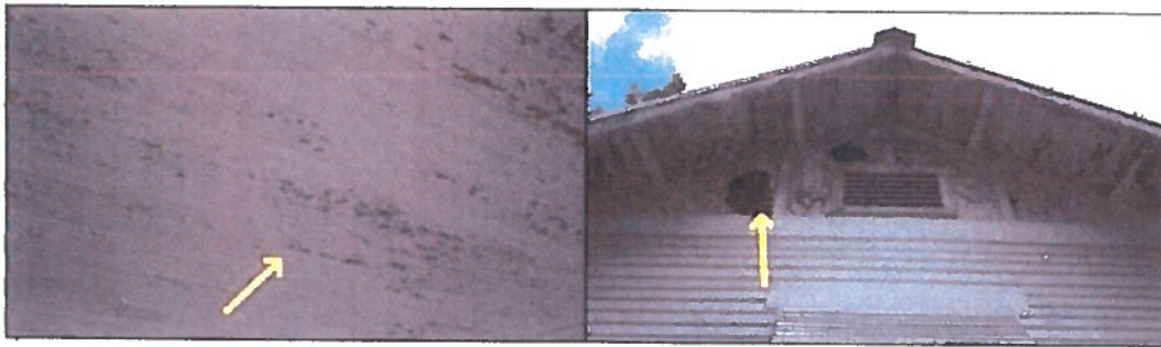
Holes in asphalt paper on West gable
