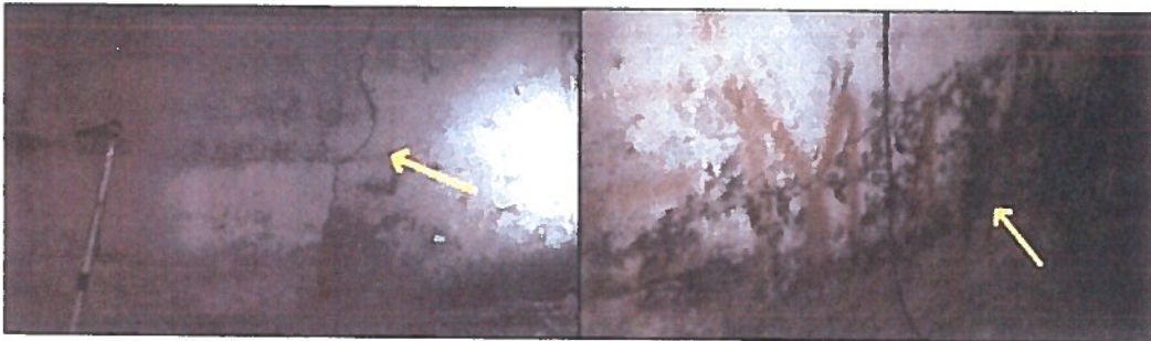
Stains/fungal growth on SE stem wall.
