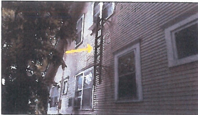
Fire escape ladder noted on East side
