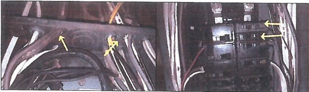
240v breaker has been improperly switched with two 120v breakers in main disconnect section of panel.
