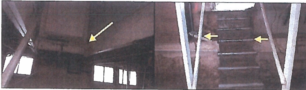
Basement stairway handrail is improper
