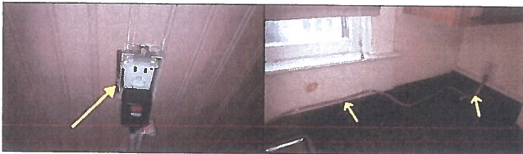
Extension cord permanently installed - Unit 2
