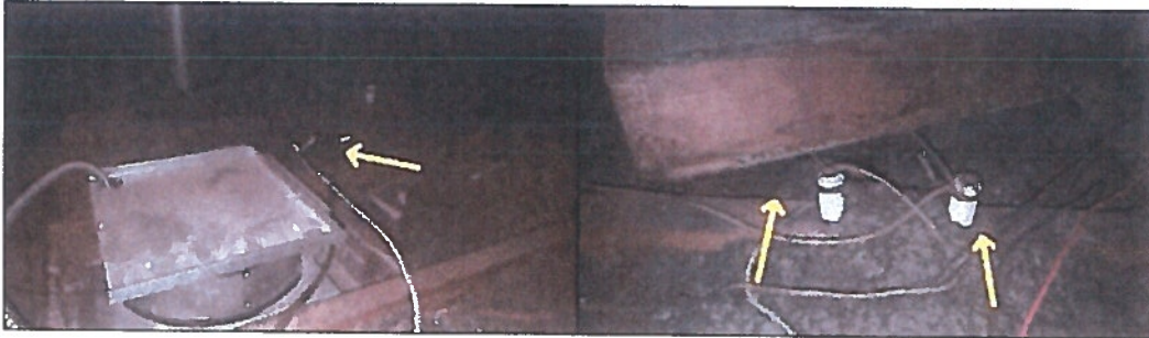
Knob and tube wiring noted
