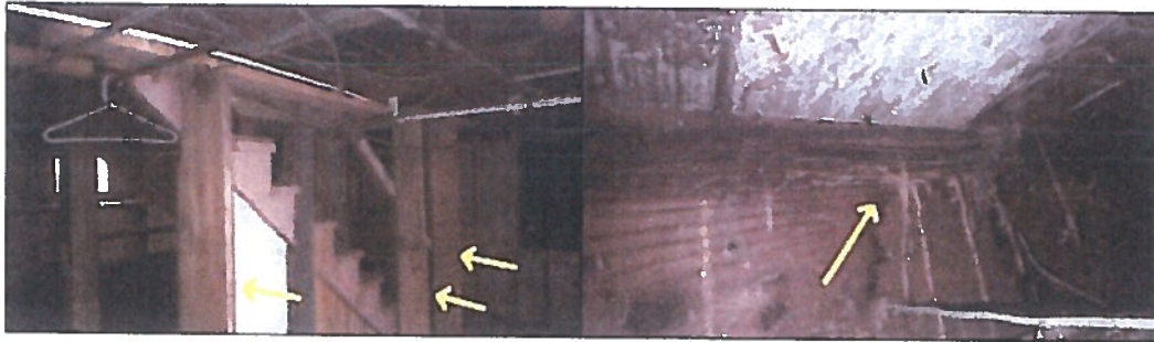
Signs of termite damage near exterior stairway. (Full termite report available if requested.)
