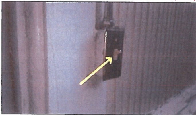
Improper switch
