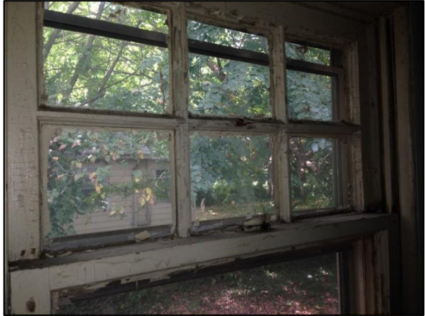
A18.) Chipping interior paint
