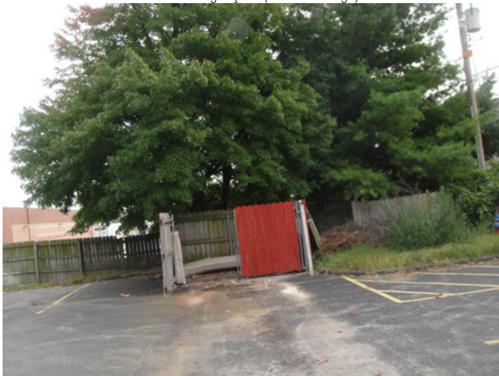
Deteriorating Site Improvements
