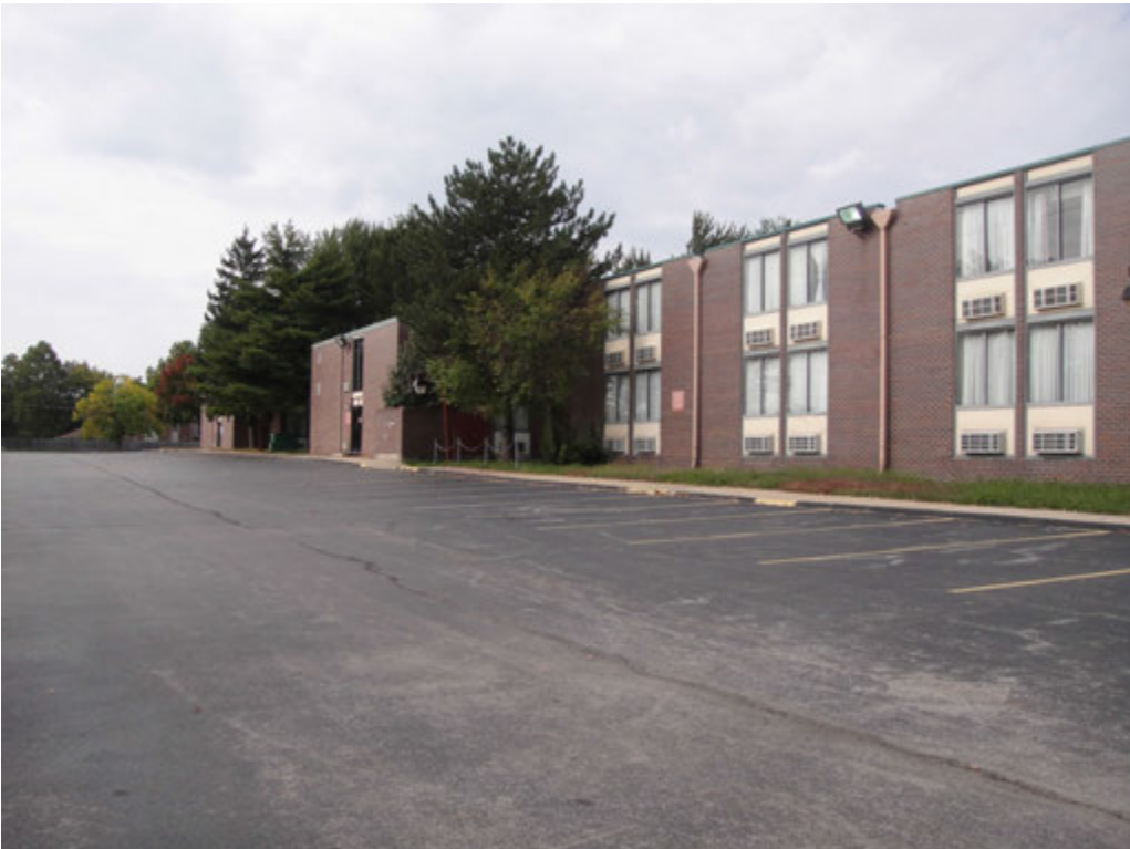
Deteriorating Surface Parking
