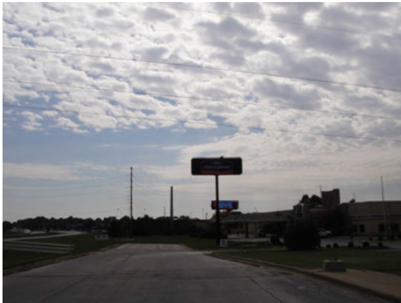
Premature sidewalk termination / No connection to bus stop
