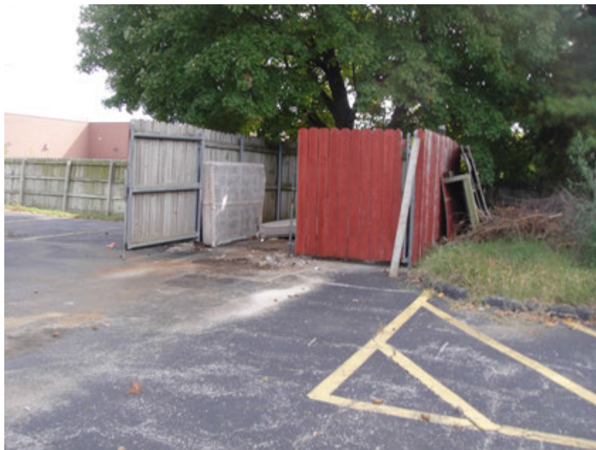
Damaged fencing with missing and/or damaged pickets
