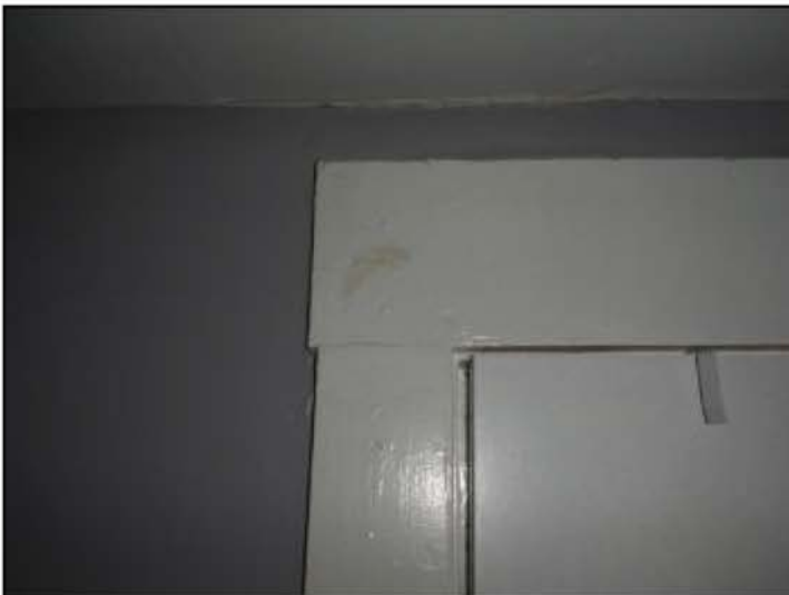
Frames out of square, typical for age
