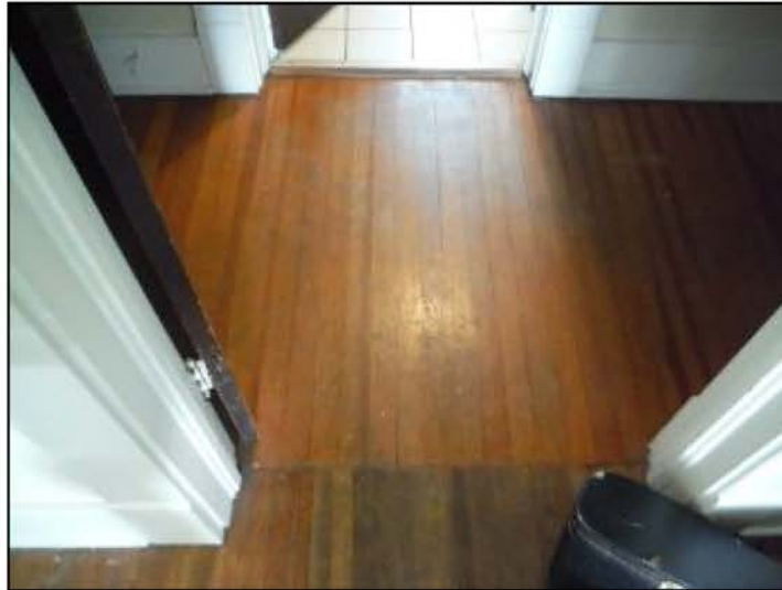
Generally serviceable, normal wear and tear
