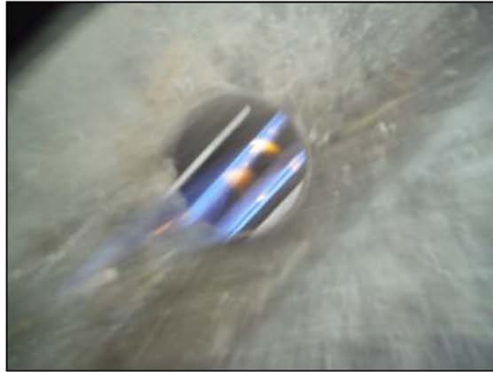
Serviceable flame pattern and color
