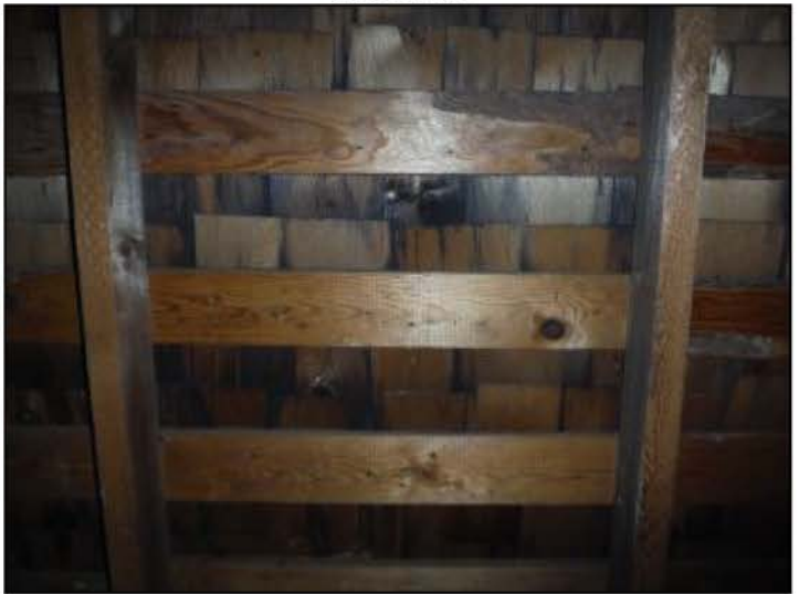
Wood shingles over gapped boards/sheathing, then two or more layers of composition shingles
