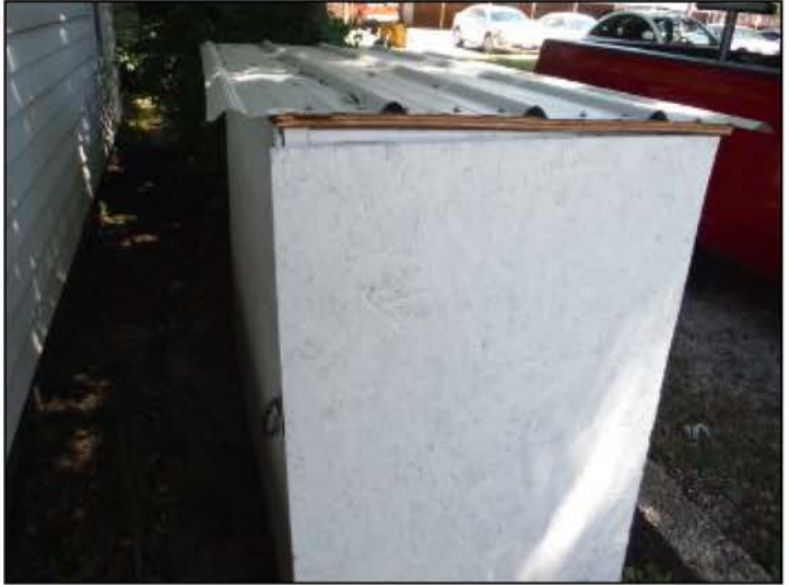
Makeshift storage shed works
