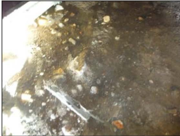
Dry ground, partial plastic film
