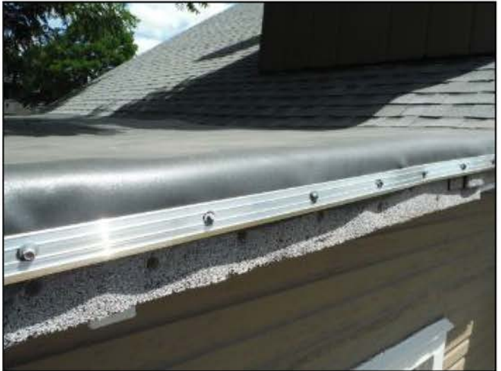
EPDM top layer recover over multiple layers of composition
