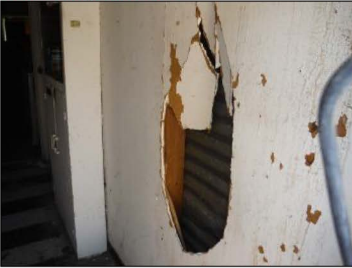
Damaged drywall
