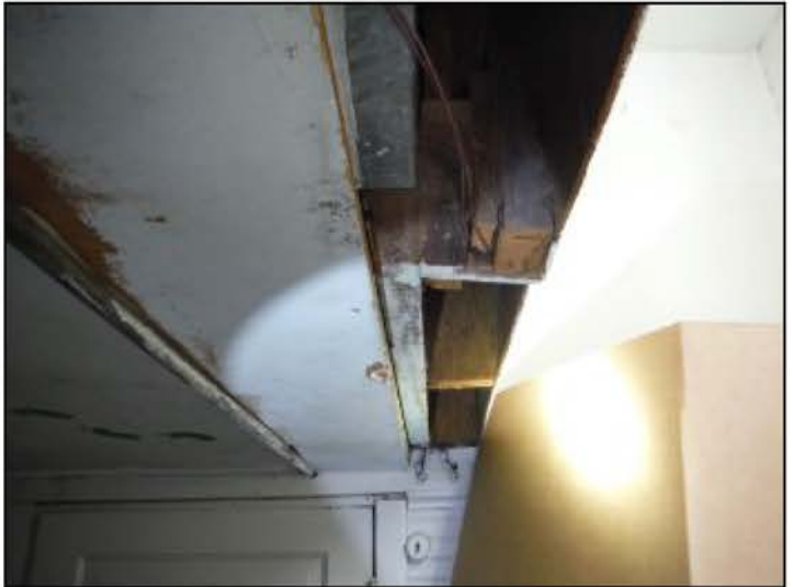
Mostly finished, limited inspection
