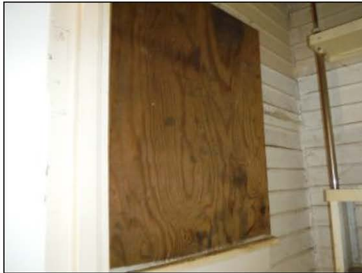
Unvented space, not to current commercial standards
