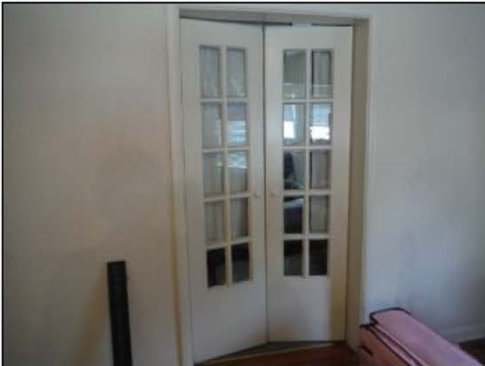
Untempered glass not to current standards at French set
