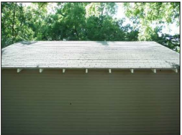
Older three tab composition roofing, limited evaluation
