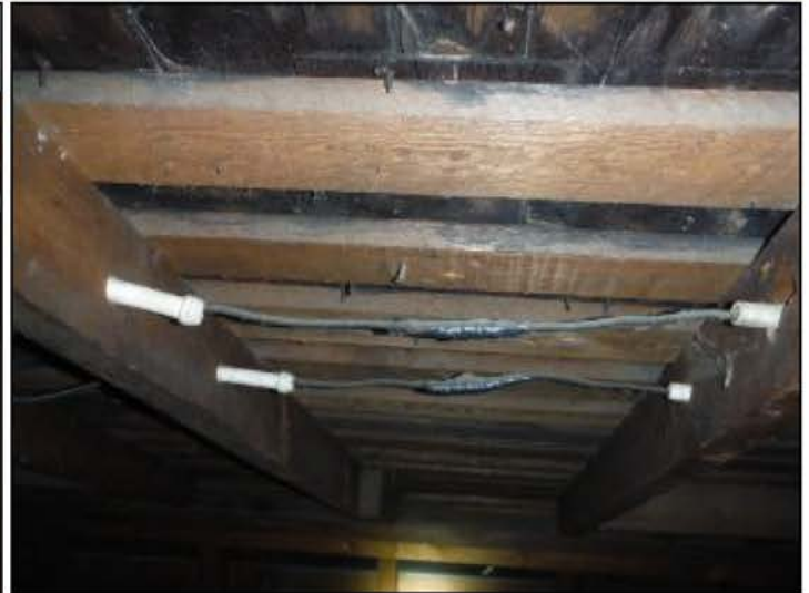
Multiple layers of roofing, first layer is wood (is sheathing/substrate for composition)
