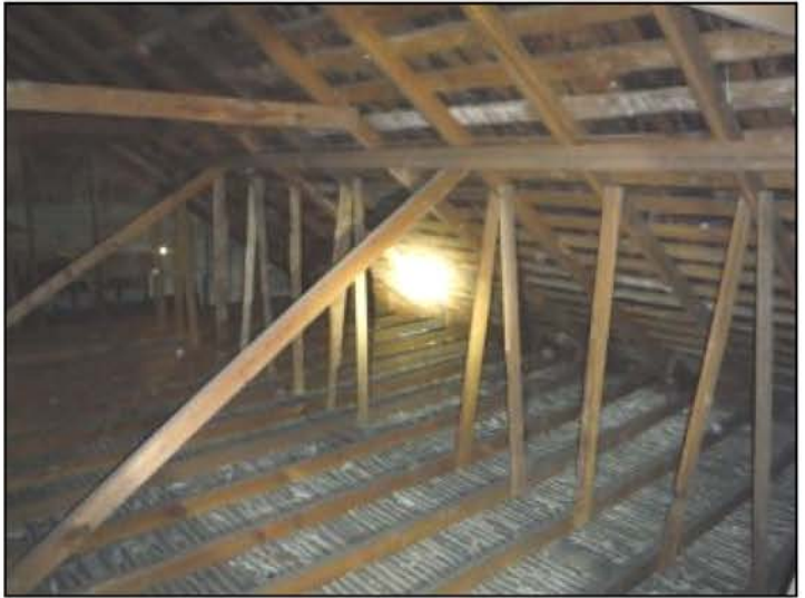
Roof structure appears serviceable, no defects observed
