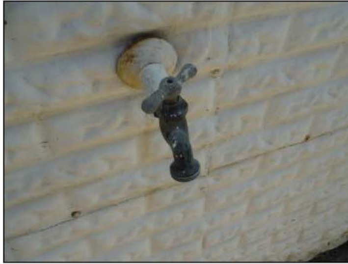
Not frost free type, untested (no water)
