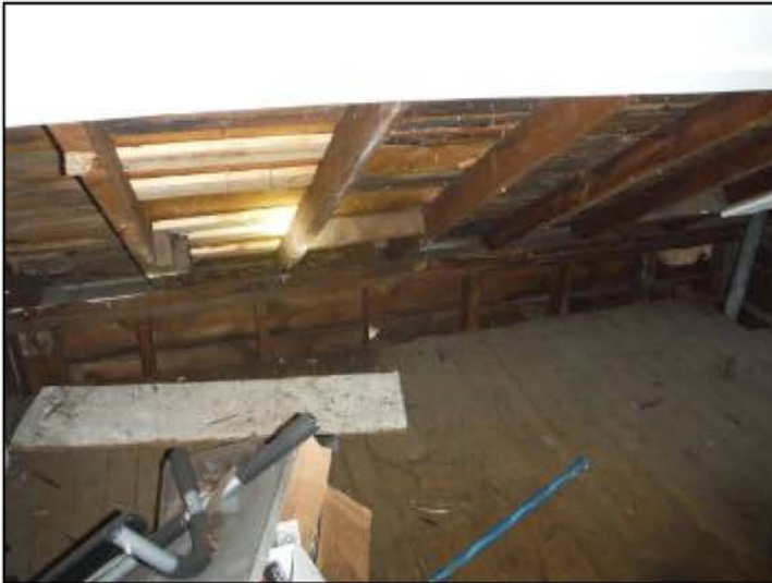
Partial access, this area is floored
