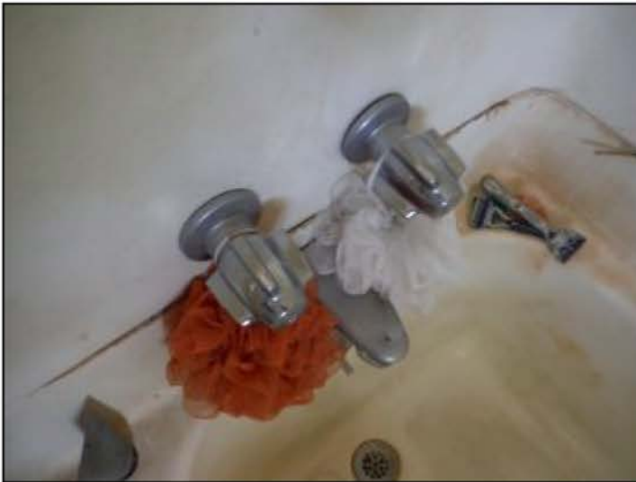
Note valves not balance type
