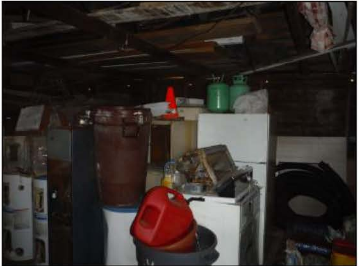
Storage limits inspection, some is hazardous
