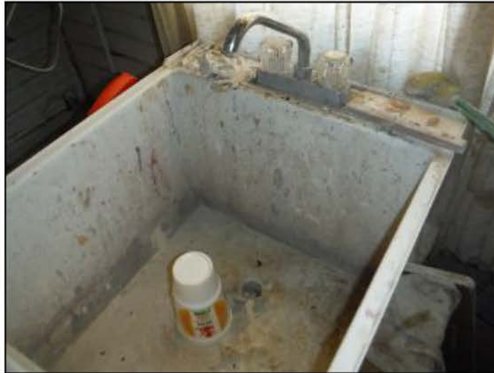
Untested wash tub sink, water off
