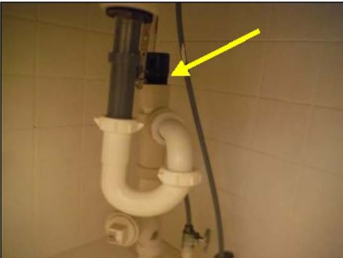
Pro vent below half bath sink, sign of modified system
