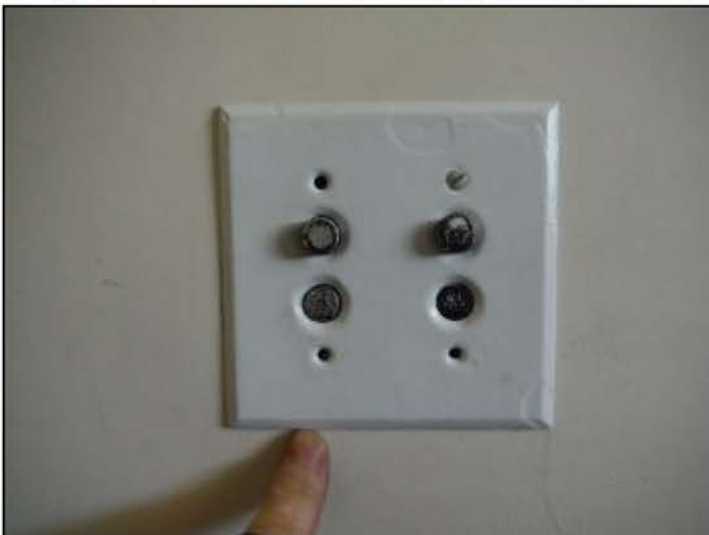
Some push button switches have mercury in them
