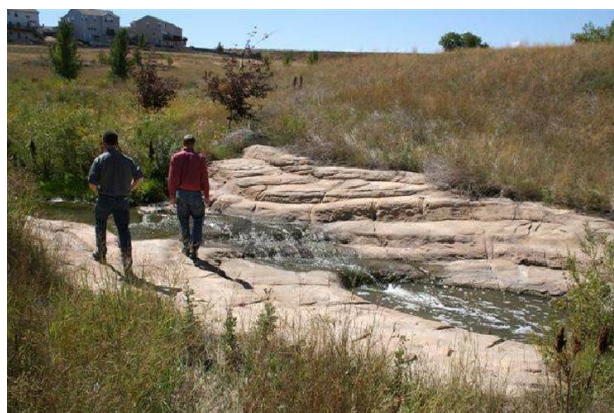
Photo 15. Sculpted sloping grade control structure designed to blend into landscape.
