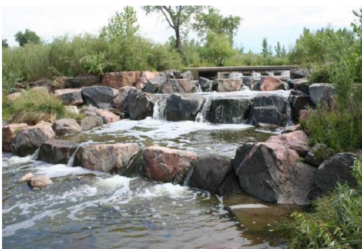
Photo 8. Grouted boulder channel and drop structures.
