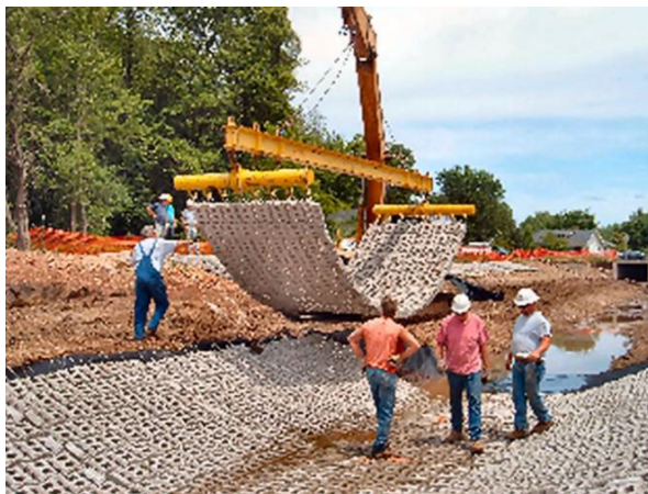
Photo 11. A large, retrofitted urban composite channel using articulated concrete blocks, TRM, sod, and seed/mulch during construction.
