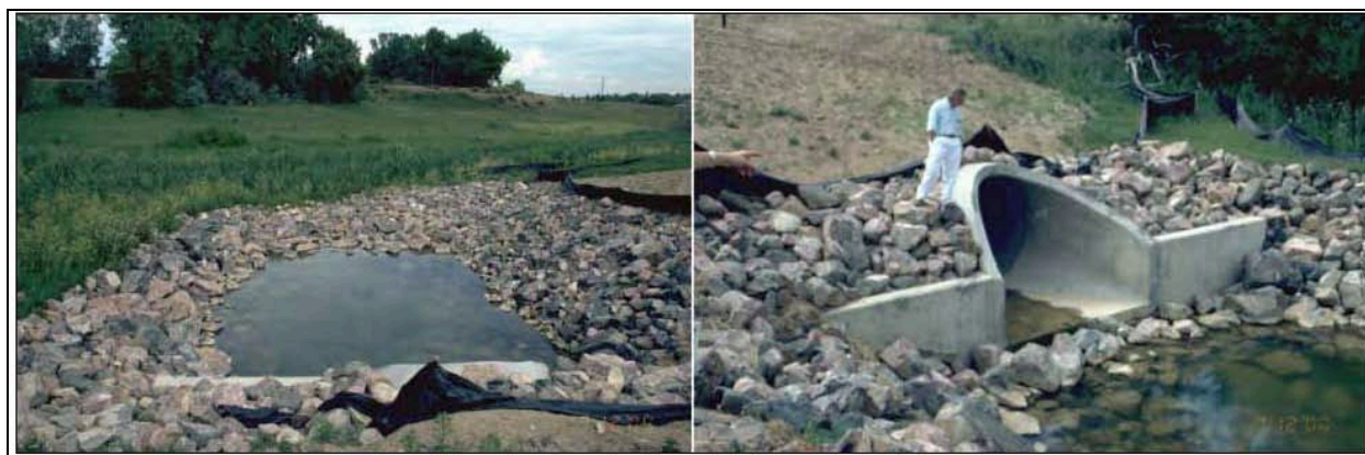
Photograph 5. Upstream and downstream views of a low tailwater basin protecting downstream wetland area. Burying and revegetation of the rock would blend the structure better with the adjacent terrain
