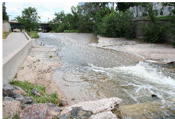
Photo 13. Sloping concrete grade control structure.
