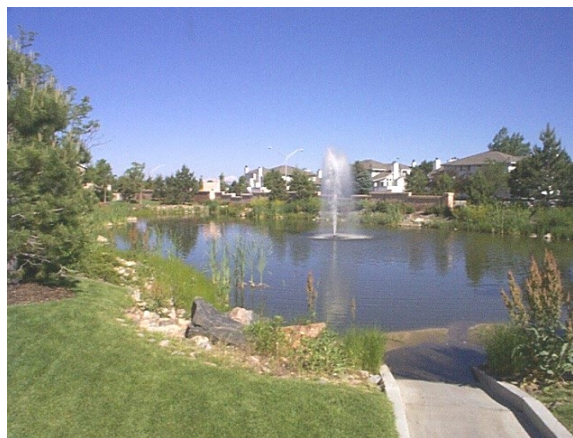
Photo 17. Extended wet detention basin.
