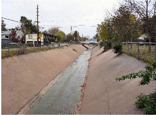
Photo 10. Trapezoidal concrete channel.
