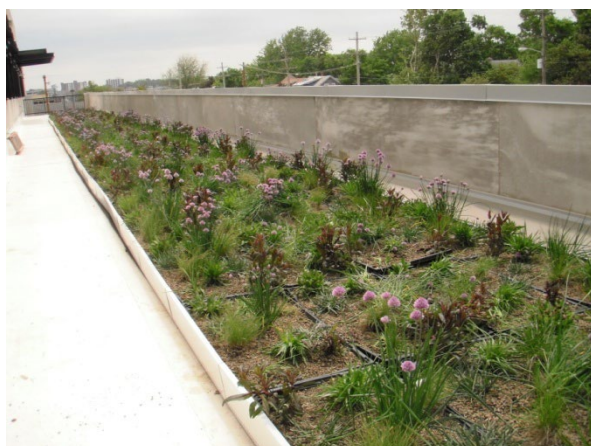
Photo 18. Extensive green roof on employee balcony of Greene County Public Safety Center.
