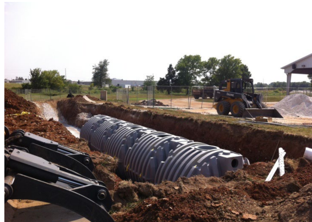
Photo 23. Installation of underground cistern at the Missouri State University Pinegar Arena.
