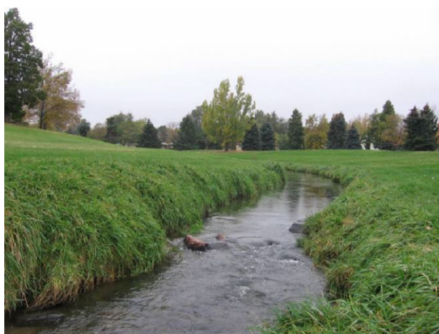
Photo 7. A small channel stabilized with riprap and vegetation.
