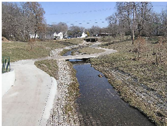
Photo 12. Urban composite channel from Photograph 11, shortly after construction.
