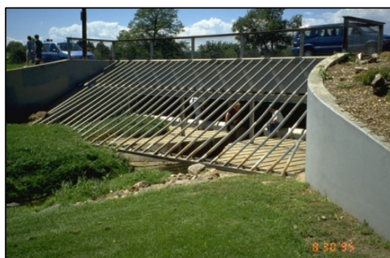
Photograph 1. Public safety considerations for long culverts should be accounted for with designs such as this collapsible trash rack at a park-like setting.
