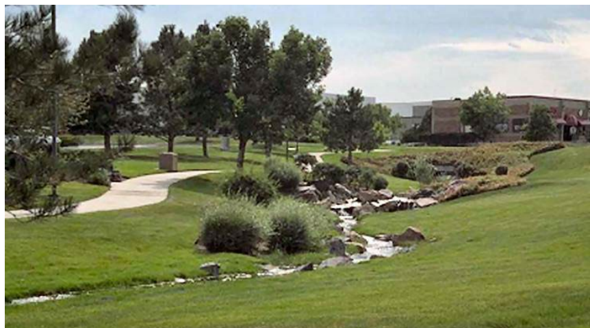
Photo 4. Engineered grass-lined drainageway with rock-lined, low-flow channel, natural components and community recreation uses.
