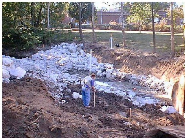
Photo 14. Newbury-style grade control structure under construction.
