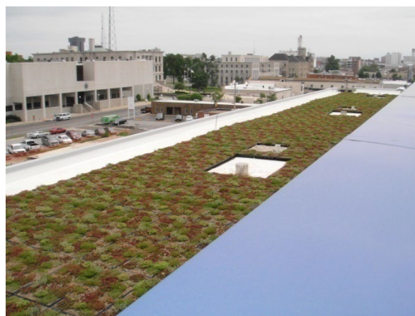
Photo 19. Extensive green roof on Greene County Public Safety Center.
