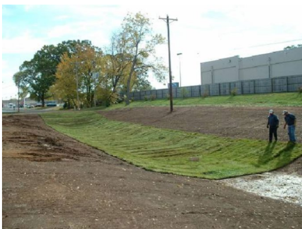
Photo 5. A large drainageway with a reinforced sod channel lining to maintain stability and enhance water quality.
