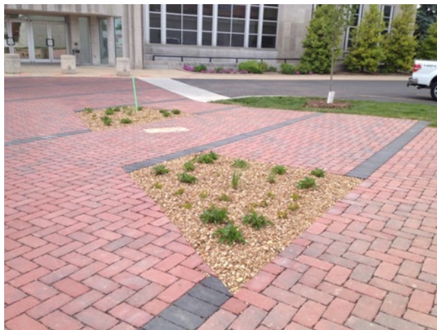
Photo 10. Permeable interlocking concrete pavers at the City Government Plaza.
