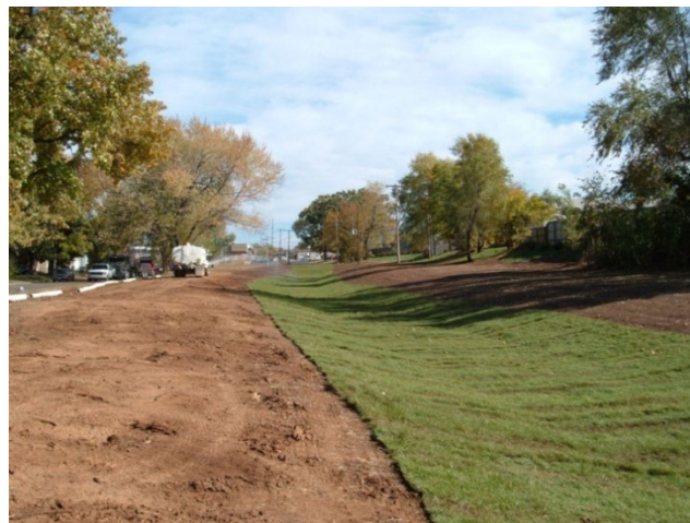
Photo 8. Construction of a grass channel along Erie Street.
