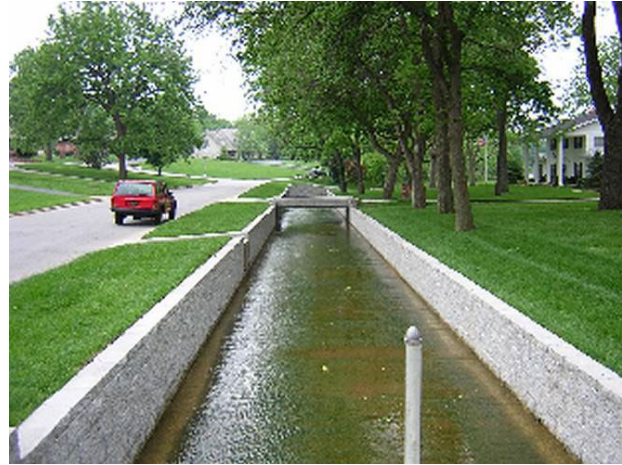
Photo 9. Rectangular channel constructed of concrete and modular blocks.
