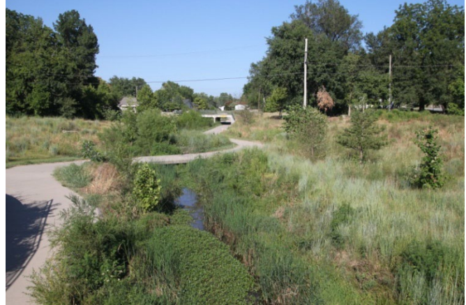
Photo 1. A well planned major drainageway provides biological diversity, recreational opportunities, and aesthetic benefits in addition to flood conveyance.
