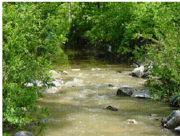
Photo 17. Newbury-style grade control structure following construction.
