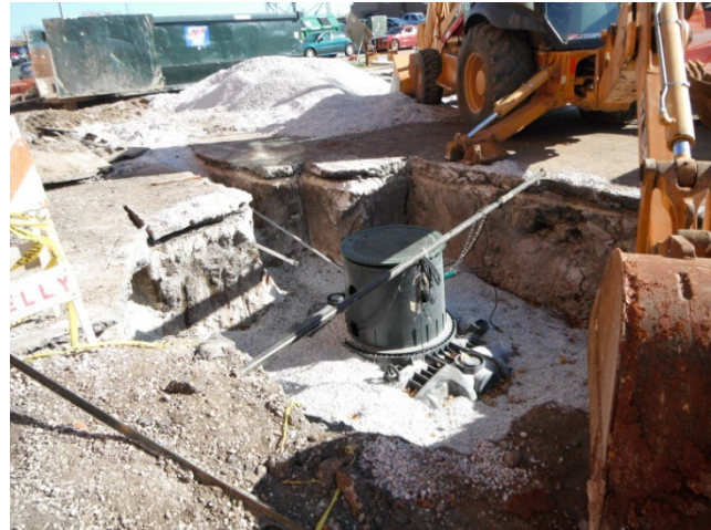
Photo 22. Installation of underground cistern at the City Environmental Resource Center.
