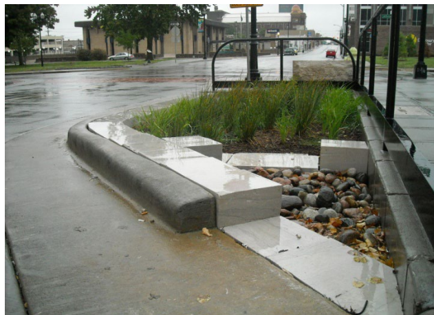
Photo 12. Rain garden on Park Central East and Jefferson.
