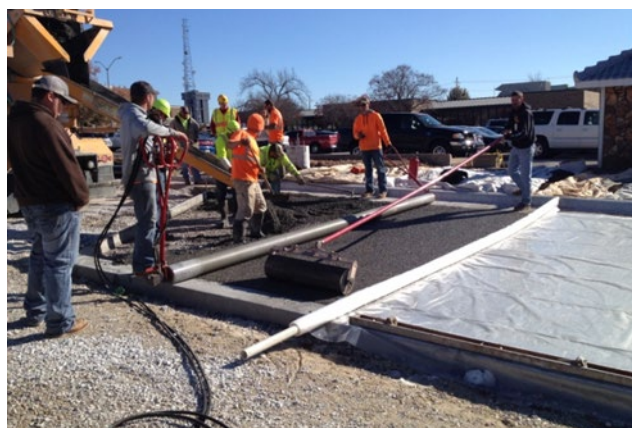
Photo 11. Installation of pervious concrete at the City Government Plaza.
