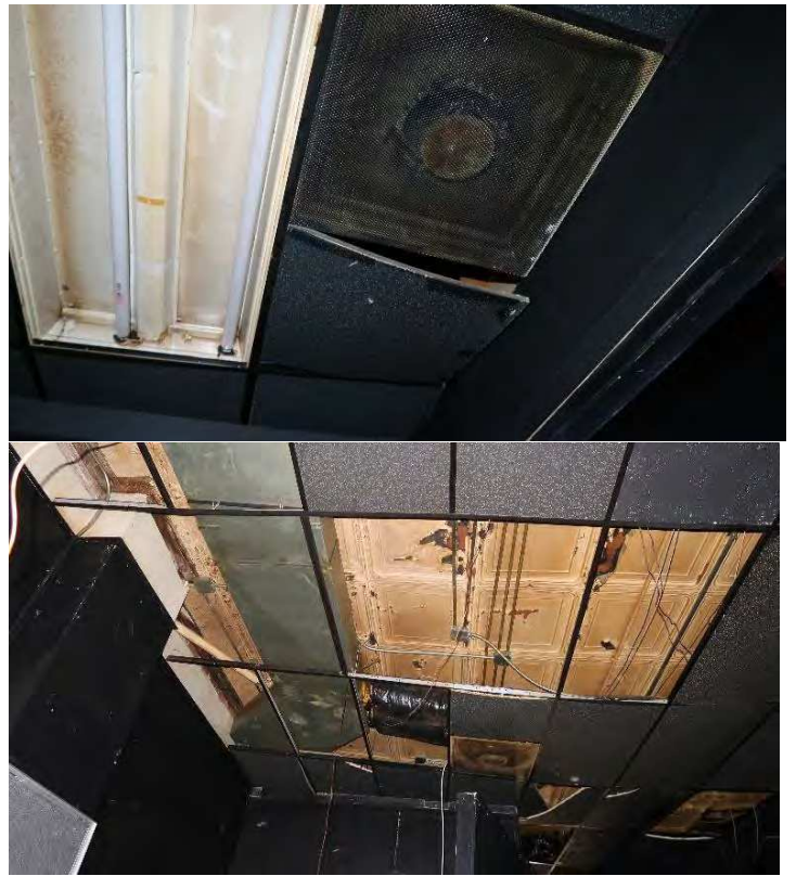
Inside Nightclub / Saw & Tool Building: Many ceiling tiles missing throughout the building. Evidence of water damage in many places on the ceiling above the tiles. Many electrical wires hanging from the ceiling with electrical conduit exposed.
