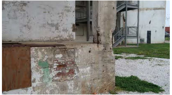
Front Elevation of JVIC Building: Concrete columns are deteriorated to the point where rebar reinforcement is exposed to the elements and shows signs of significant rust.
