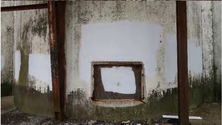
North Elevation of Area 3 Grain Tower (below steel platform): Pillars supporting the steel platform are significantly rusted. Concrete footings into which the pillars are secured are deteriorated with evidence of spalling. Exterior of concrete structure is dilapidated with large holes in exterior walls which have been covered by temporary wood and metal patches. A large rusted steel box, lumber, old sandbags and other trash are scattered about the front of the premises.
