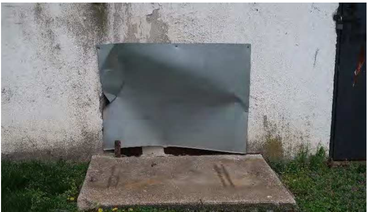
South Elevation of Area 2 Grain Tower: Large holes and smaller holes in exterior wall. Temporary metal patch over ground level opening is dented inward creating easy entry points for rodents, snakes and other pests. Deteriorating concrete pad on ground with rusty bolts protruding above the concrete surface creates a trip and fall hazard. Rusted metal pipes and other rusted metal components protruding from exterior walls.
