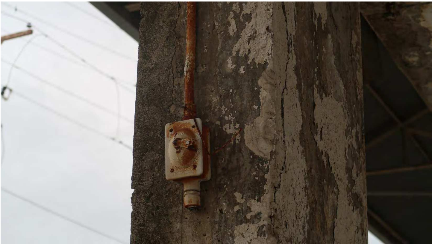
Electrical conduits and components simply cut off at reachable level.
