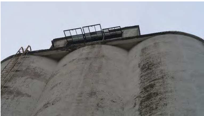
North Elevation of Area 2 Grain Tower: Ladder extending to the top of the grain tower shows significant rust. Remains of electrical service simply cut off.
