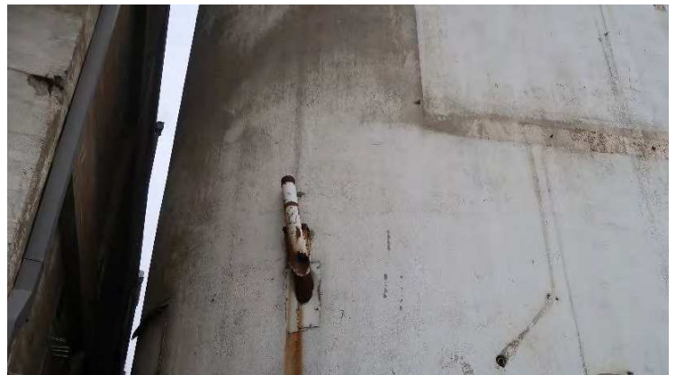
South Elevation of Area 2 Grain Tower: Large holes and smaller holes in exterior wall. Temporary metal patch over ground level opening is dented inward creating easy entry points for rodents, snakes and other pests. Deteriorating concrete pad on ground with rusty bolts protruding above the concrete surface creates a trip and fall hazard. Rusted metal pipes and other rusted metal components protruding from exterior walls.
