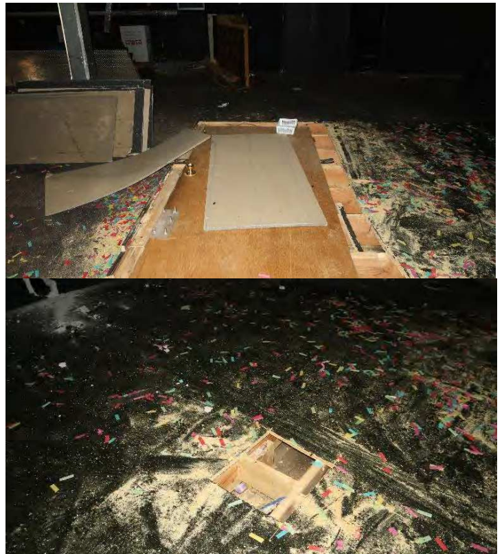
Inside Nightclub / Saw & Tool Building: Substantial air and light infiltration around temporary patches over entryways reflects building is not well secured from the elements. Holes cut into the floor of the building create open hazards.
