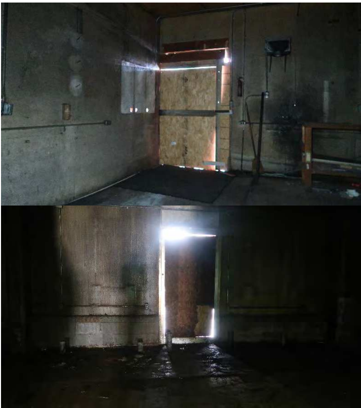
Inside Nightclub / Saw & Tool Building: Substantial air and light infiltration around temporary patches over entryways reflects building is not well secured from the elements. Holes cut into the floor of the building create open hazards.
