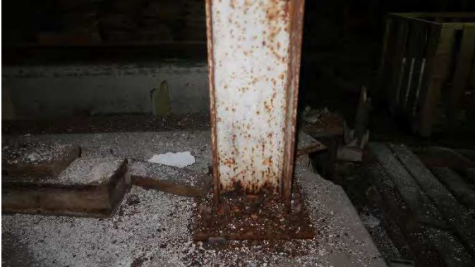
Inside JVIC Building: Concrete and steel structural components show significant decay, including spalling of concrete surfaces and severe rust on steel components.
