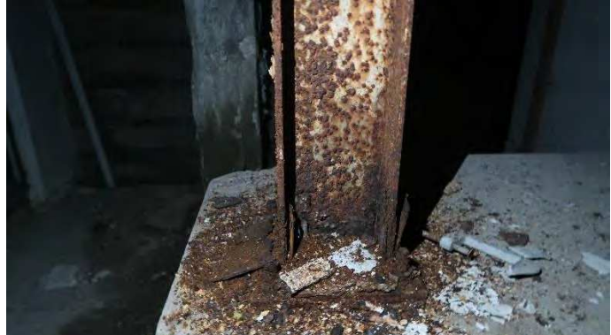
Inside JVIC Building: Concrete and steel structural components show significant decay, including spalling of concrete surfaces and severe rust on steel components.
