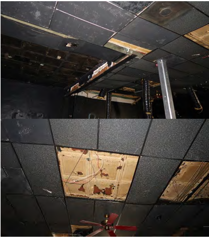
Inside Nightclub / Saw & Tool Building: Many ceiling tiles missing throughout the building. Evidence of water damage in many places on the ceiling above the tiles. Many electrical wires hanging from the ceiling with electrical conduit exposed.
