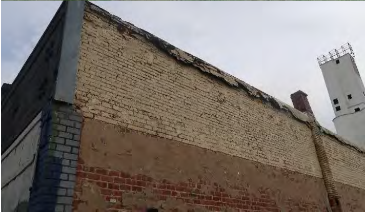
Side (South) Elevation of Nightclub / Saw & Tool Building: Brick façade and roof line are significantly deteriorated. Portion of brick façade at southeast corner of building appears to be missing. Holes exist in exterior wall and in boards placed over exterior openings.
