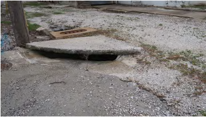
Surface Area Surrounding Area 3 Grain Tower: Deterioration of pavement, damage to pavement and drainage areas from settling of surrounding ground and deterioration of concrete surfaces, combined with large loose rocks, present trip and fall hazards to passersby.
