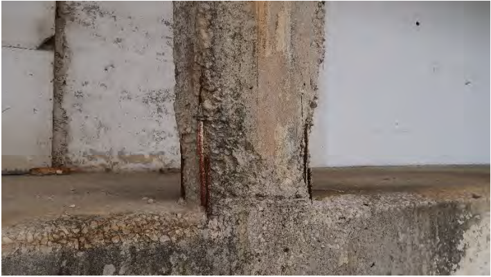
Front Elevation of JVIC Building: Concrete columns are deteriorated to the point where rebar reinforcement is exposed to the elements and shows signs of significant rust.
