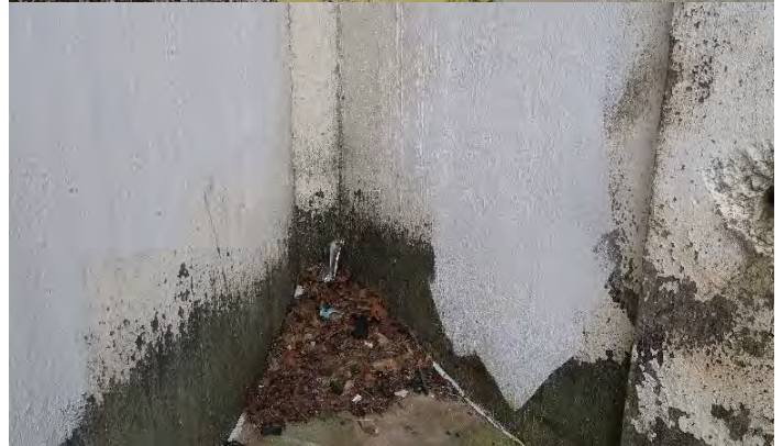
North Elevation of Area 3 Grain Tower (below steel platform): Pillars supporting the steel platform are significantly rusted. Concrete footings into which the pillars are secured are deteriorated with evidence of spalling. Exterior of concrete structure is dilapidated with large holes in exterior walls which have been covered by temporary wood and metal patches. A large rusted steel box, lumber, old sandbags and other trash are scattered about the front of the premises.
