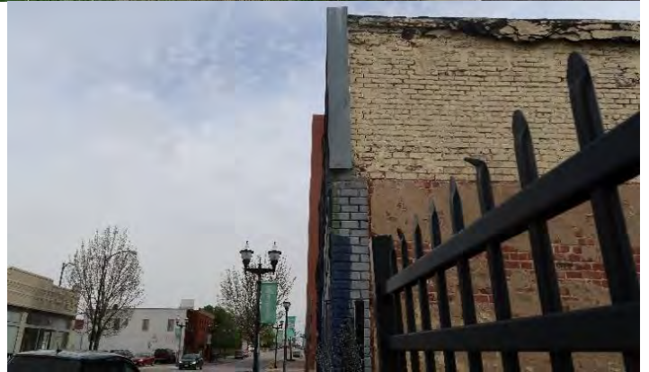
Side (South) Elevation of Nightclub / Saw & Tool Building: Brick façade and roof line are significantly deteriorated. Portion of brick façade at southeast corner of building appears to be missing. Holes exist in exterior wall and in boards placed over exterior openings.
