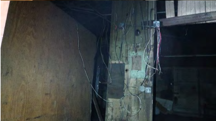
Inside Nightclub / Saw & Tool Building: Exposed electrical wiring is pervasive throughout the interior of the building, including wiring hanging from light fixtures, junction boxes, conduits and breaker boxes. Electrical breaker boxes are open and exposed.
