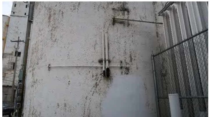
North Elevation of Area 2 Grain Tower: Ladder extending to the top of the grain tower shows significant rust. Remains of electrical service simply cut off.
