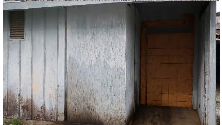
Rear Elevation of Nightclub / Saw & Tool Building: Wood siding is dilapidated with evidence of wood rot. Portions of siding are pulling away from exterior of building. Holes in exterior wall; makeshift patches over doorway and window. Debris scattered around the rear of the building. Pavement is a mix of gravel and weeds on north and east sides of building.
