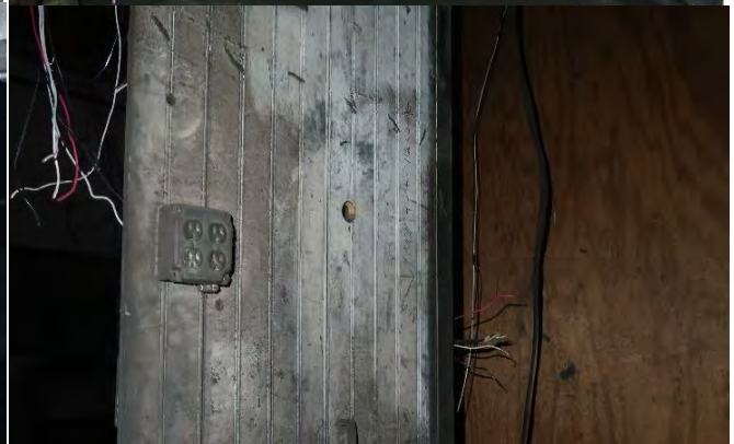
Inside Nightclub / Saw & Tool Building: Exposed electrical wiring is pervasive throughout the interior of the building, including wiring hanging from light fixtures, junction boxes, conduits and breaker boxes. Electrical breaker boxes are open and exposed.
