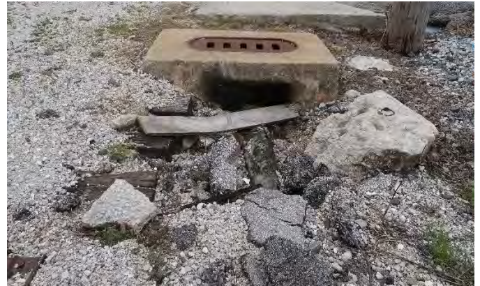
Surface Area Surrounding Area 3 Grain Tower: Deterioration of pavement, damage to pavement and drainage areas from settling of surrounding ground and deterioration of concrete surfaces, combined with large loose rocks, present trip and fall hazards to passersby.
