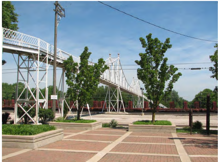
Jefferson Avenue Footbridge, east profile, facing northwest
