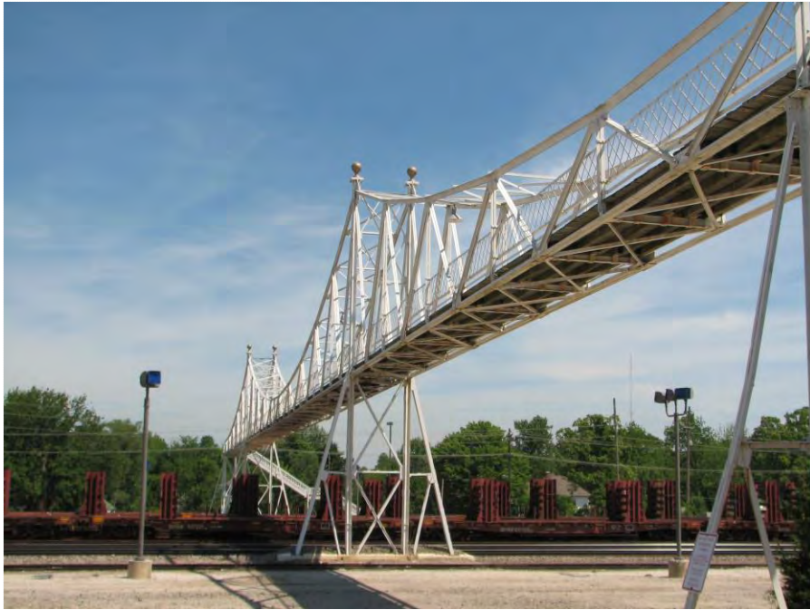
Jefferson Avenue Footbridge, west profile, facing northeast
