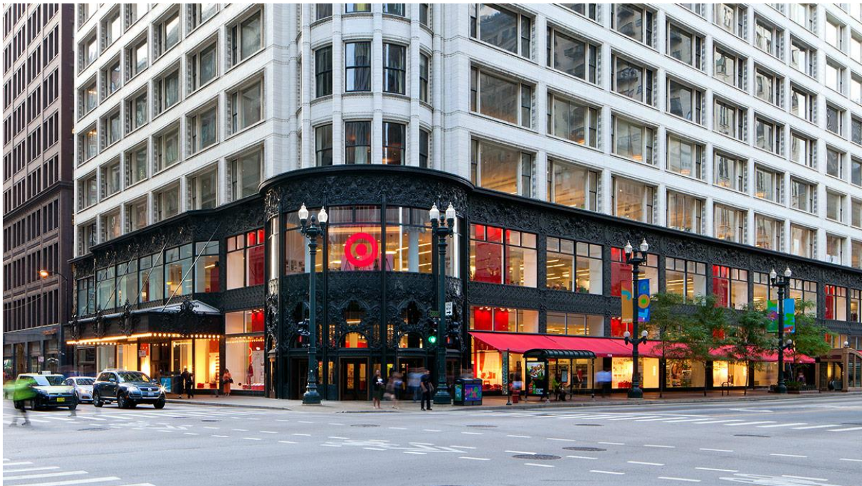
Figure 23 - Carson, Pirie, Scott and Company Building – State and Madison Target Store Photo Courtesy of Walsh Construction
