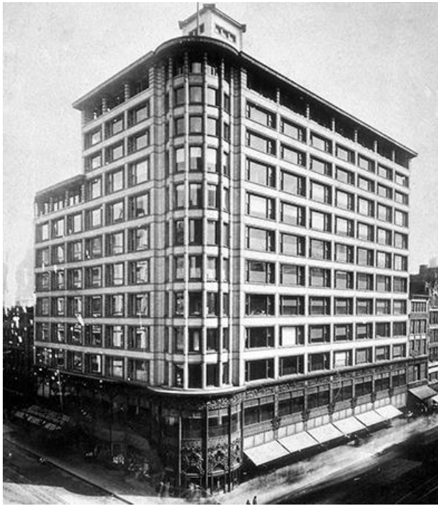
Figure 21 – Carson, Pirie, Scott and Company Building by Louis Sullivan 1898-1899 - Courtesy of City of Chicago Landmarks
