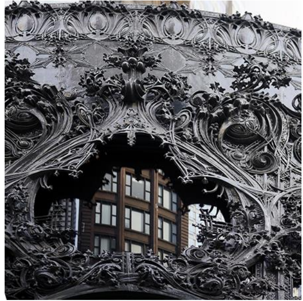
Figure 22 - Carson, Pirie, Scott and Company Building cast iron detailing. Photo courtesy of Dauvit Alexander.
