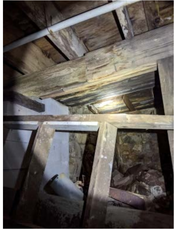
Exterior Access Pit #2 in Basement
