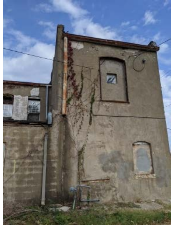
South Exterior Wall (East Side)
