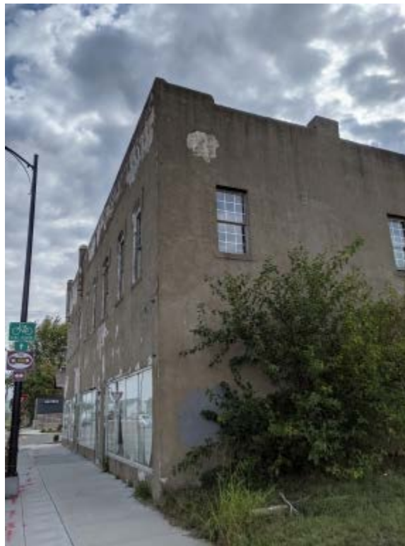
North-West Exterior Corner
