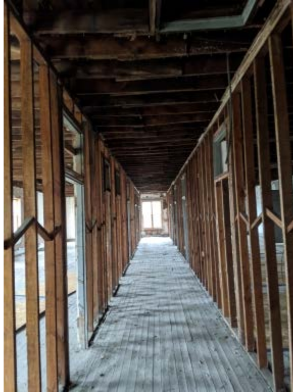
Load-Bearing “Hallway” Walls on Second Floor of West Suite
