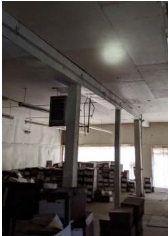
Beam-Column Line on First Floor of West Suite
