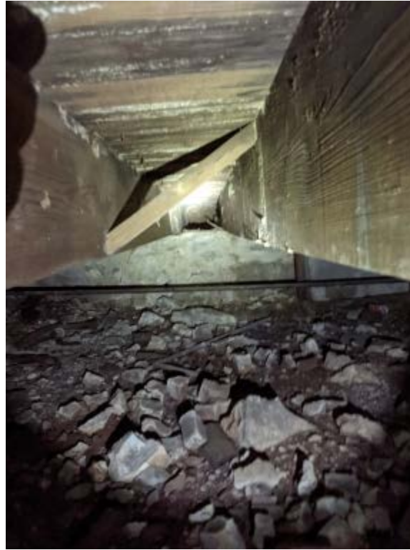
Crawlspace at West Suite
