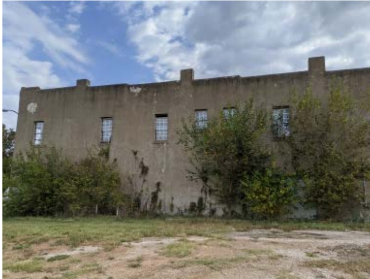
West Exterior Wall
