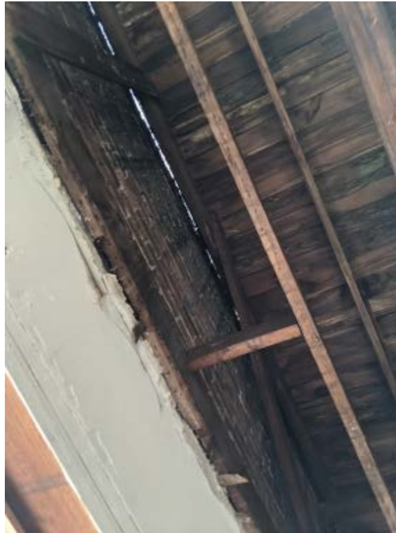
Horizontal Gap at North Wall and Roof of West Suite
