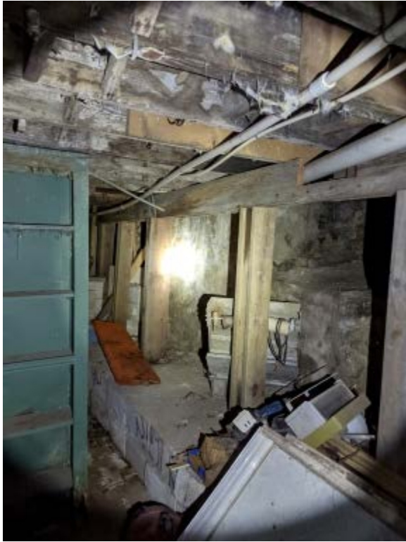
Additional First-Floor Supports in Basement
