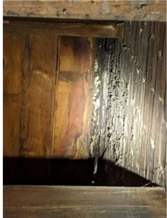
Exposed Roof Membrane at West Suite
