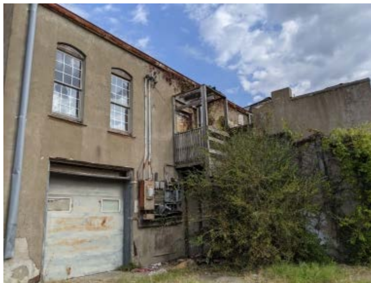
South Exterior Wall (West Side)
