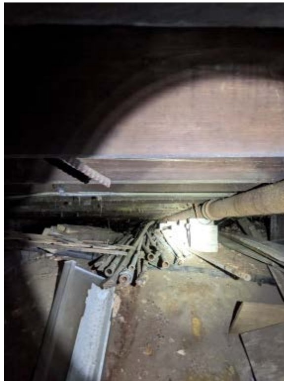
Additional First-Floor Supports in Basement (Cast Iron Pipe Girder)
