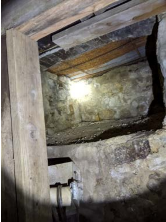
Exterior Access Pit #1 in Basement
