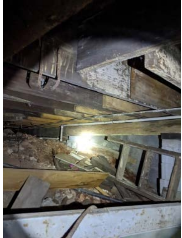
Additional First-Floor Supports in Basement
