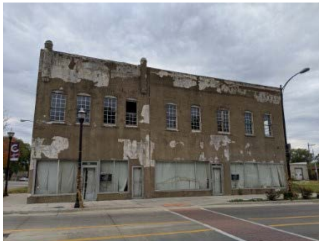
Front of Building
