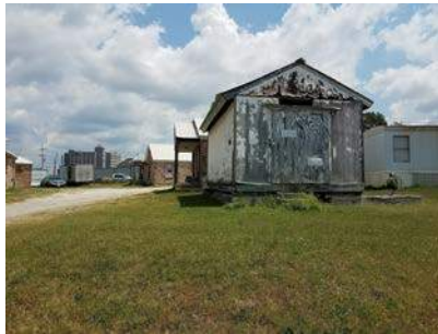
Figure 42 – 2300 block N Delaware Ave, east side
