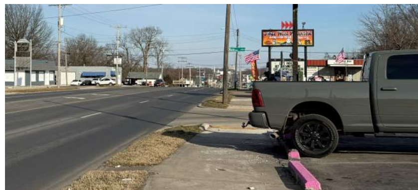
Parking Stops, Site Constraints, Non ADA Compliant.
