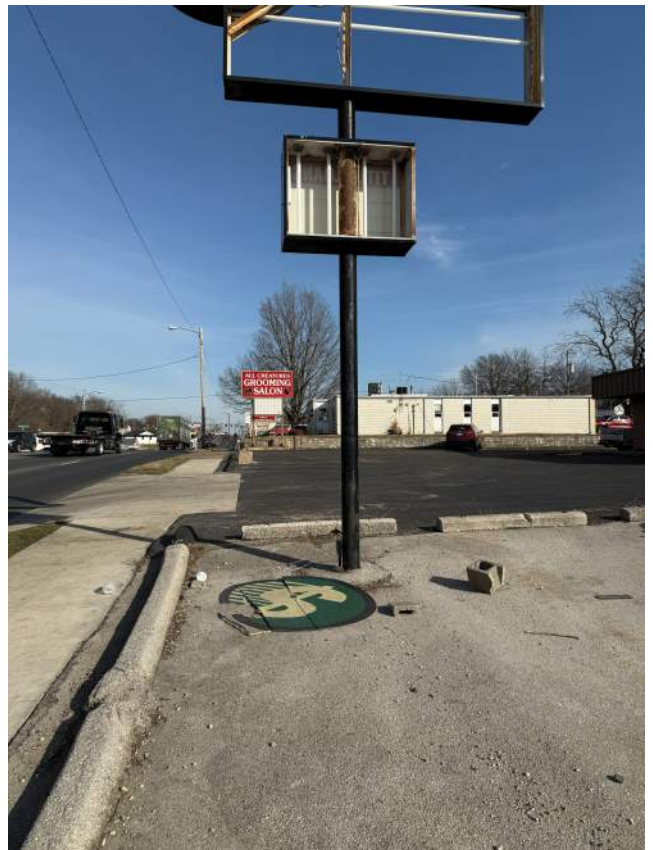
Located at 400 W Kearney, Signage is exposed and deteriorated. Lack of Sidewalk has gravel and uneven surfaces. Non ADA compliant.
