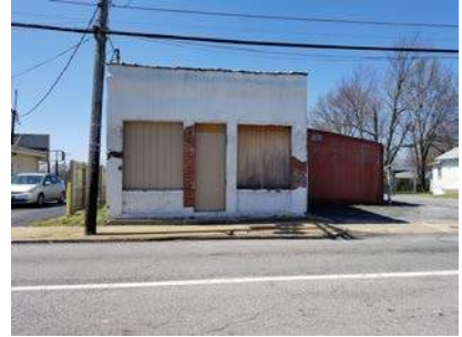
Figure 40 – 2400 block N Grant Ave, west side
