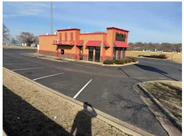
Located at 1421 W Kearney Building vacant.
